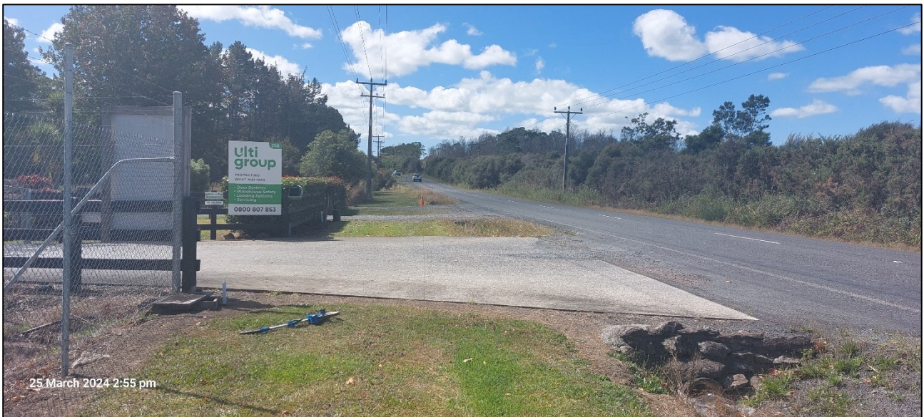
Figure 6 Existing vehicle crossing
