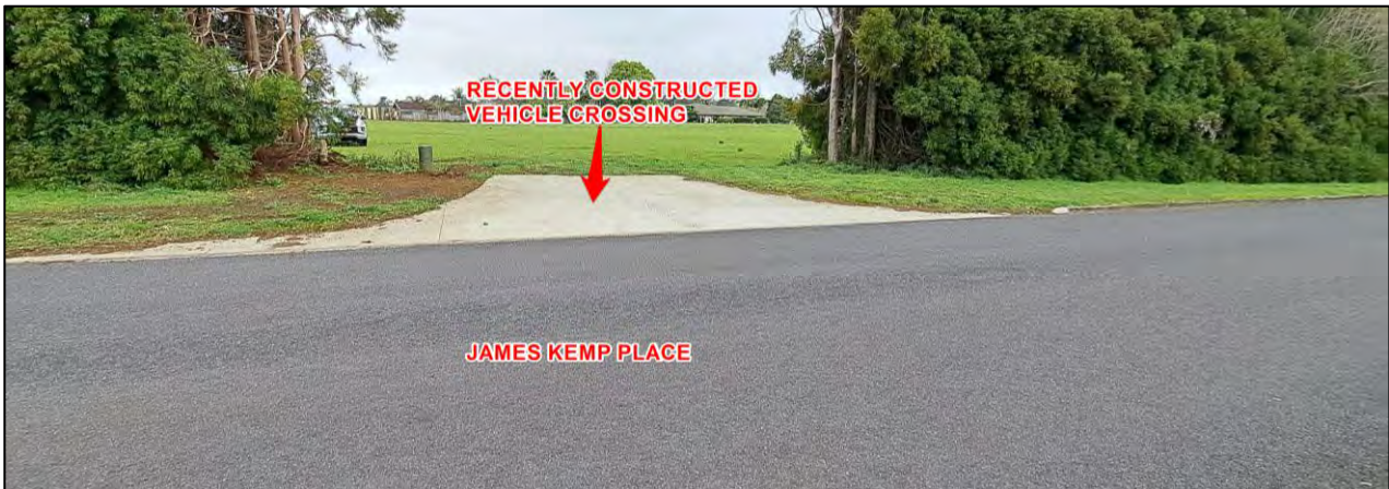
Figure 14: Site Photo Showing Recently Constructed Vehicle Crossing off James Kemp Place.
