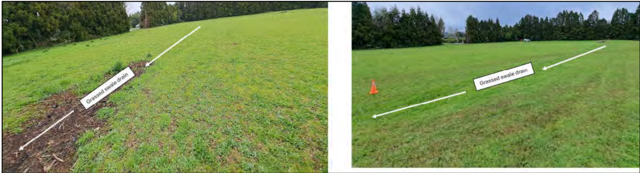
Figure 5: Grassed swale drains traversing through the property.
