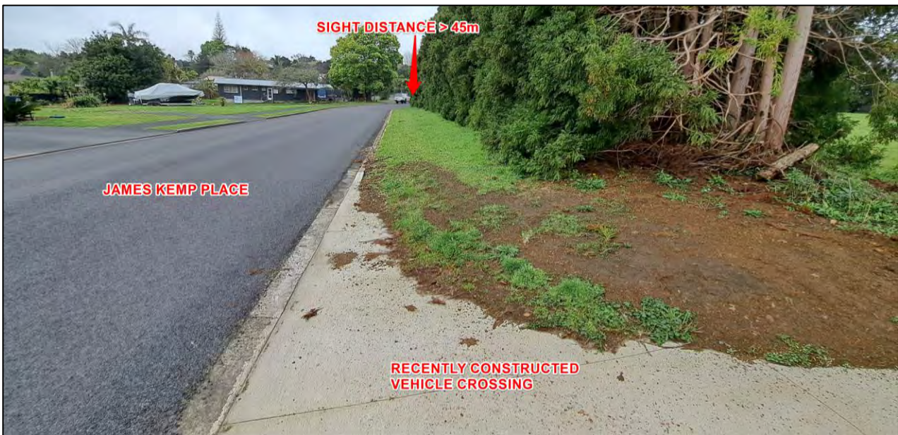
Figure 16: Recently Constructed Access Point on James Kemp Place Facing Northwest, >45m Sight Distance Available.
