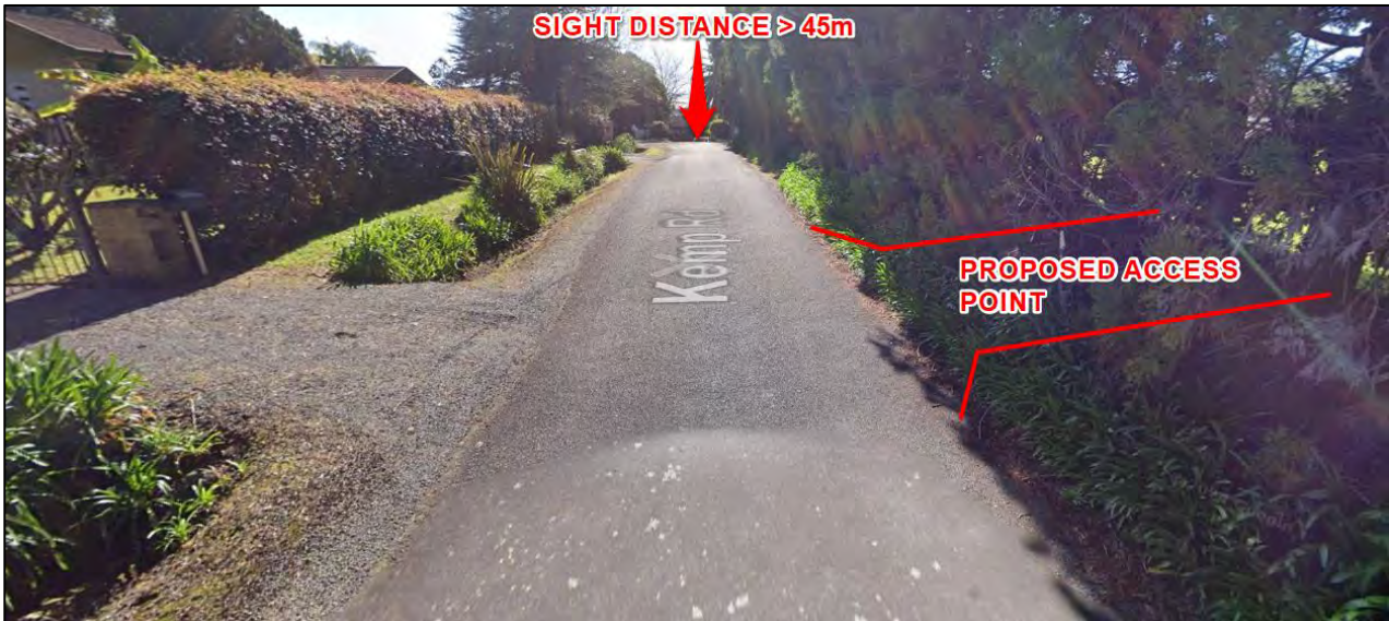
Figure 12: Proposed Access Point on Kemp Road Facing Northeast, >45m Sight Distance Available.
