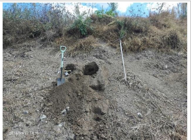
Photograph 9. HA05, stockpile in the proposed location for the boron plant.
