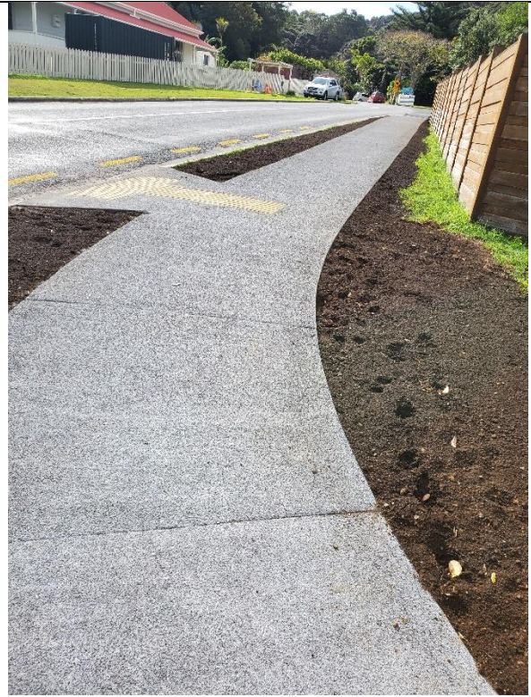
7-23-187 Queen Street New Footpath – Complete
