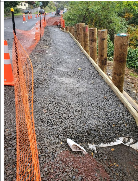
7-23-188 Parnell Street, Rawene – First retaining wall installation.
