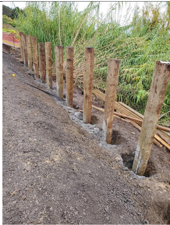
7-23-188 Parnell Street, Rawene – Second retaining wall started
