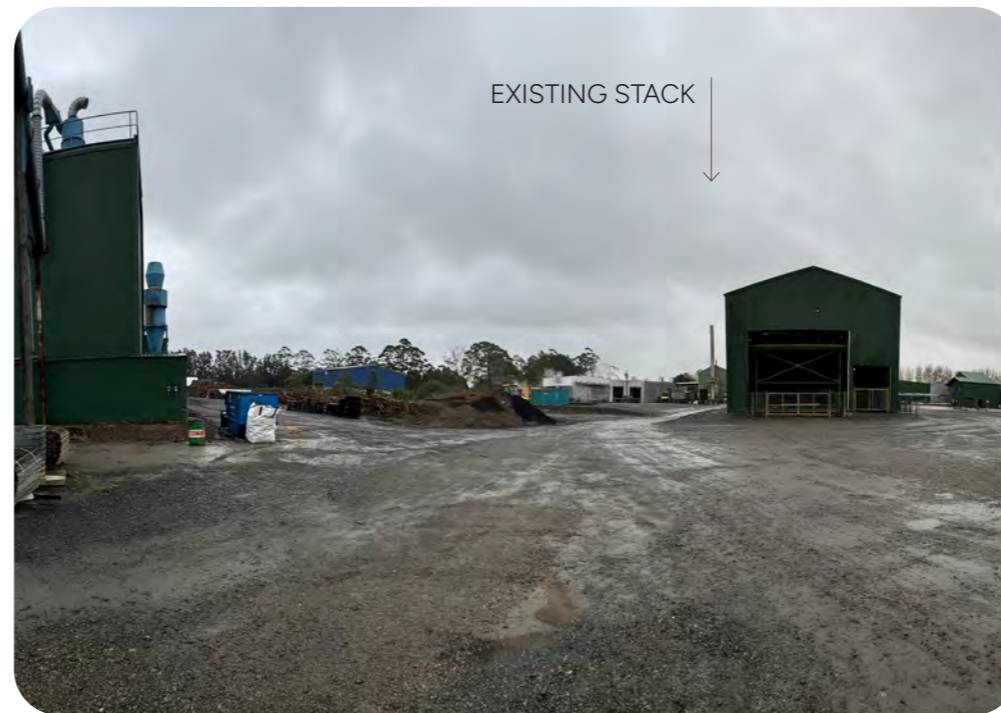
EXISTING STACK PHOTO
