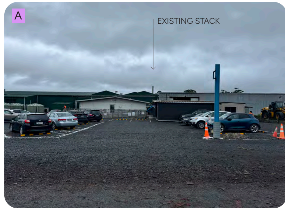
STAFF CAR PARK NORTHERN BOUNDARY Existing stack beyond office, dry mill, and bin sorter
