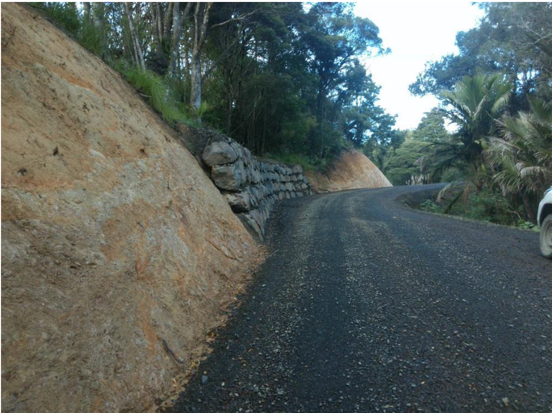
Over slip repair completed on Waiotehue Road by Far North Roading crew.
