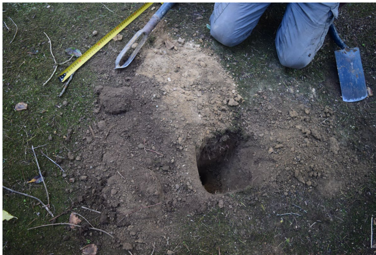
PLATE 20. THE COMPACTED MADE SOIL FROM TP11
