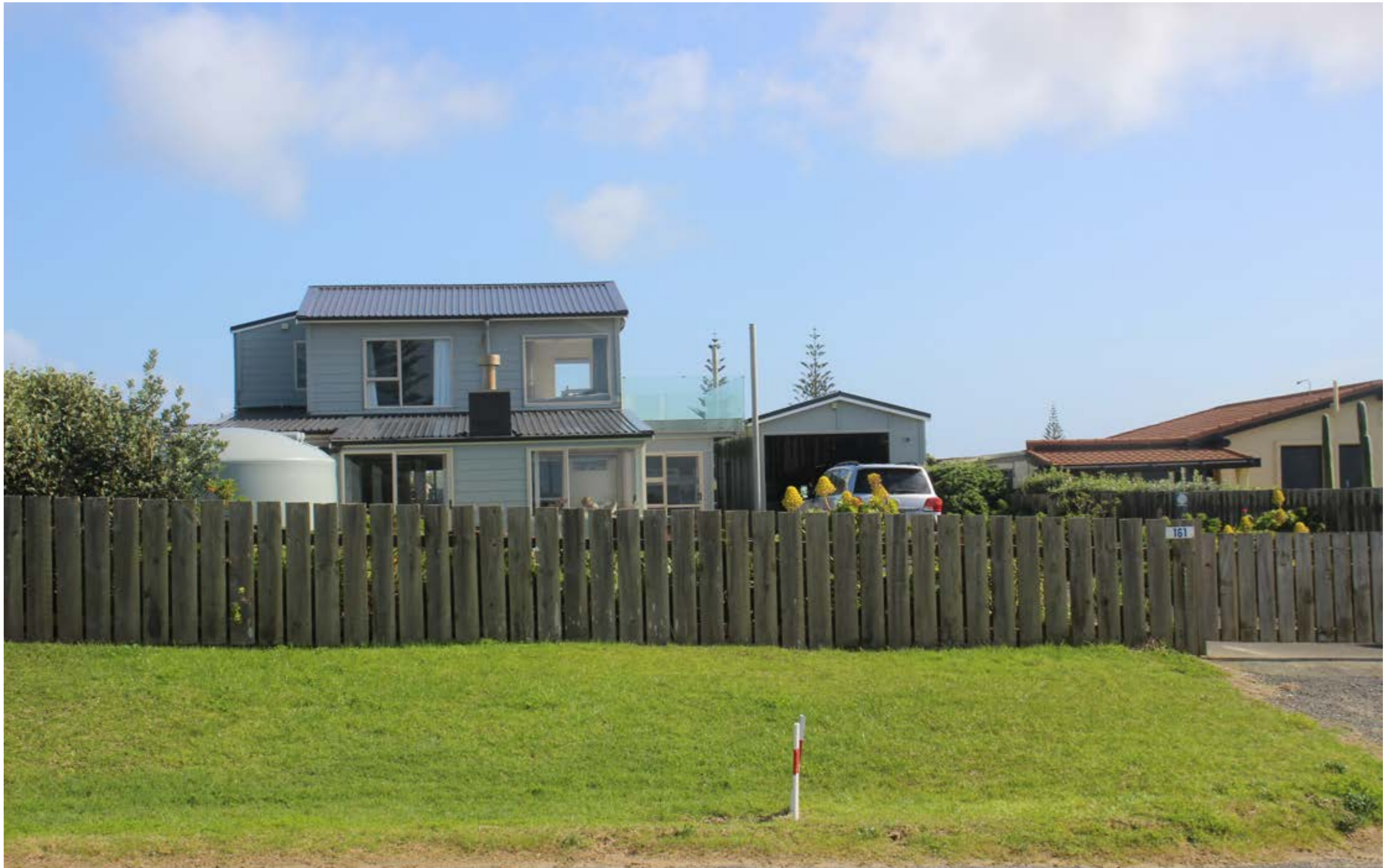
Photo 5: #161 Ramp Road from road
