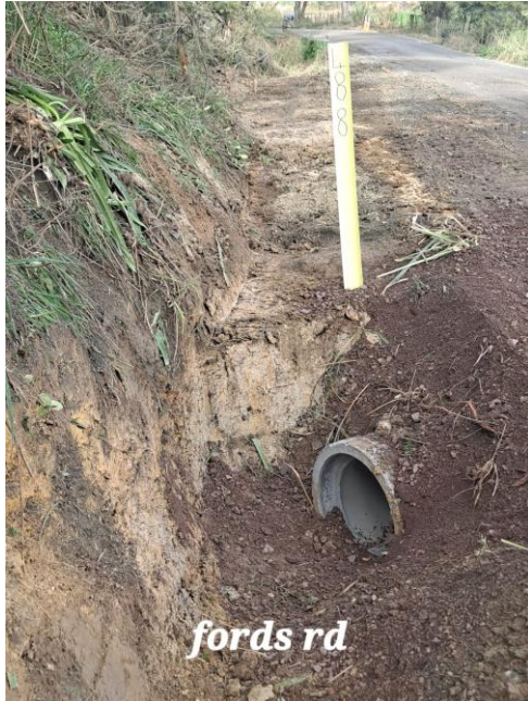
Fords Road / Paiaka Road (headwalls still to be installed)
