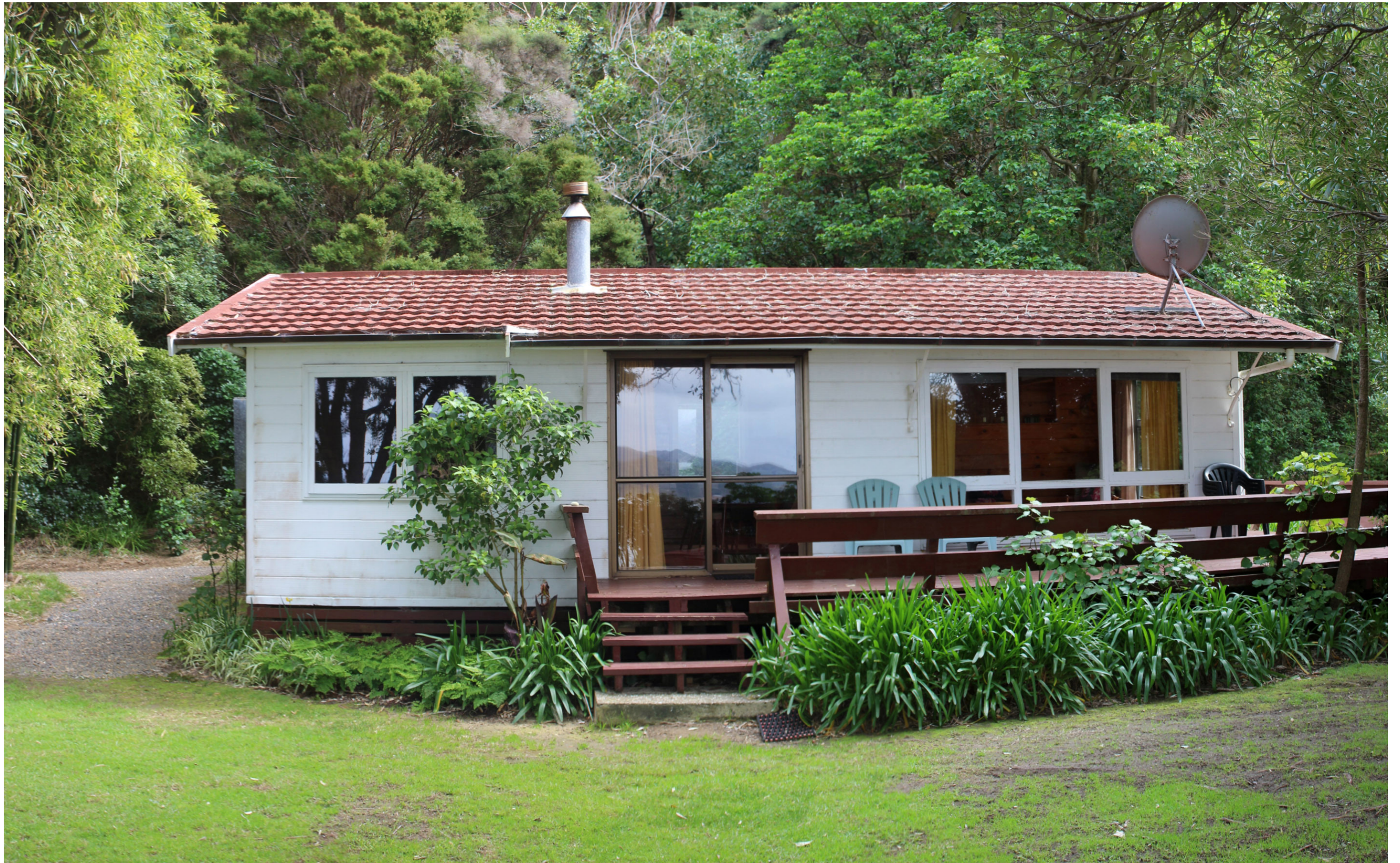
Photo 5: Existing Lockwood (red-roofed) building
