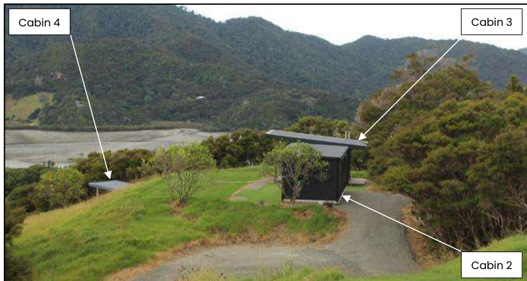
Figure 12. Cabins 2 – 4 (Source: SCLA).
