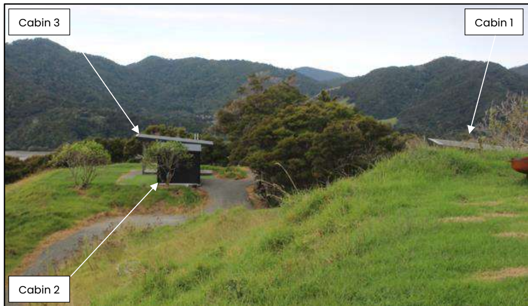
Figure 11. Cabins 1 – 3 (Source: SCLA).
