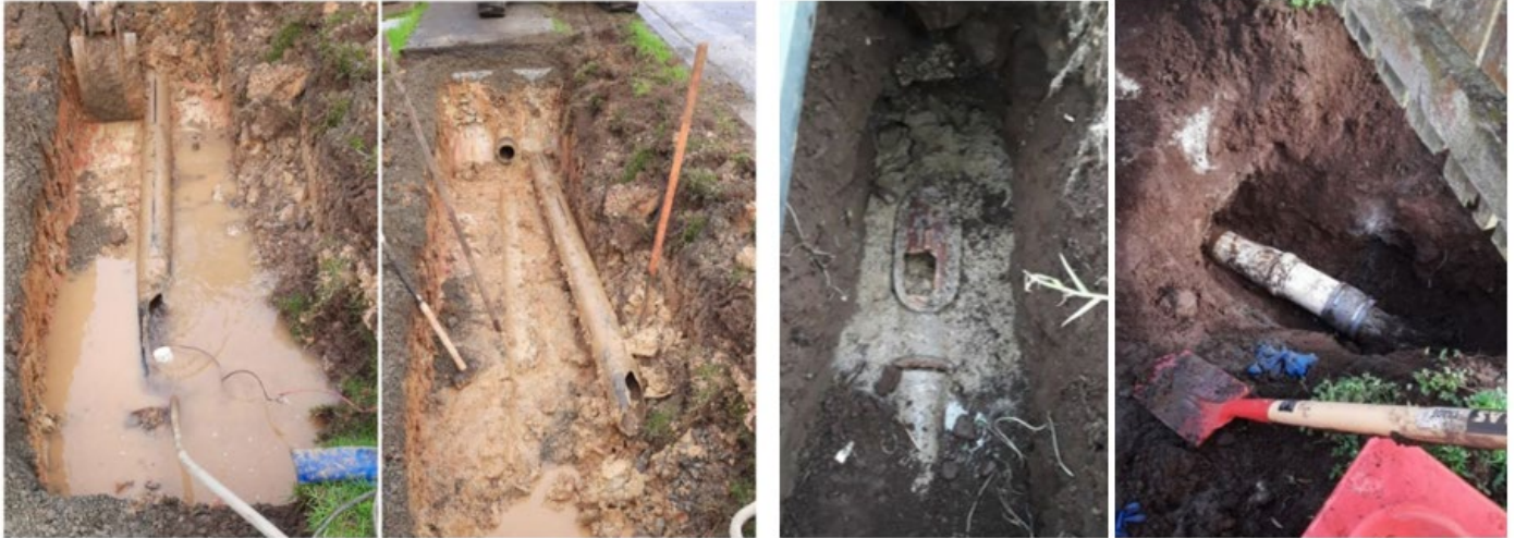
Water line repair, Redan Road, Kaitaia
