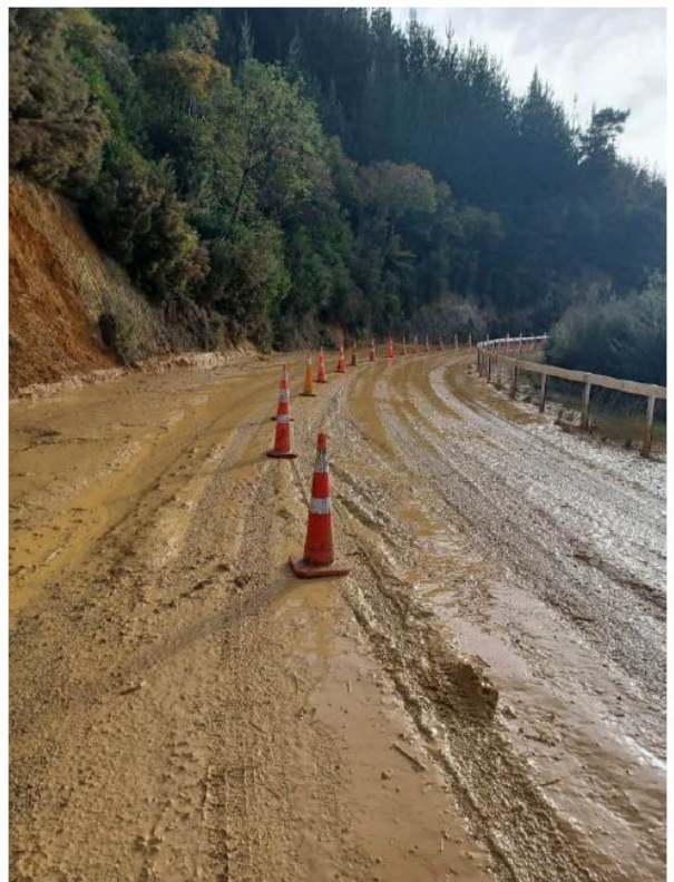
Waiare Rd – Sloppy slip site. Material has continued to wash down out of the forestry. With no option to clean the road as the slurry continued for days afterwards the road was reduced to a single lane.
