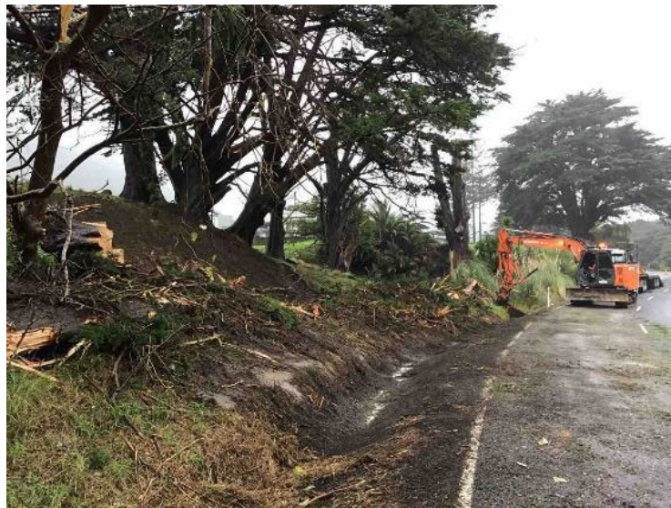
Figure 8: Kaitaia Awaroa Rd Fallen Tree Removal
