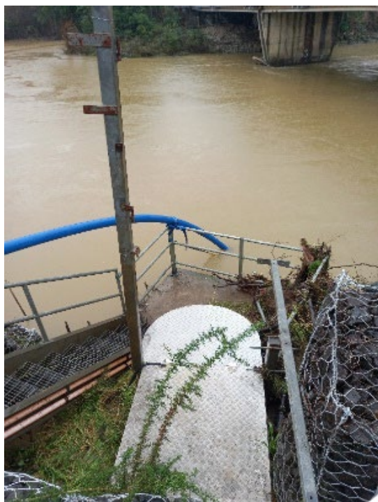
Paihia WTP: Installation of a spare pump in the Waitangi river.
