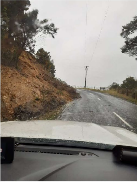
Ngapipito Rd – Large Slip cleared late in the month with a bench set up to catch further unstable material
