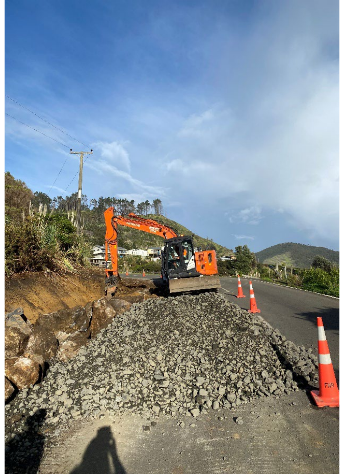
Progress of initial clearing and drain/swale preparation on the Foreshore Road heading up to Te Kohanga
