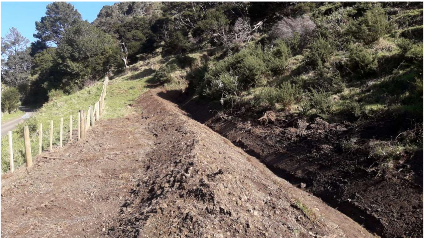
Waitemarama Gorge Rd – Large under slip with a lot of details to think about. Initial temporary repair works to reduce chance of further slippage, how to retreat a corner, boundaries, and surveying to confirm, residents’ permission to enter property to shape private spill way (above photo), service locates in an emergency, culvert
