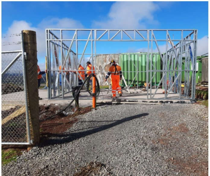
Monument Bore – new build to house equipment
