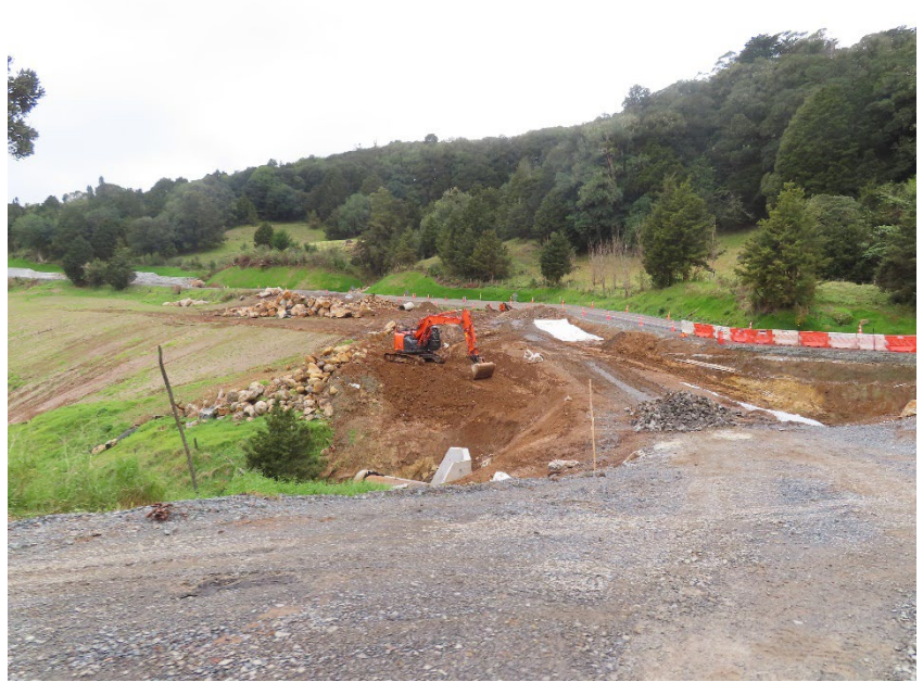
Figure 1) Temporary Road, 2100 diameter culvert and new road alignment
