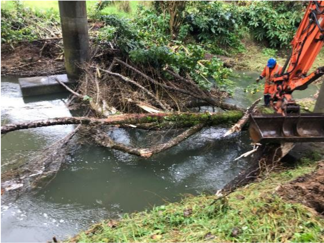
Figure 10: Takahue Rd Bridge Debris Removal
