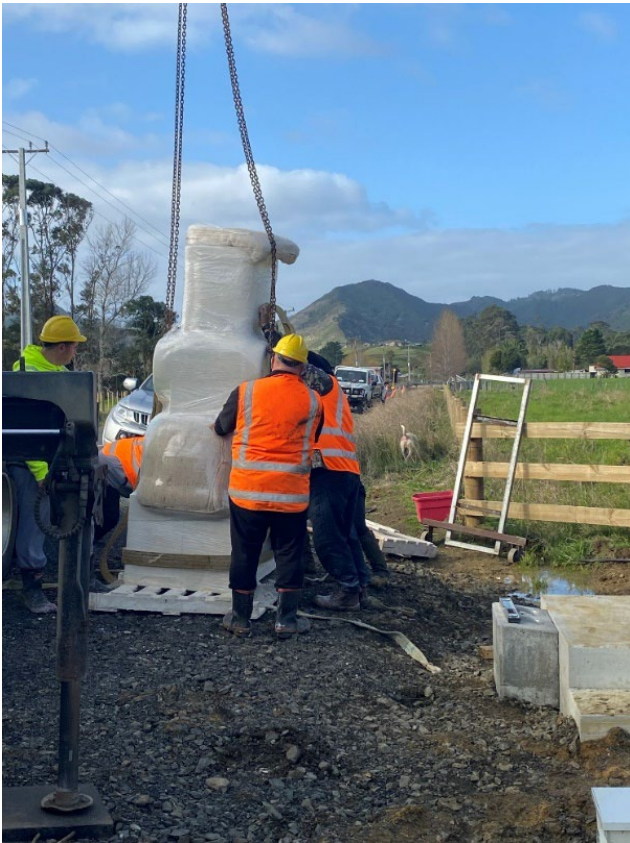
Above: Moving stonework into place
