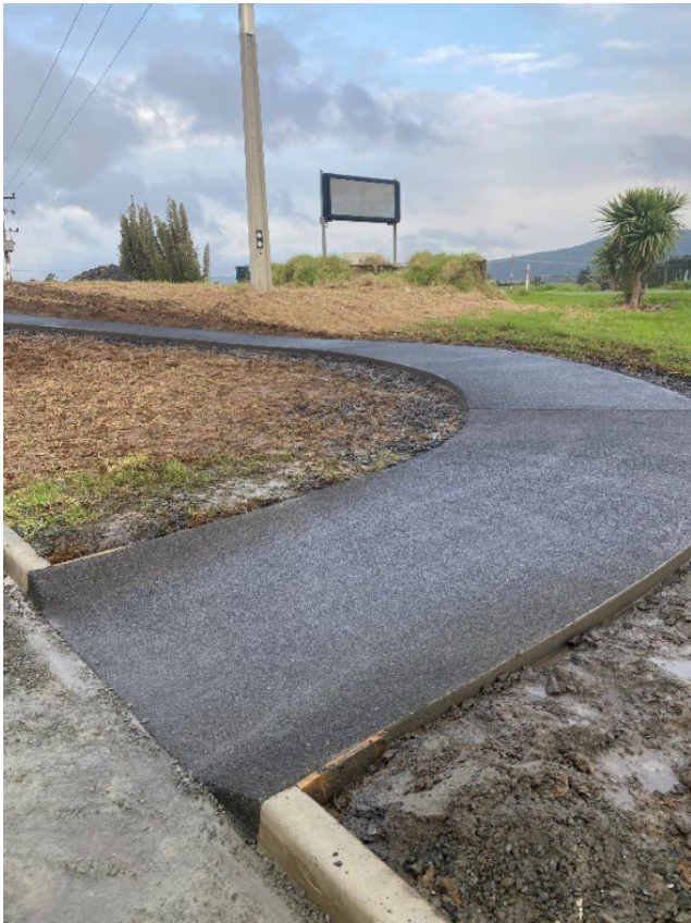
Below: Concreted from carpark to pou
