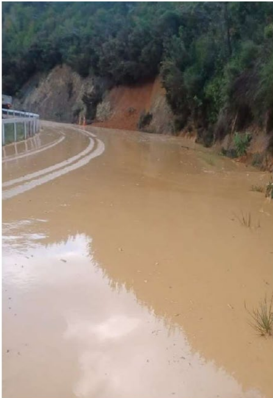
Waiare Rd – Sloppy slip site. Material has continued to wash down out of the forestry. With no option to clean the road as the slurry continued for days afterwards the road was reduced to a single lane.
