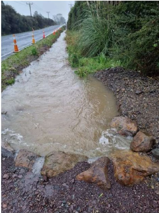
Inlet and Outlet on 25/7/22. Note the rapids on the outlets showing the pressure the lines are under.
