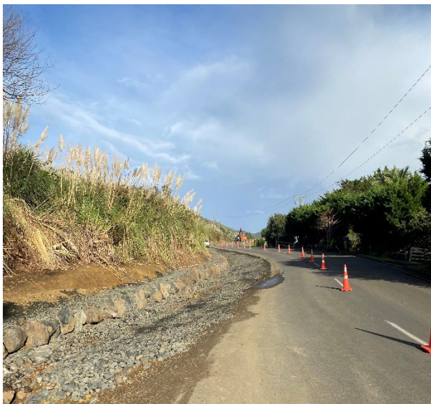
Progress of initial clearing and drain/swale preparation on the Foreshore Road heading up to Te Kohanga
