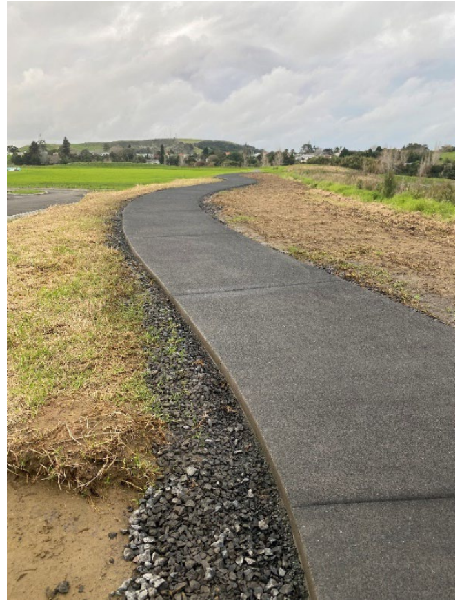
Above: Curved path concreted to join loop
