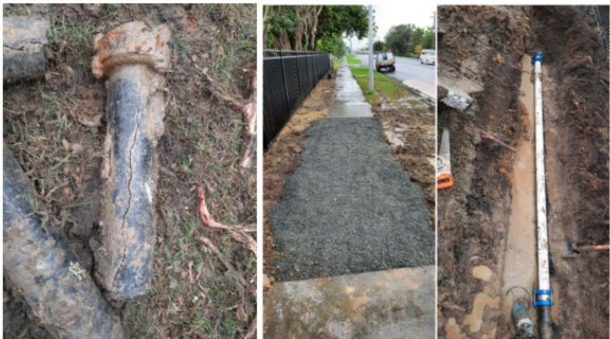
AC Water main repair on North Rd Kaitaia
