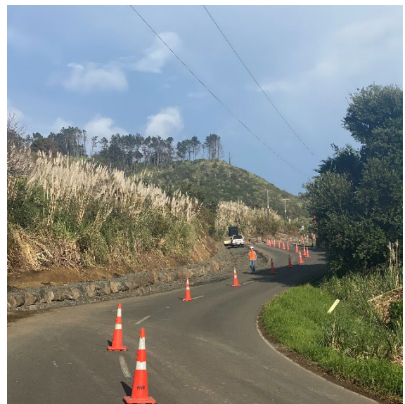
Progress of initial clearing and drain/swale preparation on the Foreshore Road heading up to Te Kohanga
