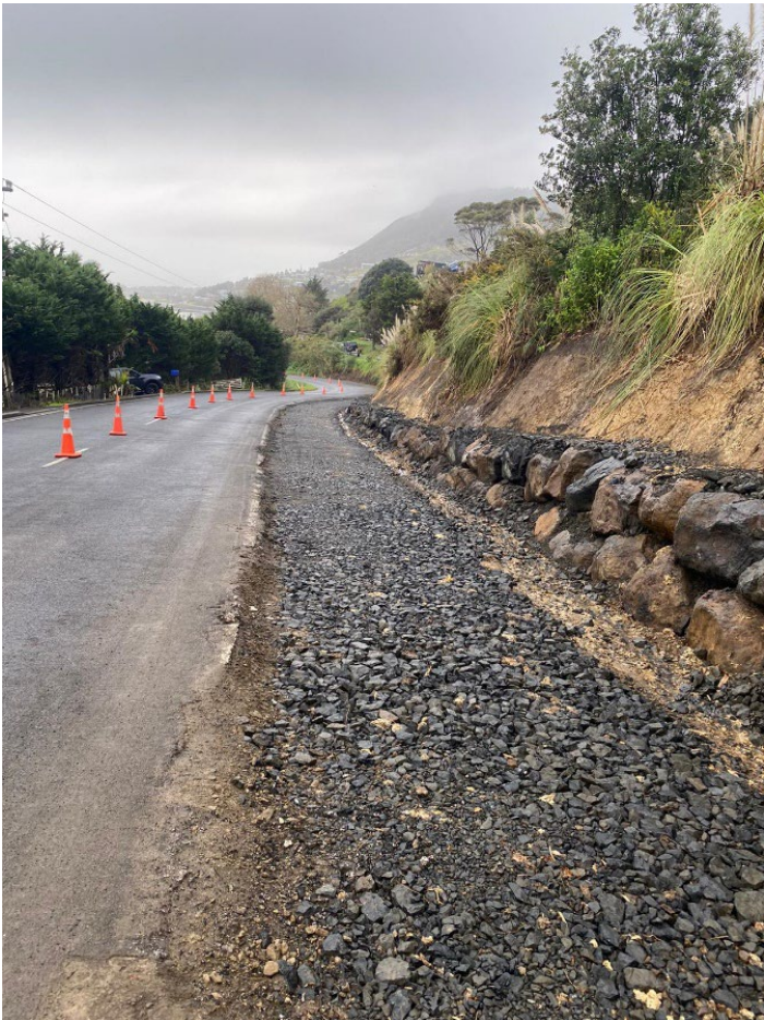
Progress of initial clearing and drain/swale preparation on the Foreshore Road heading up to Te Kohanga
