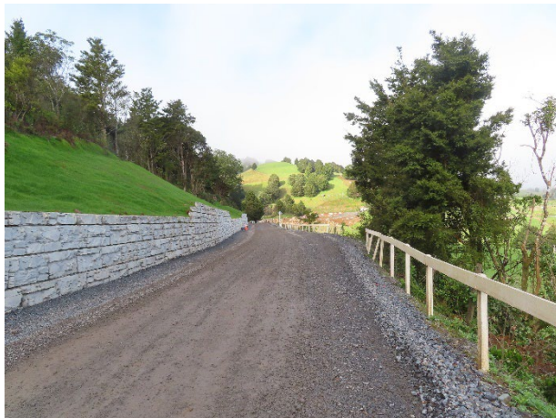
Figure 2) Mass block wall and hydroseeding
