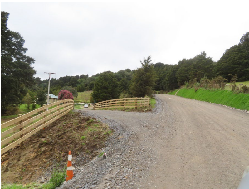
Figure 3) Landowner's accessway and permanent fencing upgrade works well underway
