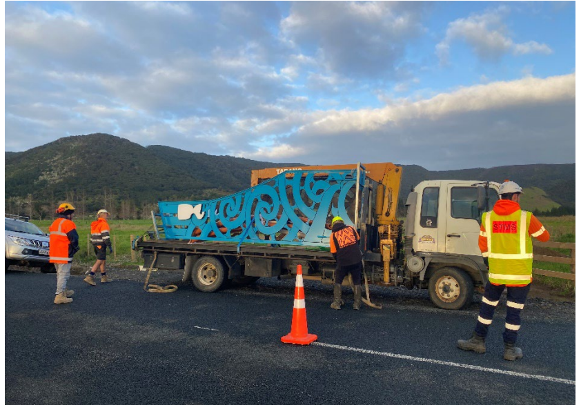
Above: First truck arrived with the steel work from Aravisions
