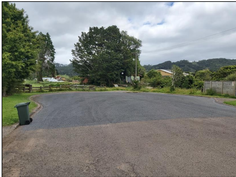
Figure 5: Existing sealed Bisset Road turning head (Chester 05/09/2023)
