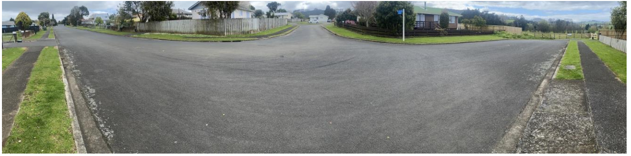
Photo 3. A panorama of Harold Avenue from south (left) to north centred on Rimu Place (centre). The current end of Harold Avenue is at upper right.
