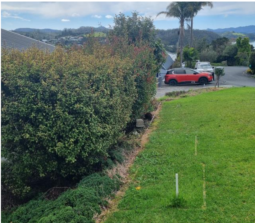
The location of the proposed retaining wall. The extent of the wall will reach the white peg and follow the line to the grey post in the distance (behind the car). The peg represents the property boundary with the wall angling into the road reserve at the far end.
