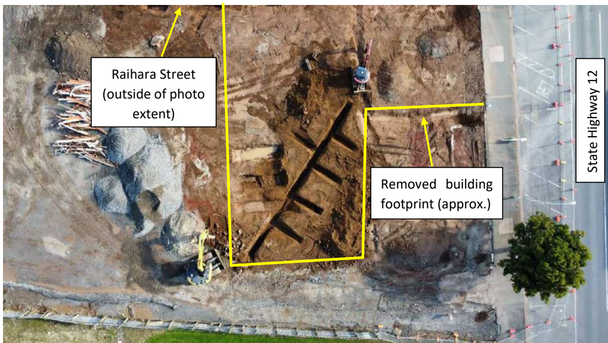
Figure 1 - Drone Photograph Prior to Backfilling
