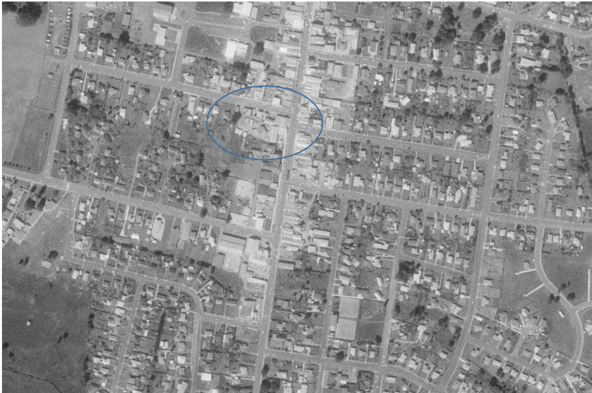
Figure 7 – Aerial Photograph – 1977 (Source: Retro Lens)
