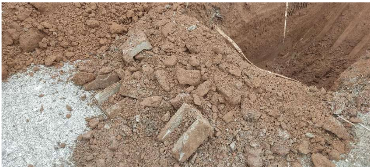
Figure 4 Excavated 'U' drains.
