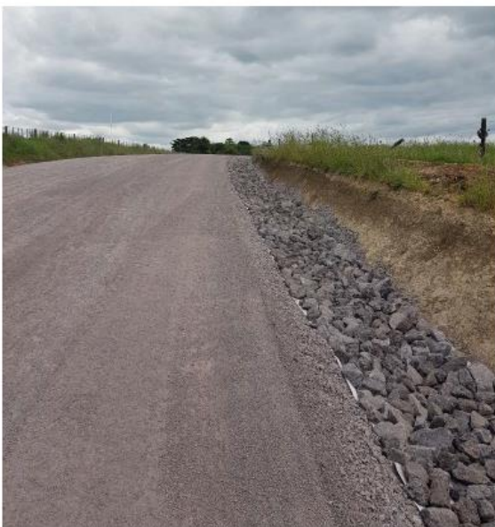
Ruapekapeka Rd – Earthworks in action, rip rap installation and stabilisation.
