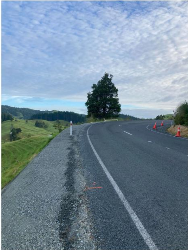
Figure 21: Peria Rd Seal Extension Section 3 Guardrail
