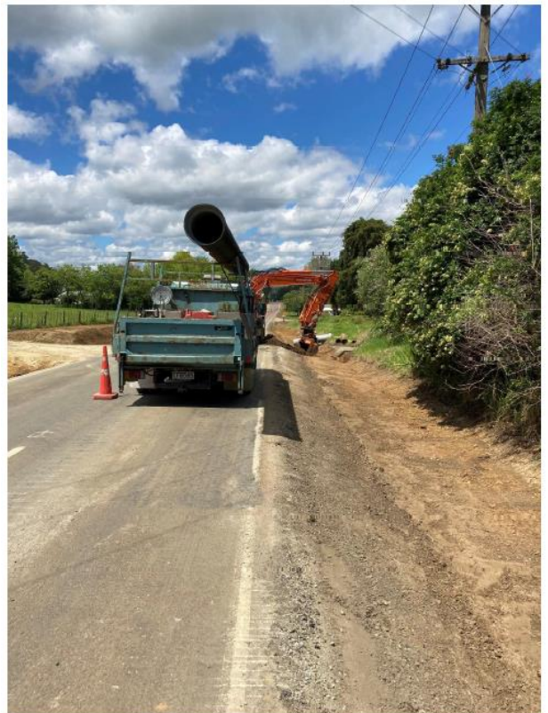
Figure 10: Oruru Rd Site 1 Rehab Drainage
