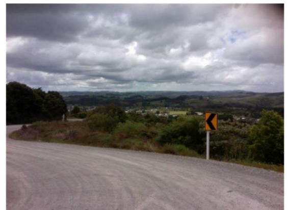
Hautapu Rd – Installed chevron and post
