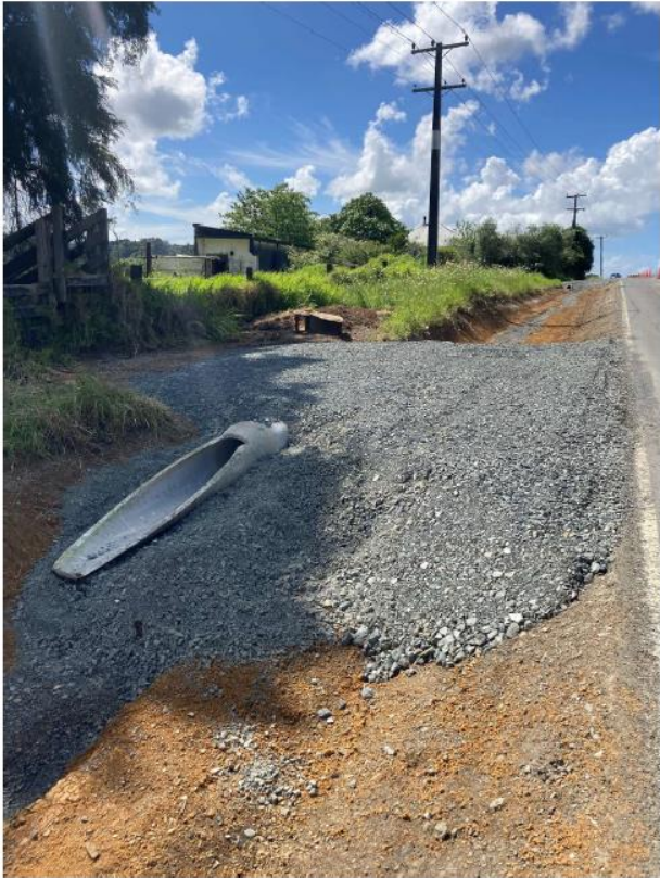
Figure 11: Oruru Rd Site 1 Rehab Drainage
