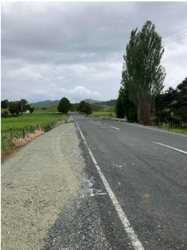
Figure 17: Peria Rd Seal Extension Section 1 Guardrail widening
