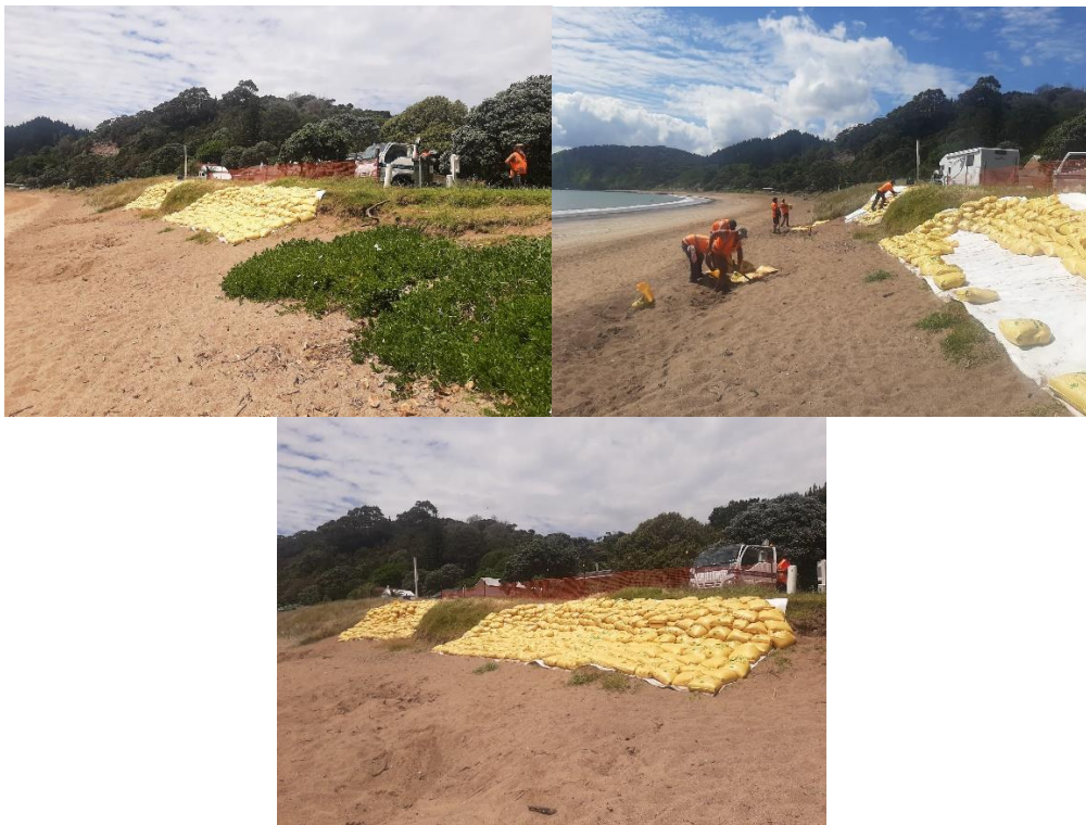
Erosion control work – Long Beach Koiwi Site, Russell
