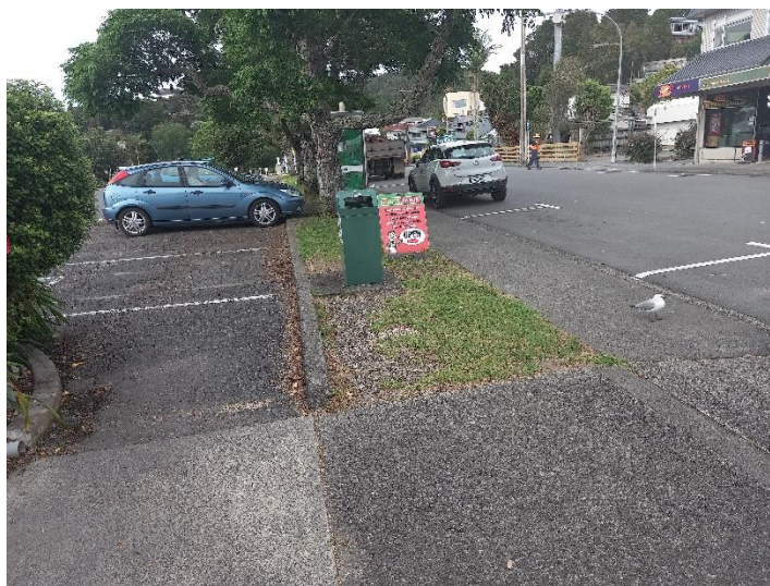
Williams Rd potential trip hazard location
