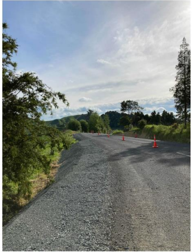
Figure 20: Peria Rd Seal Extension Section 3 Guardrail widening
