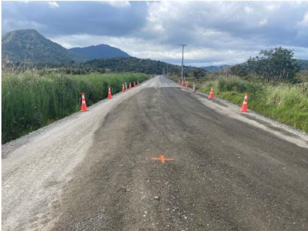
Figure 5: Go1 Pangaru Bridge Approach
