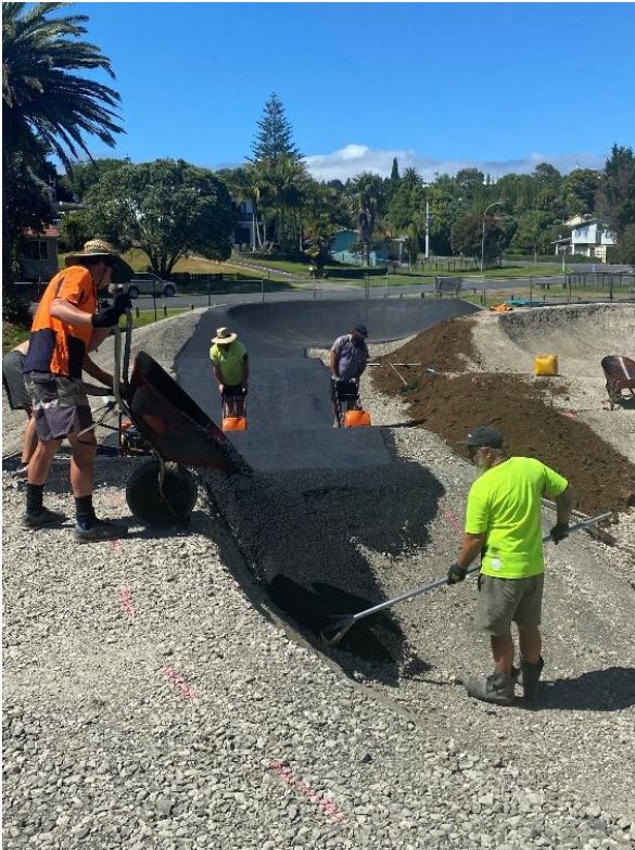
Labourers assisting with asphaltting
