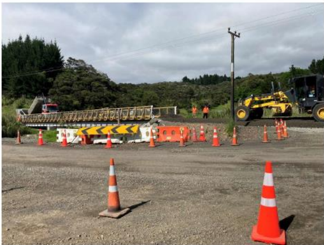
Figure 6: Go1 Pangaru Bridge Approach
