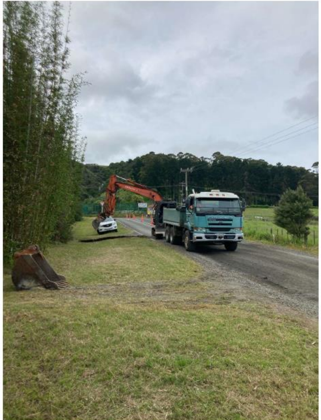
Figure 22: Brass Rd Seal Extension Clearing
