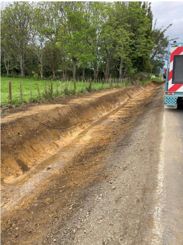
Figure 9: Oruru Rd Site 1 Rehab Site Clearing
