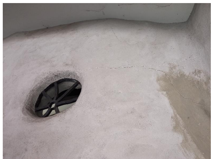
Hundertwasser toilets - cracking in plaster work and wooden beams pulling away from neighbouring building
