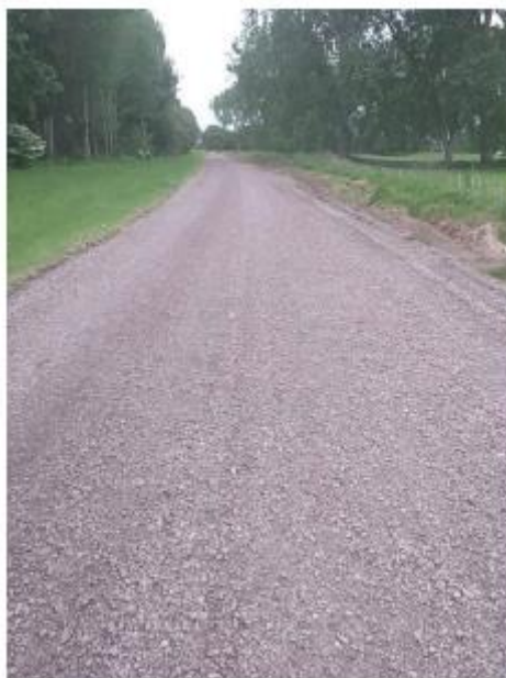
Smith Rd,– Maintenance Metalling
