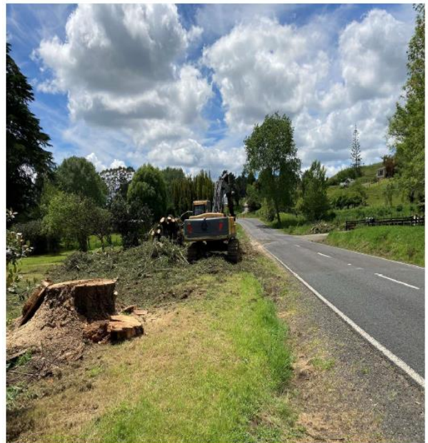
Figure 14: Oruru Rd Rehab Site 2 Tree felling
