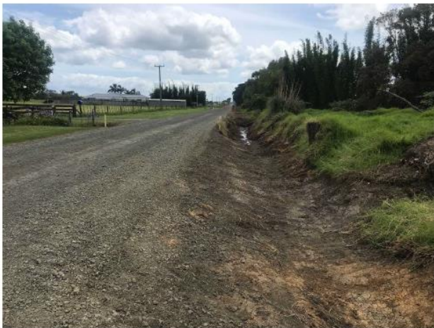
Figure 23: Brass Rd Seal Extension Clearing
