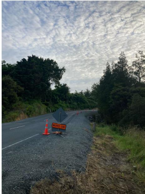
Figure 21: Peria Rd Seal Extension Section 3 Guardrail
