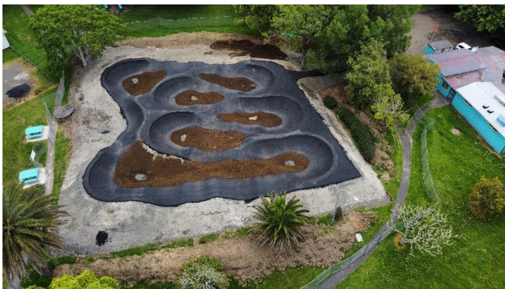
Birds eye view after track completion but prior to landscaping
