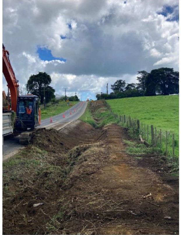
Figure 8: Oruru Rd Site 1 Rehab Site Clearing
