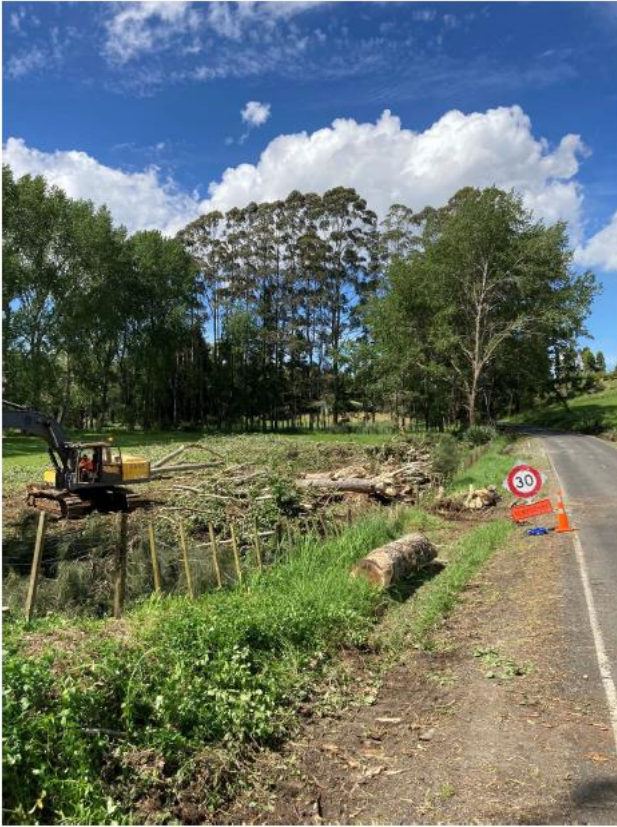
Figure 15: Oruru Rd Rehab Site 2 Tree felling
