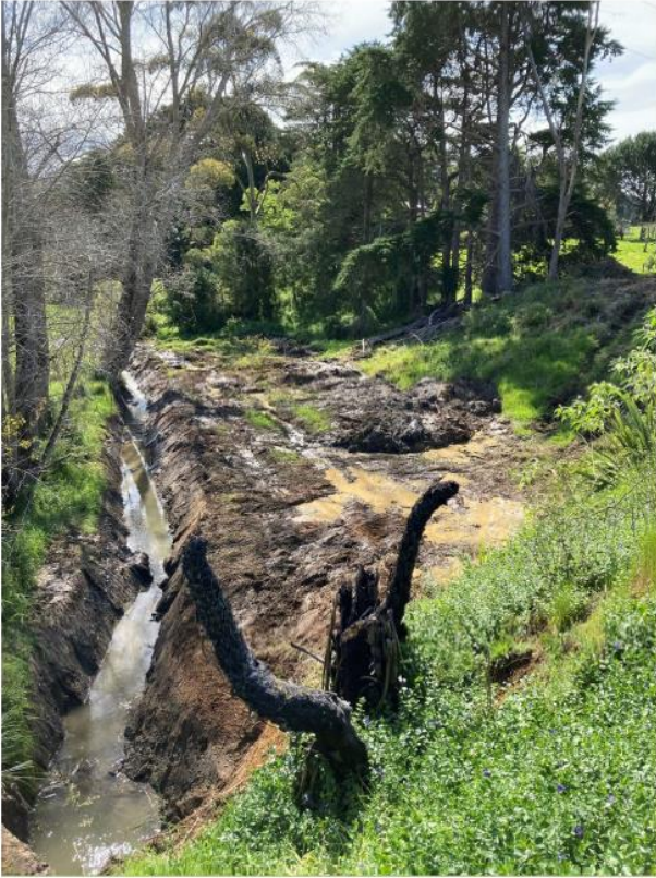
Figure 7: Oruru Rd Site 1 Rehab Culvert Clearing
