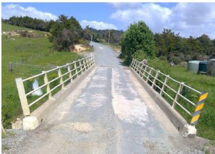
Horahora Rd – Bridge Deck Cleaning
