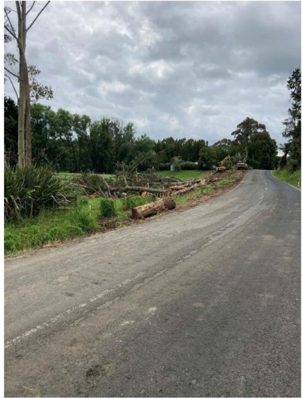
Figure 16: Oruru Rd Rehab Site 2 Tree felling
