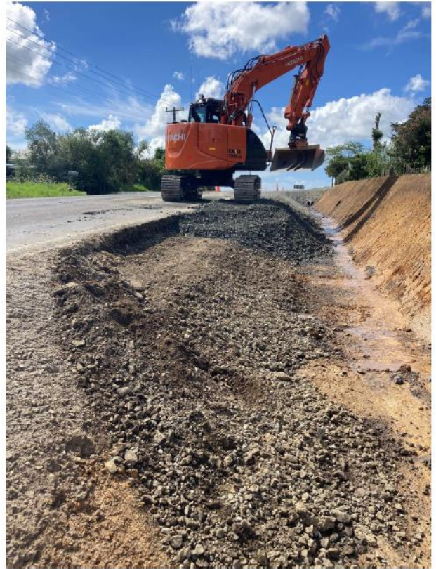
Figure 12: Oruru Rd Site 1 Rehab Shoulder undercuts
