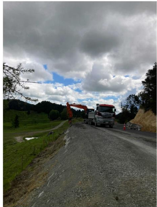
Figure 18: Peria Rd Seal Extension Section 3 Guardrail widening
