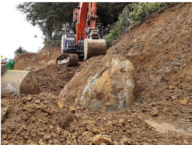
Excavator exposing rocks beneath the bank
