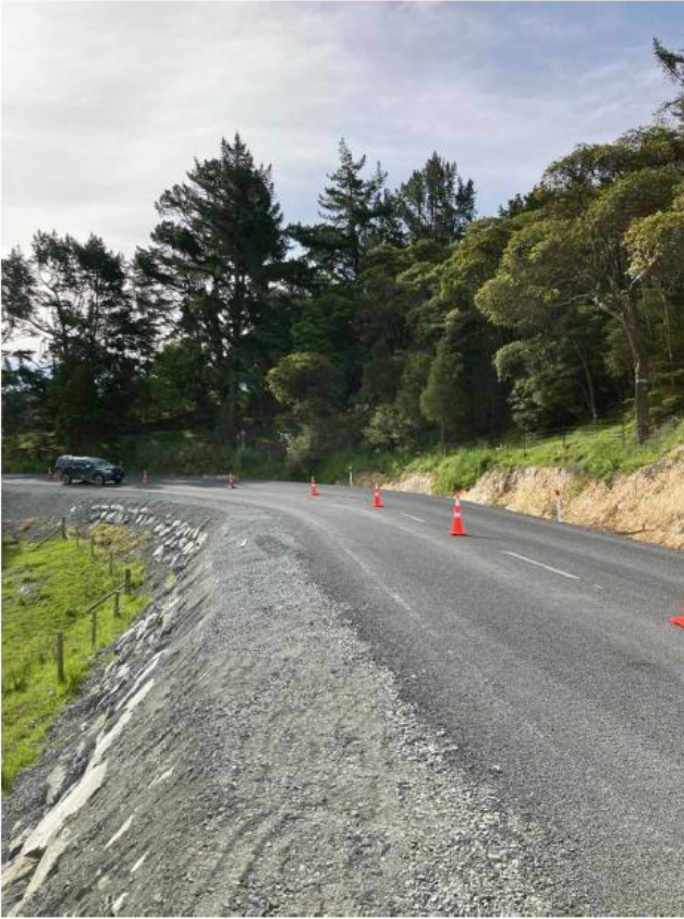
Figure 19: Peria Rd Seal Extension Section 3 Guardrail widening
