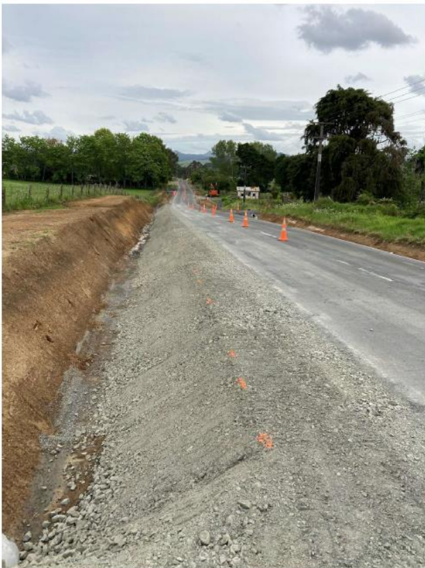
Figure 13: Oruru Rd Site 1 Rehab Shoulder undercuts
