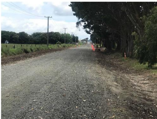
Figure 24: Brass Rd Seal Extension Clearing
