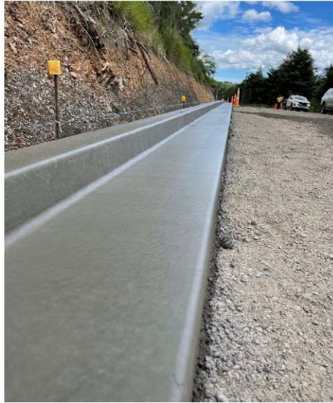
Ngapipito Rd – New Kerb and channel
