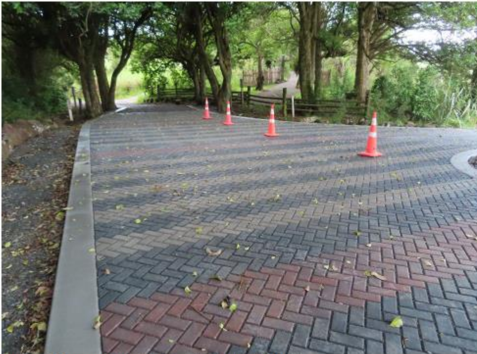
Figure 4) Monument Road Intersection Paving & Kerbing
