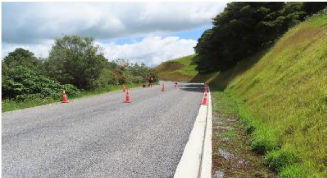
Figure 7) Pavement prepped and kerb and channel installed
