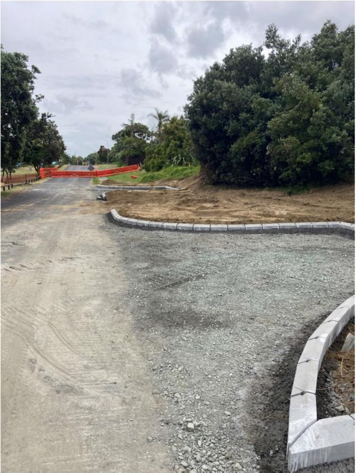
Korora Street Road Closure / Carpark Upgrade
