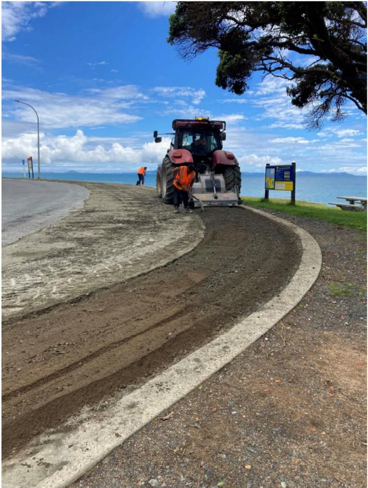
Cable Bay Carpark Upgrade / Widening
