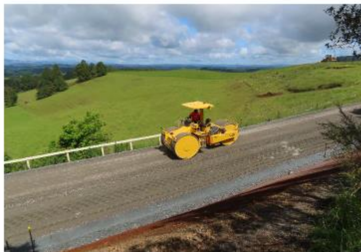
Figure 6) Pavement stabilisation - roller compaction
