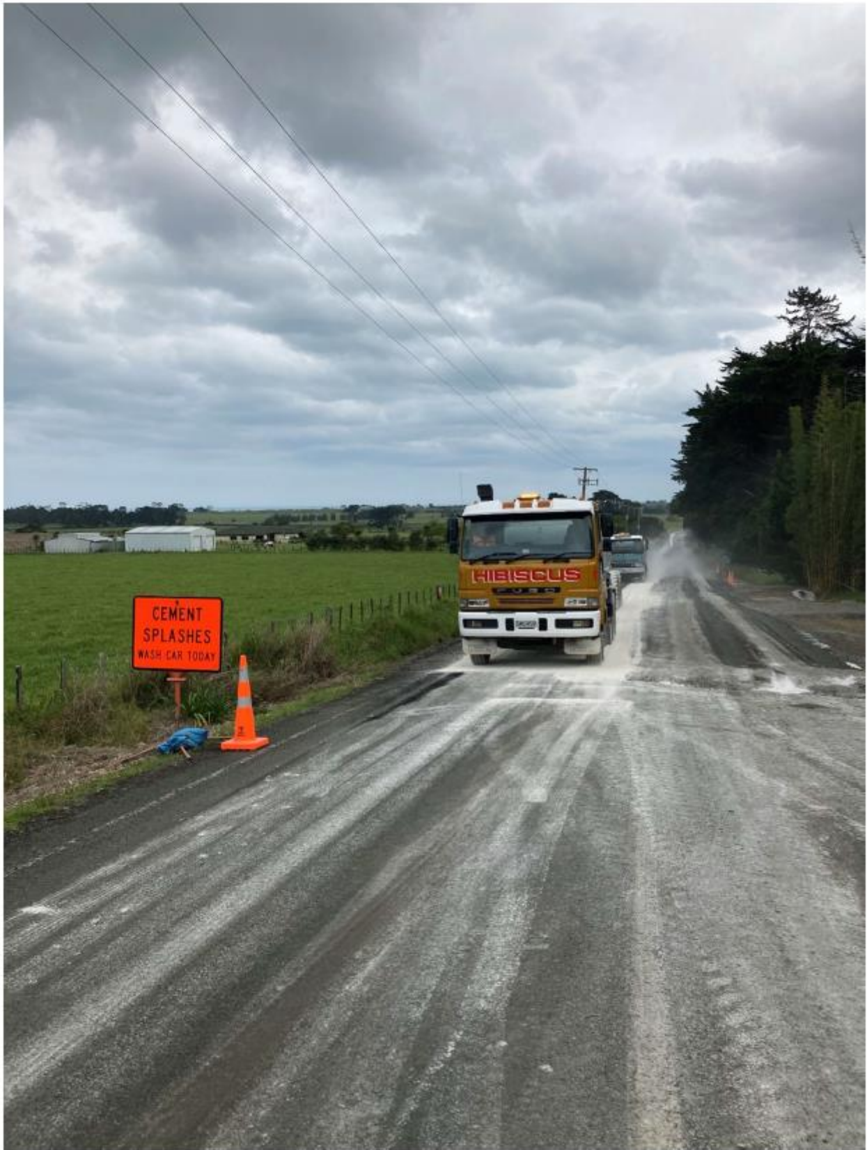
Pavement Stabilisation on the Brass Road Seal Extension
