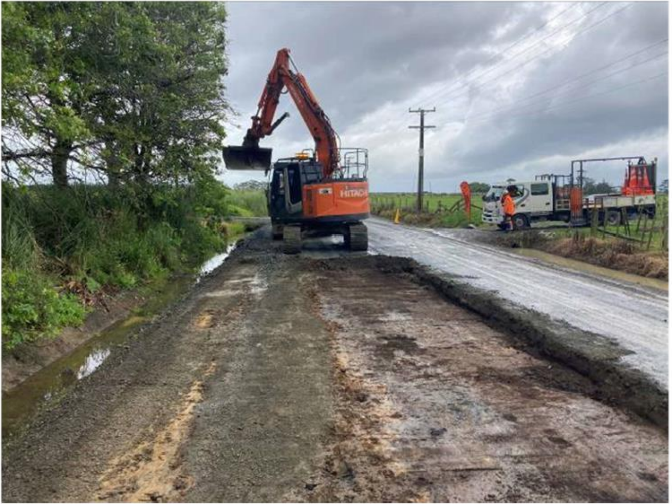
Unahi Rd Seal Extension Pavement Tie-ins
