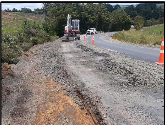
Shoulder check out (Left), Thorne carrying out Scala Penetrometer testing on a dig out.
