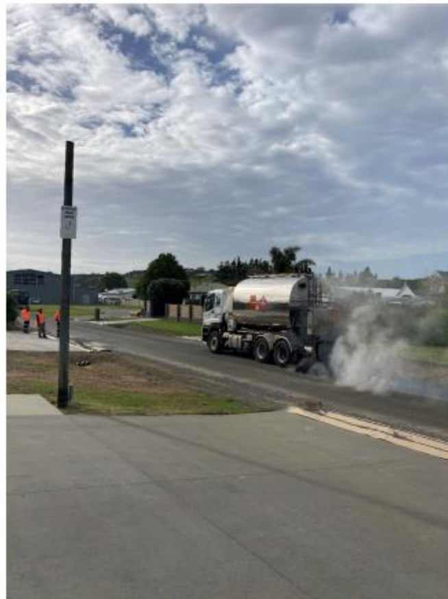
Adamson Rd Drainage Improvements final works
