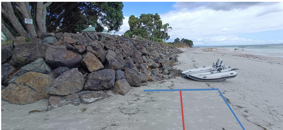
Figure K – Anticipated toe line (beneath sand) of concrete boat ramp
