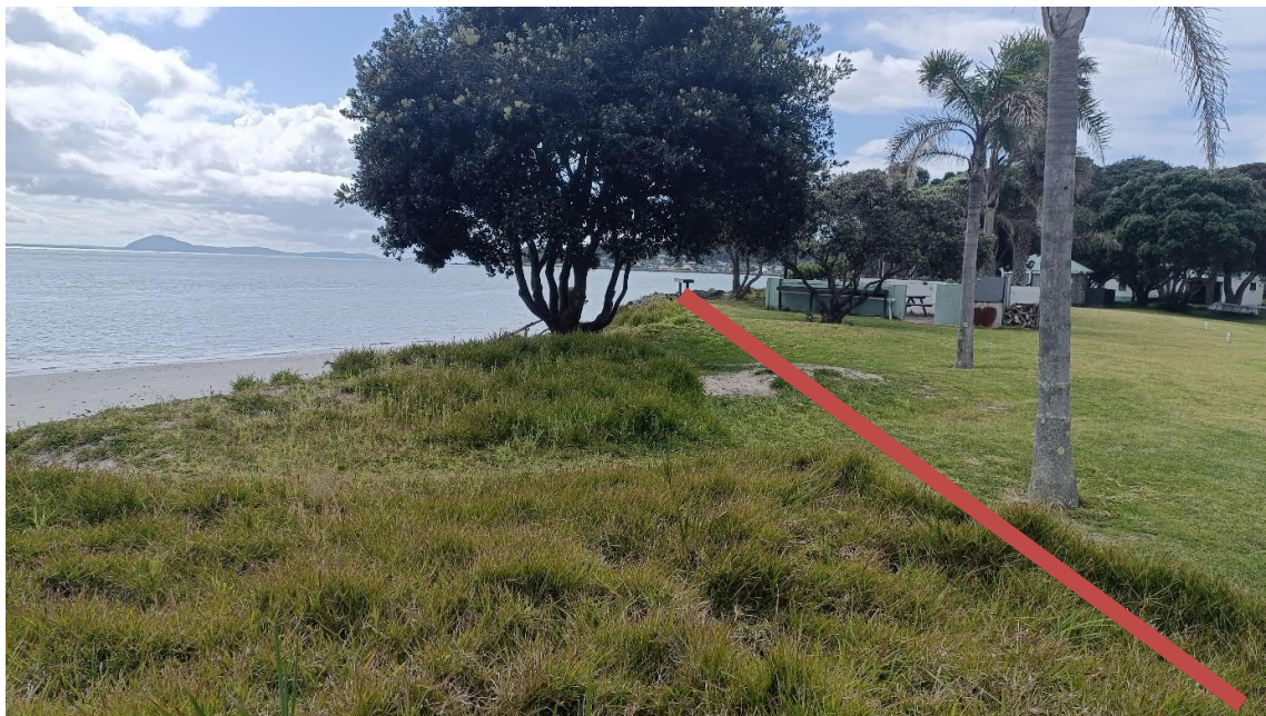
Figure H – Approximate alignment of buried rock revetment on Ghillies Road legal boundary
