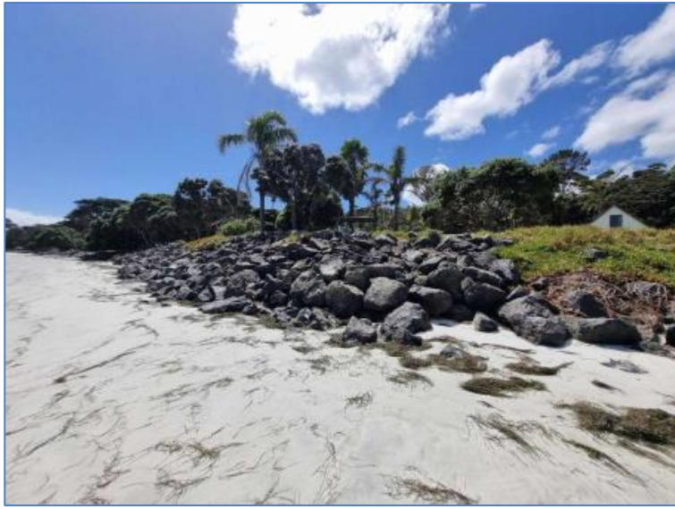
Figure 10: Existing rock revetment wall (Source: HG report)
