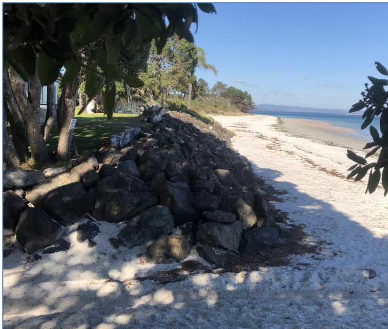
Figure 11: Existing rock revetment wall
