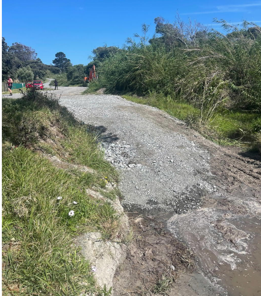
Figure G – Recent works to construct a new ramp at Gillies Road
