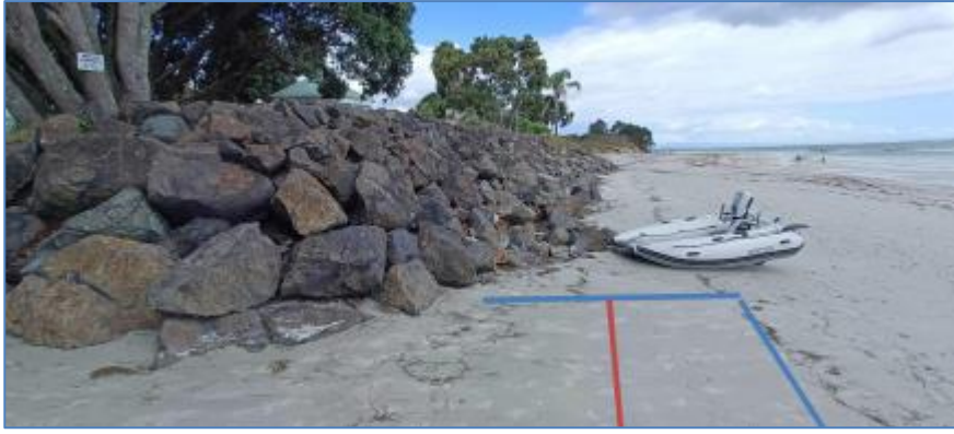
Figure 16: Existing boat ramp toe works (Source: HG report)
