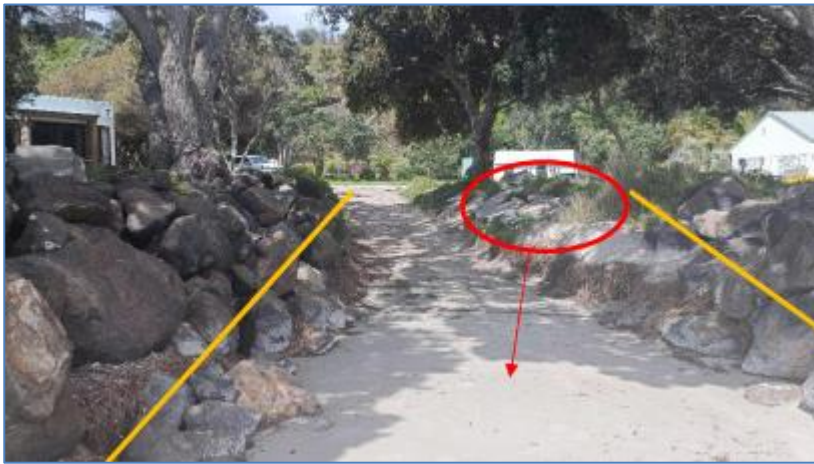
Figure 17: Existing stormwater outlet point (Source: HG report)
