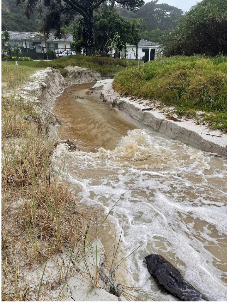
Figure E – Significant flows and associated scour during / following rainfall
