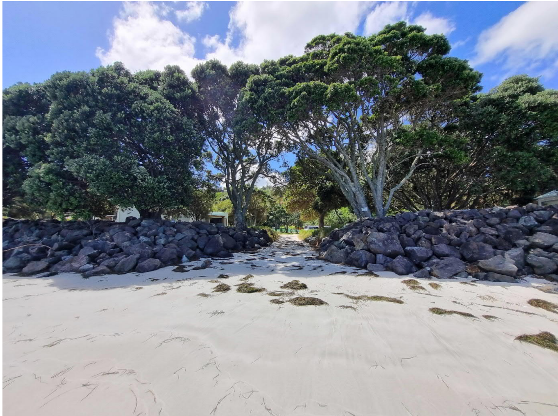
Figure C – Existing private beach vehicle access through existing seawall
