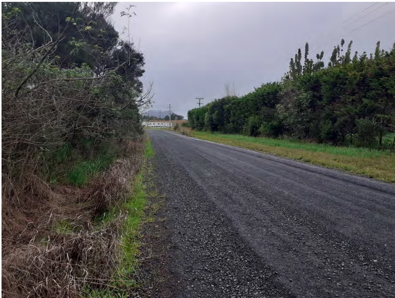
Figure 23: Road 3 – Improved view to the East (removal of vegetation)
