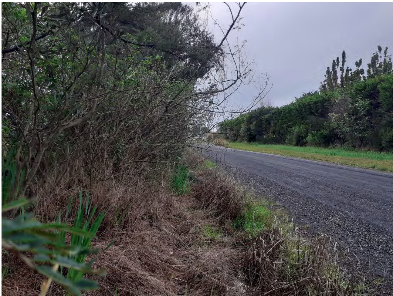
Figure 22: Road 3 – View to the East (constrained by vegetation)
