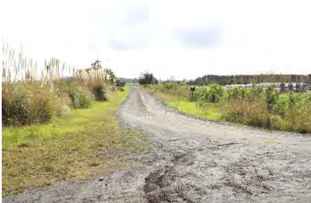
Photograph 1 (P1) – Solar farm construction to the right.
