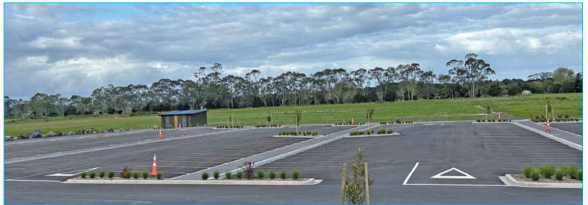
Work on the Te Puāwaitanga sports hub in Waipapa is making positive progress with Phase 1 now complete.
