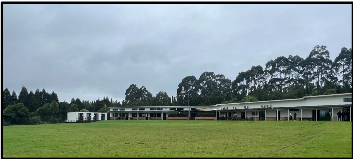
Photo 1: View of existing school looking south east
