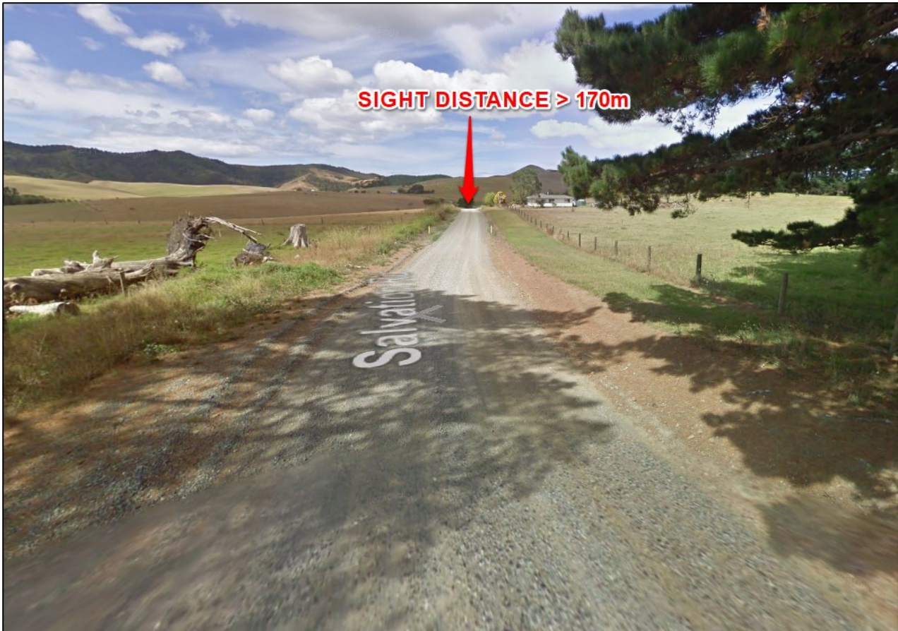
Figure 12: Indicative Sight Distance from Proposed Access Point on Salvation Road Facing Northeast, >170m Sight Distance Available.
