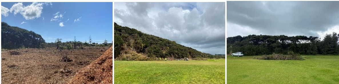
Vegetation clearance/noxious plant removal and ground preparation in Mangawhai Park
