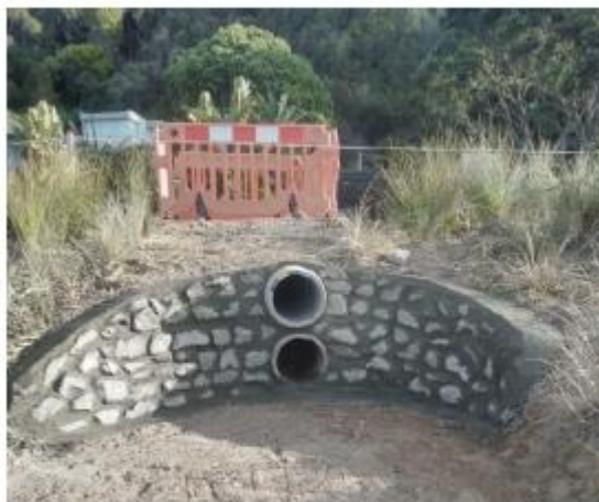
Long Beach – Large Headwall installation
