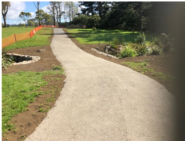
First stage - completed
