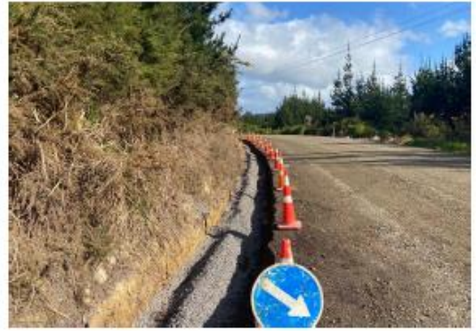
Subsoil/dish channel installation & Pre hoeing – Purerua Rd
