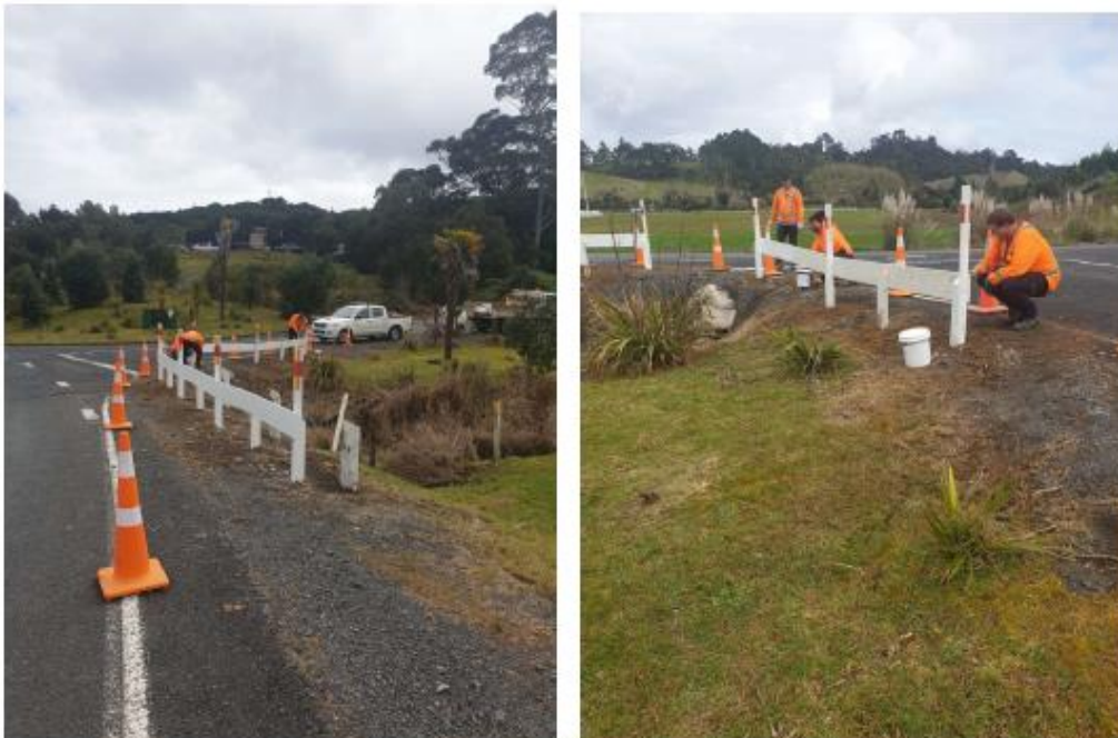
Sight Rail installation – Russell-Whakapara Rd
