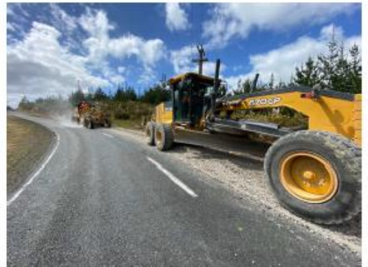
Subsoil/dish channel installation & Pre hoeing – Purerua Rd
