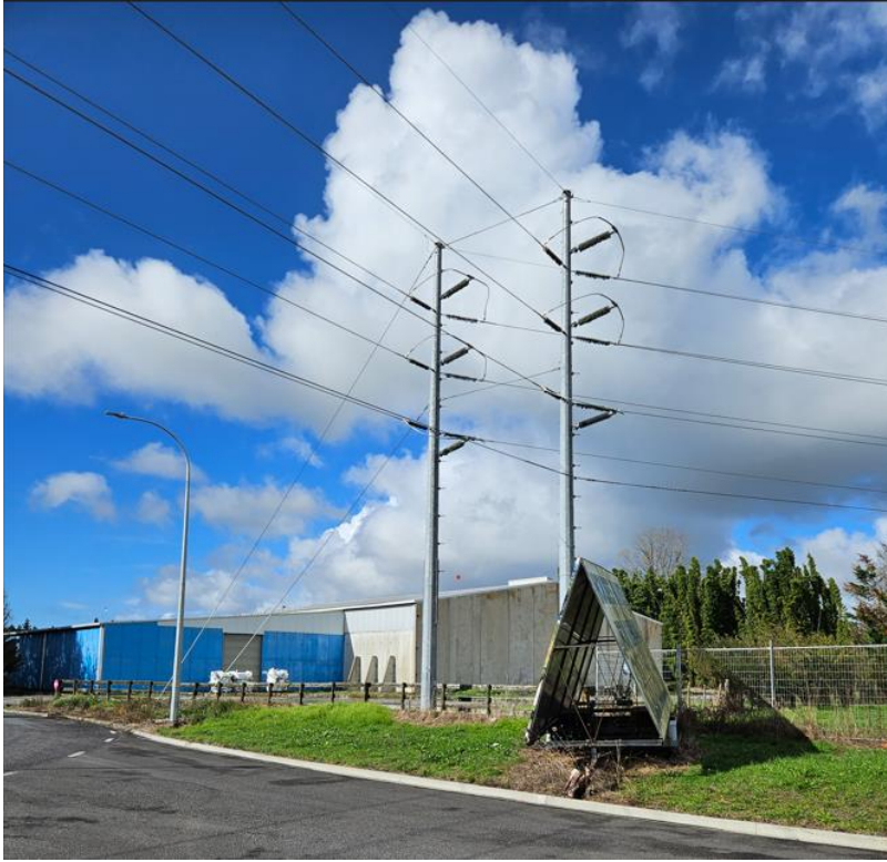
Below: The site's frontage showing the pre-loaded metal area.
