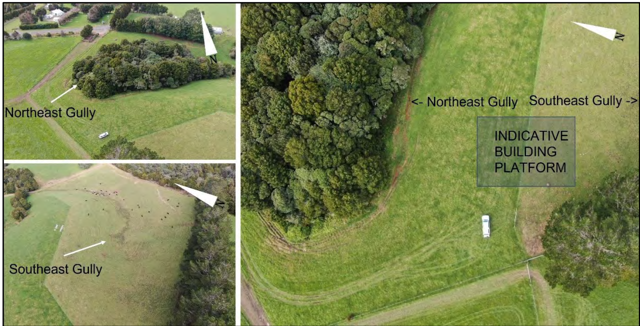
Figure 3 – Drone Photos – Capturing Nominated Building Platform in Lot 1 with the Existing Gullies to the Northeast and Southeast.
