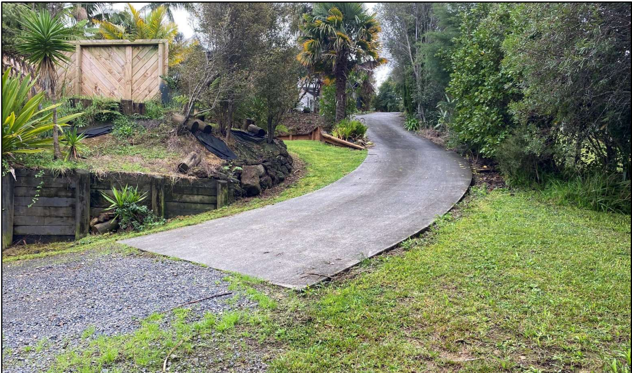
Photo – Taken from the end of concrete driveway. Approximately 22m from the Southern boundary.
