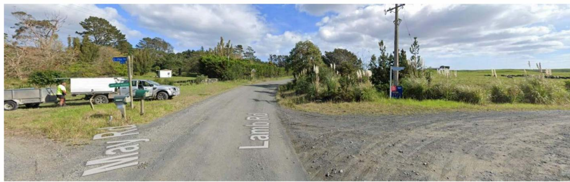
3 01 - View at corner of May rd & Korakanui O Rua Rd NTS
