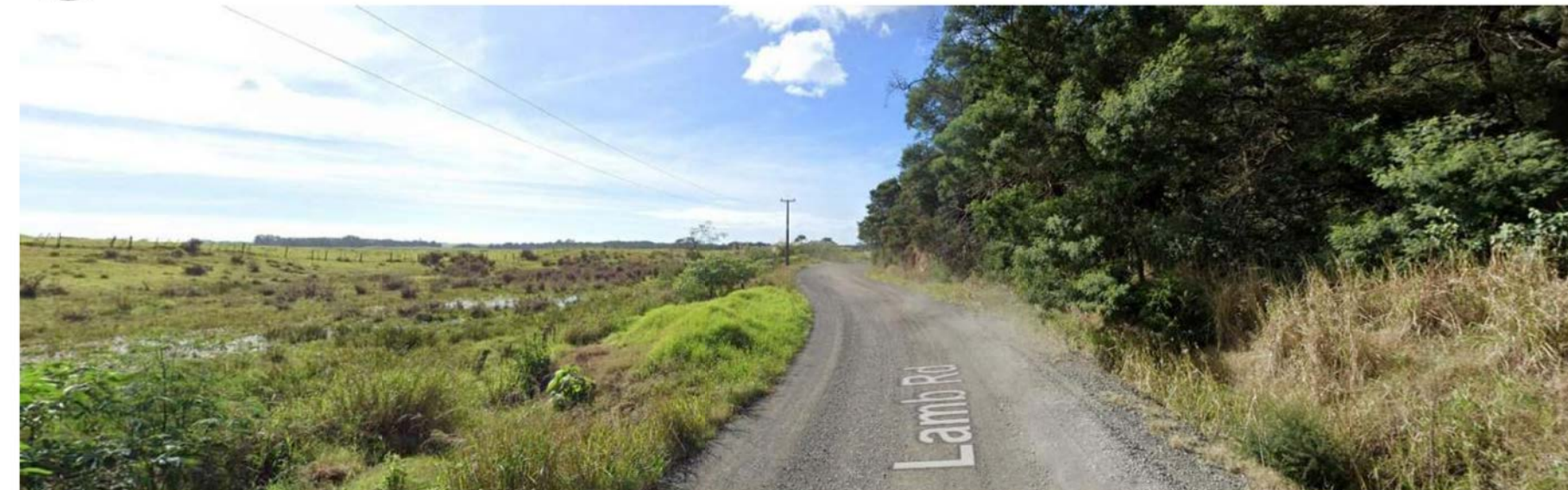
13 12 - View West further along Lamb Rd NTS
