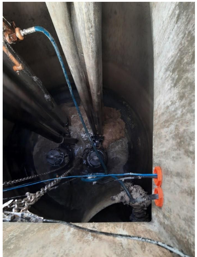
Terminal PS showing rag ball at base
