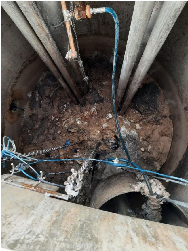
Terminal PS suspended rag and debris
