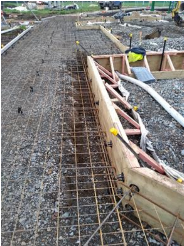
Pavement and playground edging preparation for concrete pour
