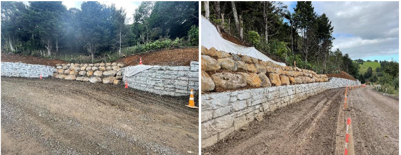
Figure 1) Retaining wall completed with rock walls incorporated.
