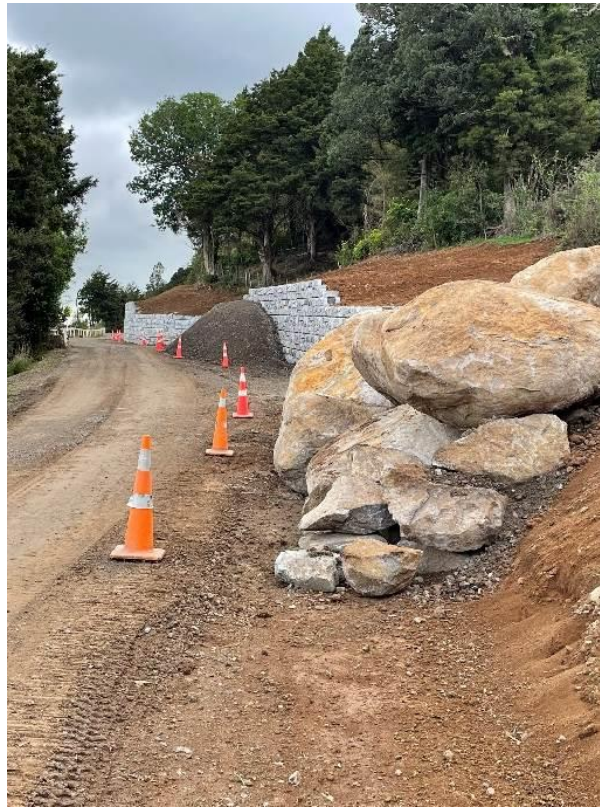
Figure 2) Rocks being incorporated into the large retaining wall.
