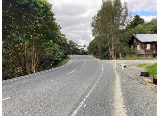
Figure 6: Kohukohu Rd Rehab Seal Complete
