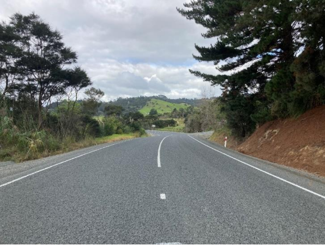
Figure 5: Kohukohu Rd Rehab Seal Complete
