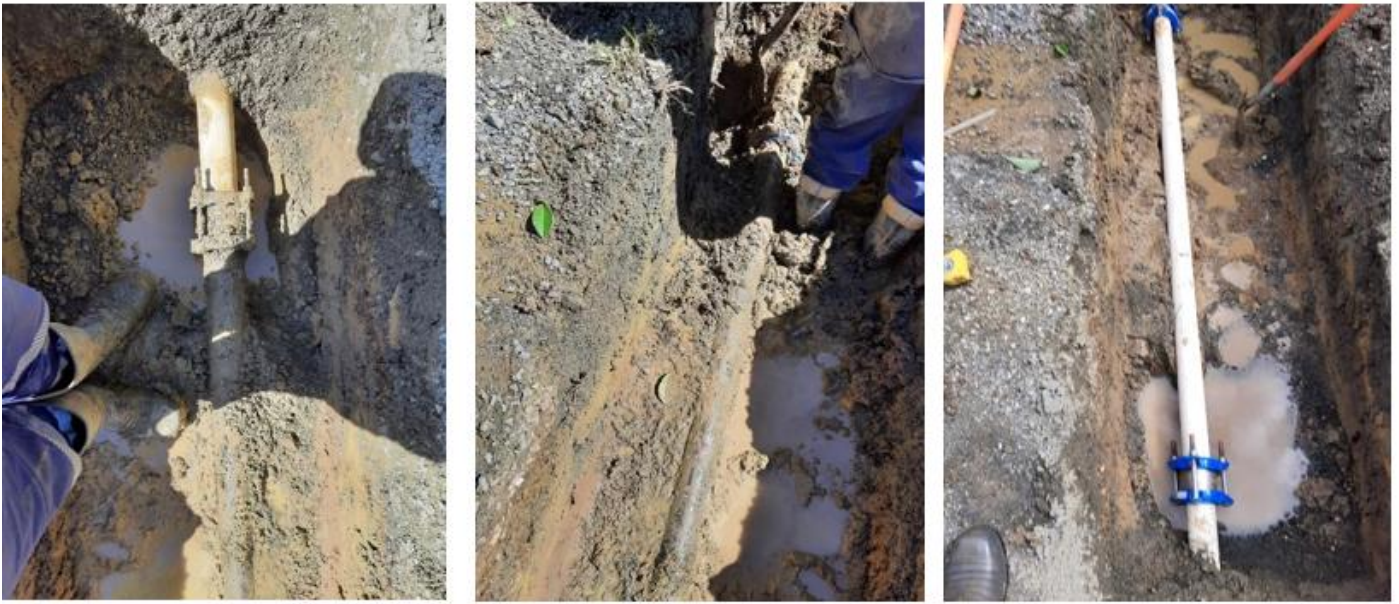
Lake Rd Kaitaia 80mm AC Watermain repair with PVC
