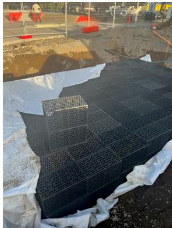
Play equipment installation underway. Stormwater attenuation being installed.
