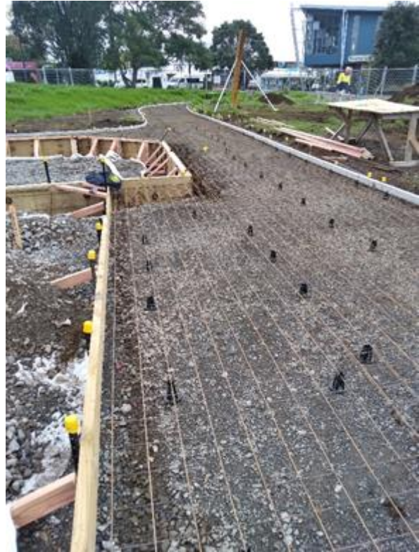
Pavement and playground edging preparation for concrete pour
