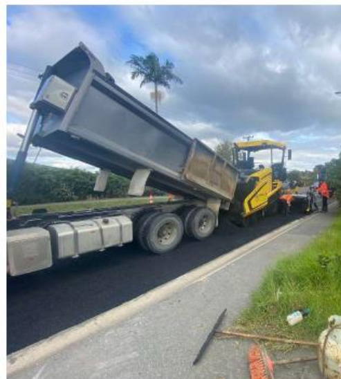
Kerikeri Rd – Deep Lift AC patches
