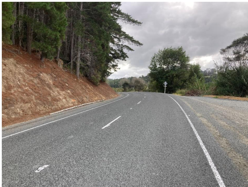
Figure 4: Kohukohu Rd Rehab Seal Complete
