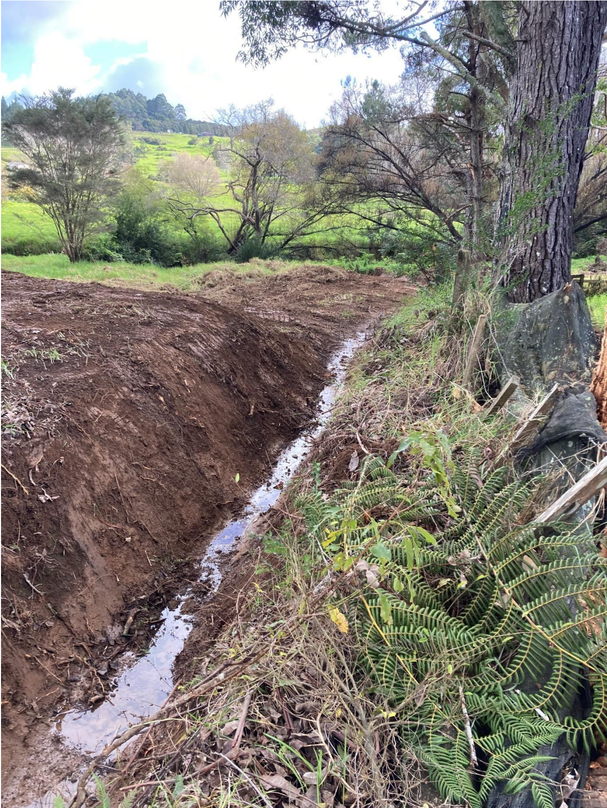
Figure 8: Oruru Rd 2 Rehab Additional Drainage Works
