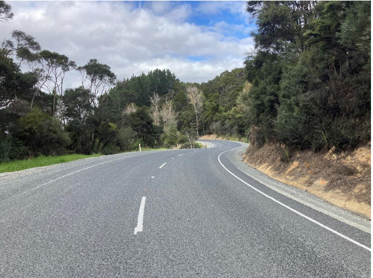
Figure 7: Kohukohu Rd Rehab Seal Complete
