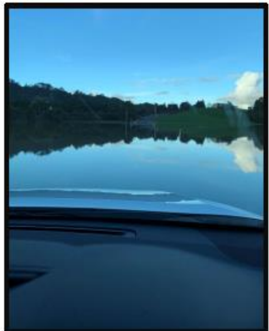
Matawaia-Maromaku Rd - Flooding
