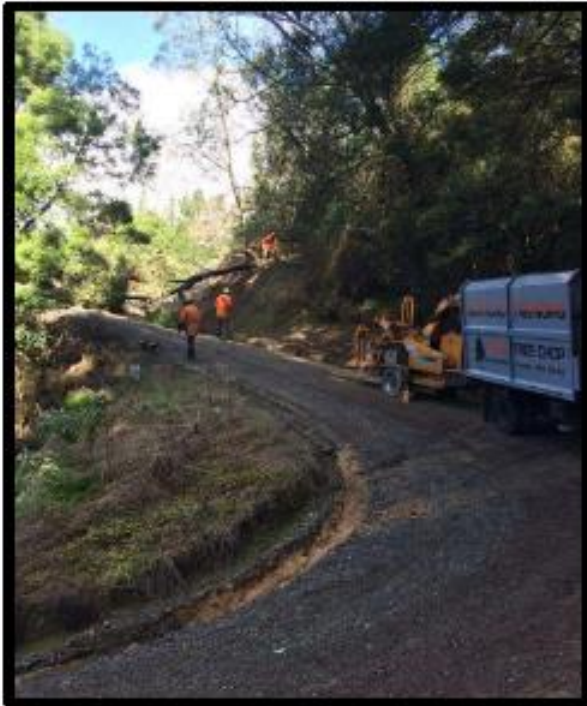
Tirohanga Rd – Tree Clearing
