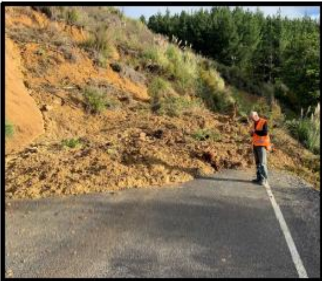
Pipiwai Rd – Major Slip
