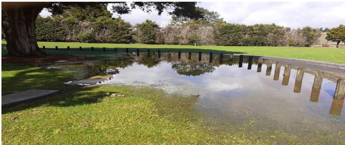
Picture showing surface water at the Kaikohe Cemetery
