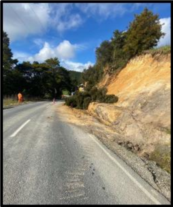
Ngapipito Rd – Slip Clearing
