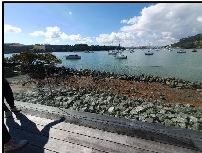
Figure 8: Image from the deck overlooking the Mangonui Harbour. Area of rocks is within the CMA, which was the portion of land identified as CMA when the title for the subject site was created in 2016.
