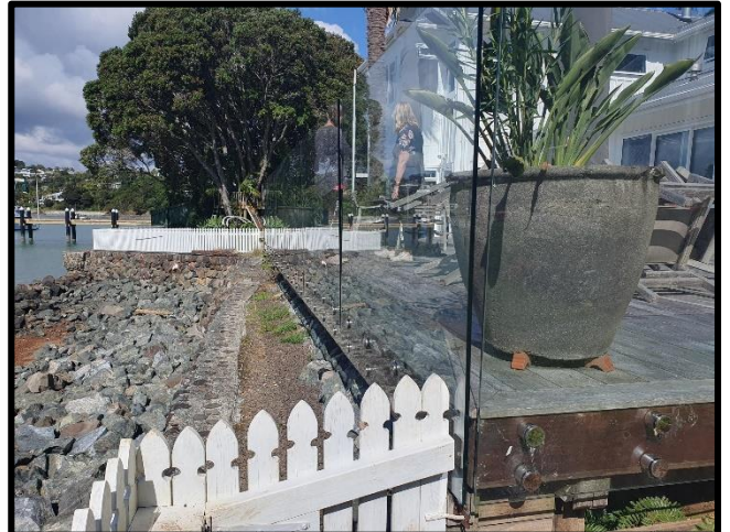
Figure 7: Existing glass balustrade which will be retained to form part of the pool fencing. Existing seawall within CMA.
