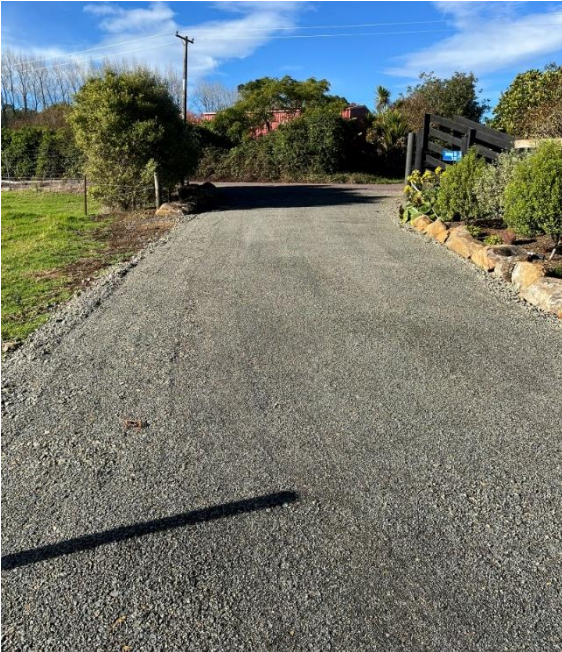
Photograph 3: Metalled Carriageway within ROW A – view south towards Waikuku Road.
