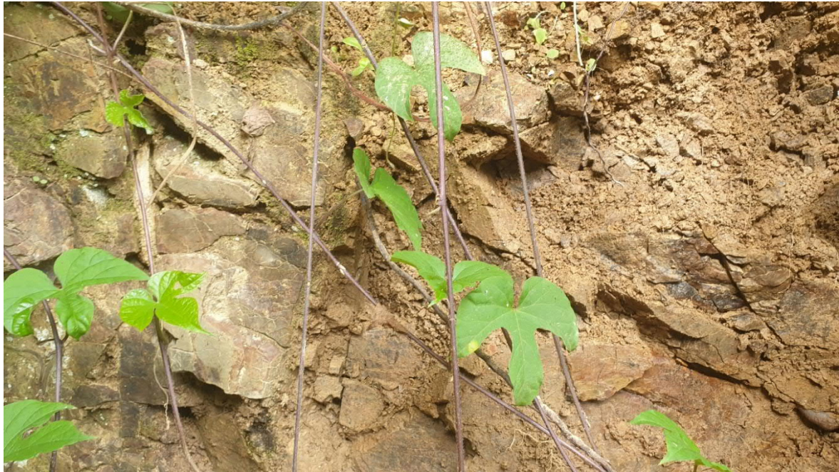
Photo 4 – Moderately to slightly weathered greywacke rock visible in a cutting in the centre of the site at the slope base.
