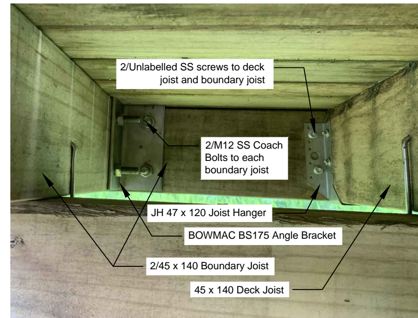
G 03 BOUNDARY JOIST CORNER CONNECTIONS SCALE(A3) NTS
