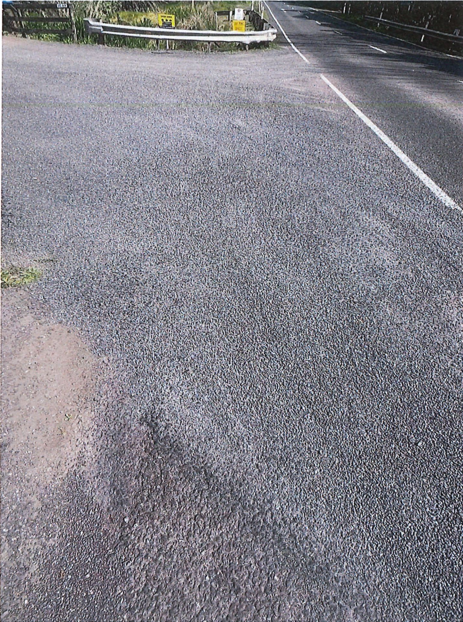
Closer view of seal.
