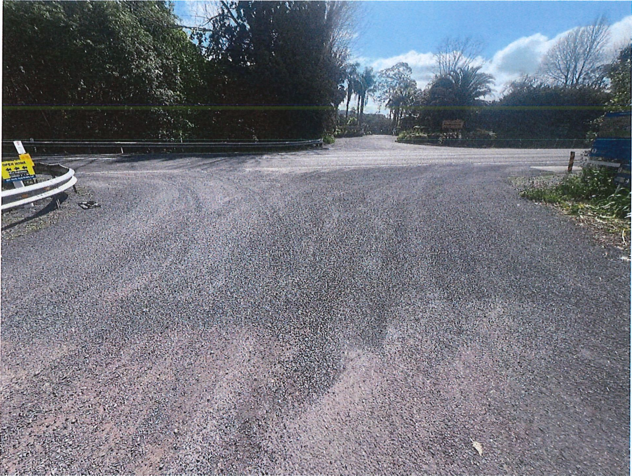
View from inside property boundary showing where new seal ends.
