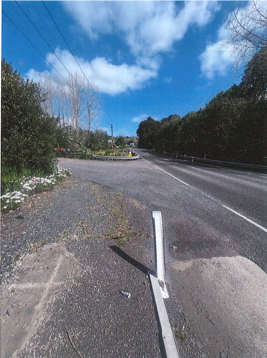
Chip sealed to boundary as per conditions.
