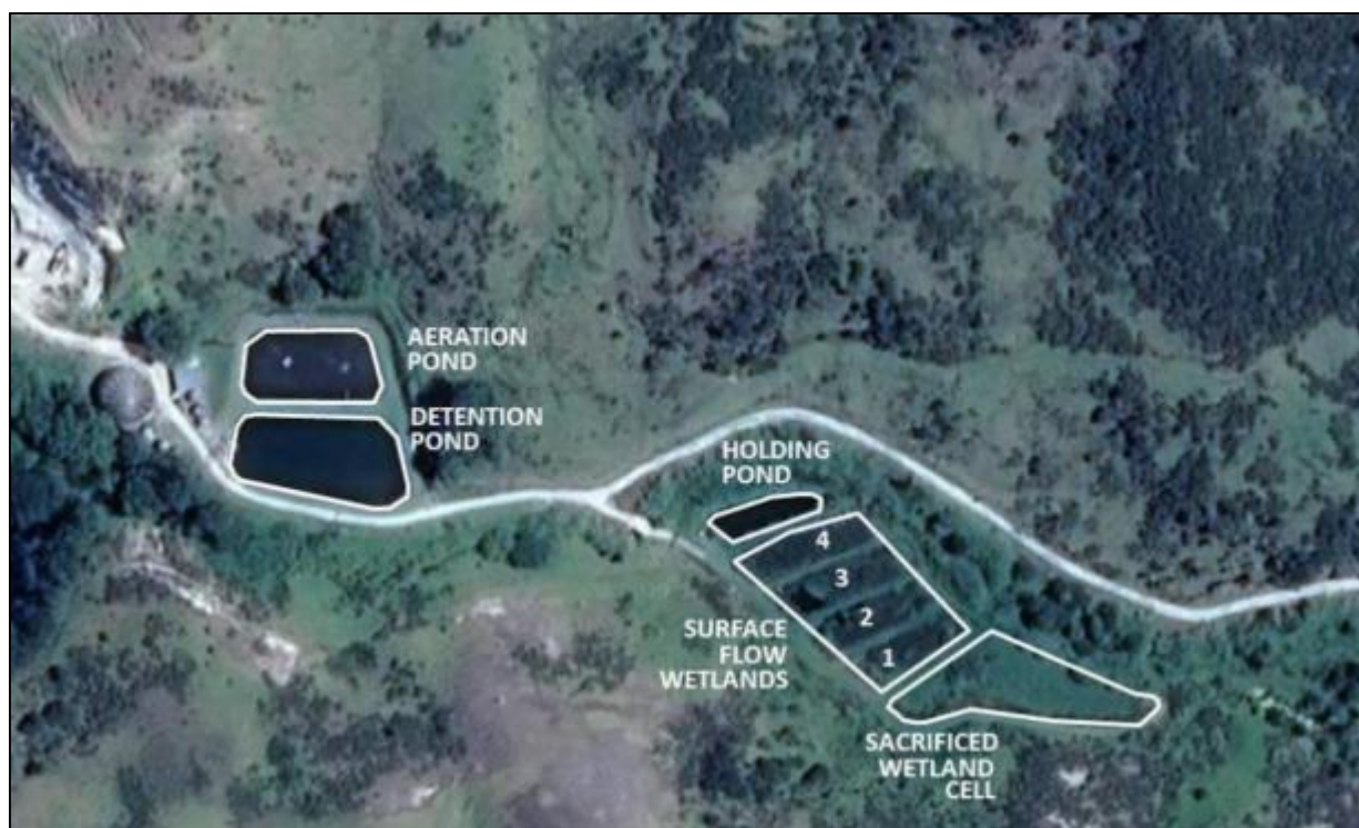
Figure 3-1: Aerial Photograph of Opononi WWTP
