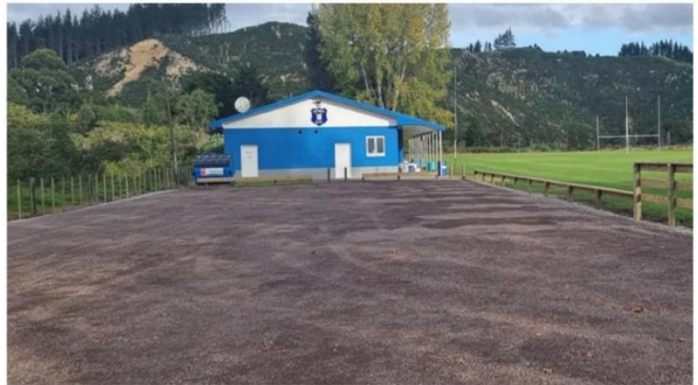
Before and after - shows external refurbishment of club, repaired boundary fence, upgraded entrance and carpark
