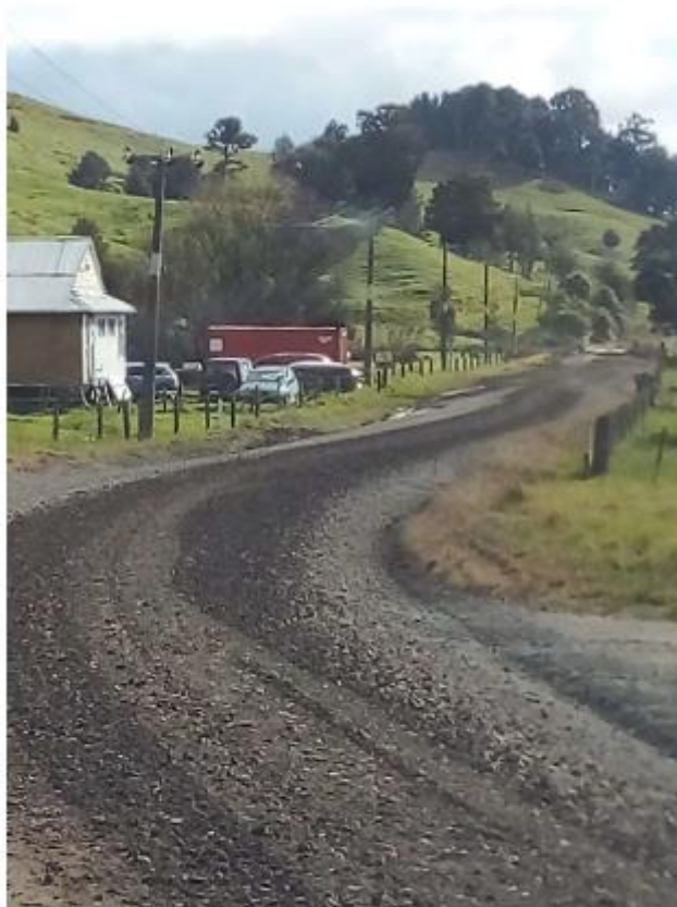
Orakau Rd – Maintenance Metalling
