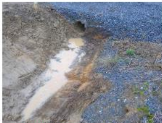
McIntyres Rd – Culvert Clearing
