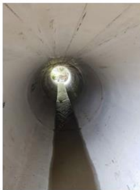
Wallis Rd – Large diameter Culvert installed
