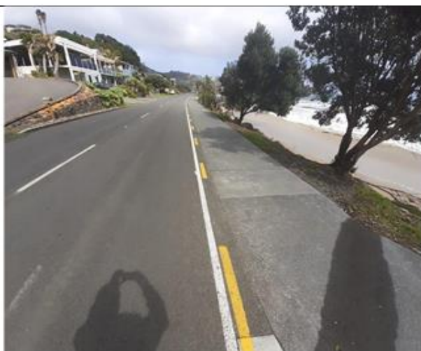
Ahipara Foreshore Road/Footpath being built on rehabbed seawall
