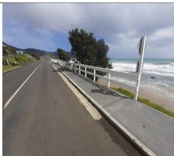
Ahipara Foreshore Road/Footpath being built on rehabbed seawall
