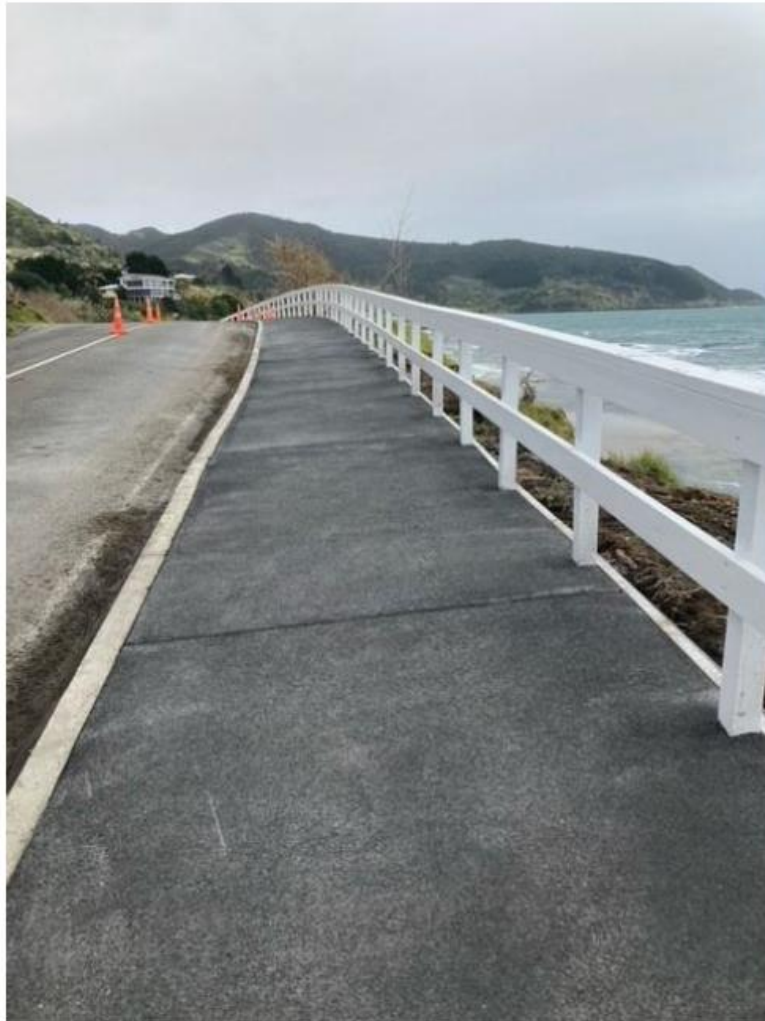
Figure 5: Foreshore Rd Footpath completed above rock wall.
