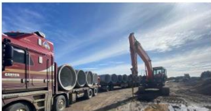
Peras Rd/Wahamati Rd – Culverts being delivered
