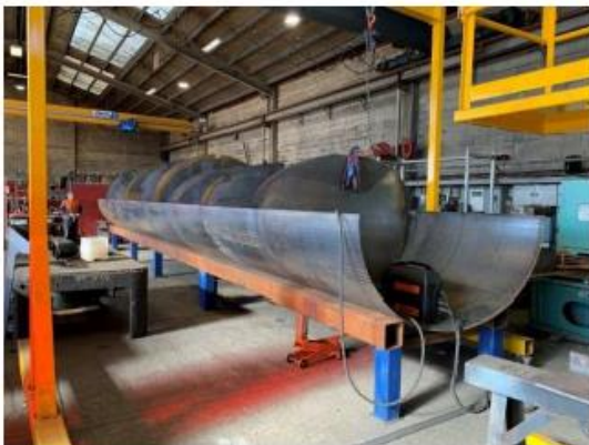
Fabrication of the new bitumen bulk tanker
