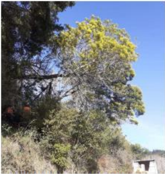
Tapuhi Rd – Emergency Works – Dangerous Tree
