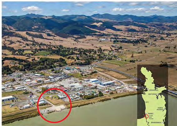
Kopu Boat Ramp, Off Quay Street, Kopu
