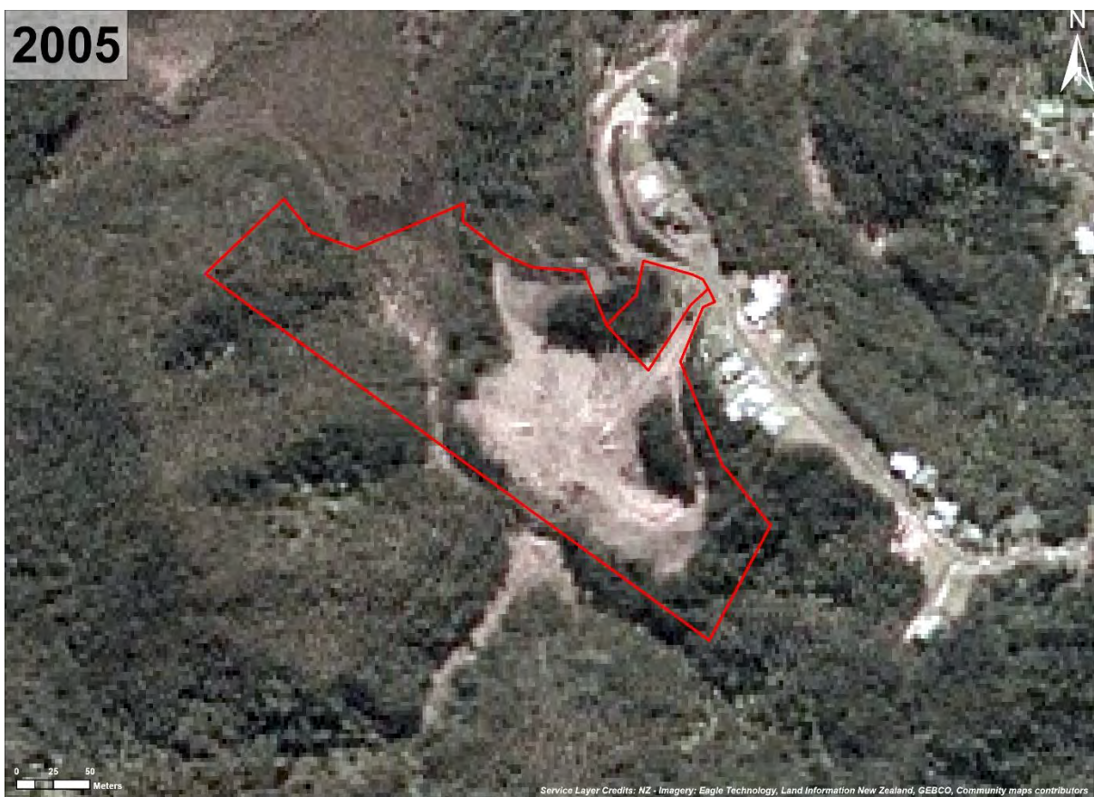
Figure 6: Showing the site and surrounds in 2005 (Source: LINZ)
