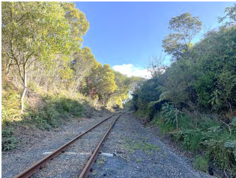
Figure 3: Edge and exotic vegetation within the project footprint.
