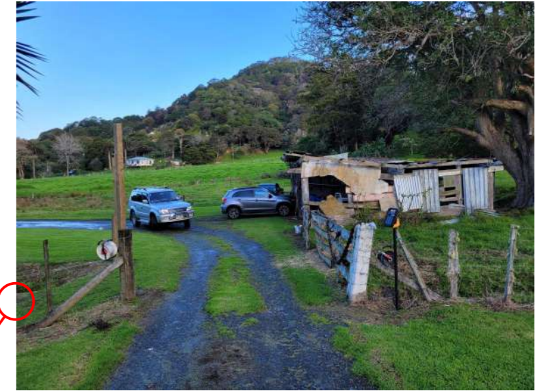
OLD UTILITY SHED - VIEW FROM HOUSE
