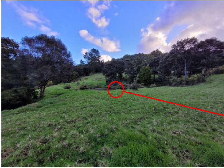
EXISTING IRRIGATION DAM
