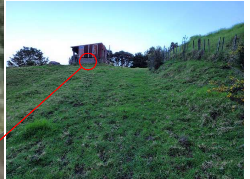
OLD COW SHED AND ACCESSWAY UP FROM ROAD
