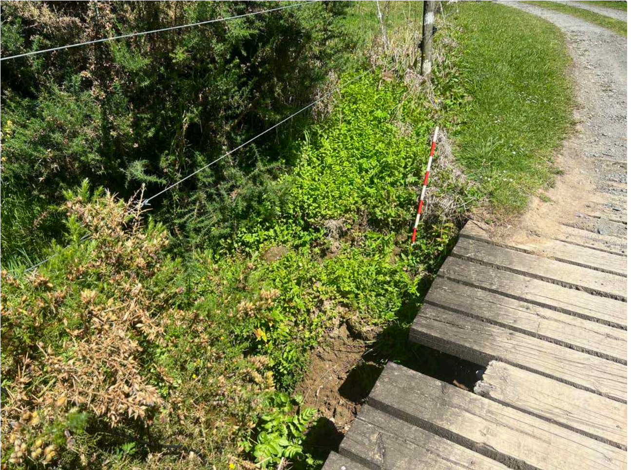
Figure 11. View adjacent to proposed bridge replacement
