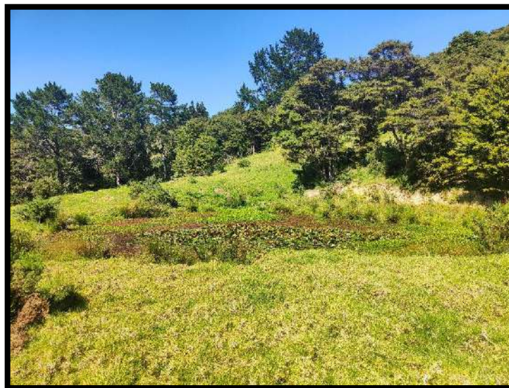
Figure 6 – Constructed irrigation dam on the upper block
