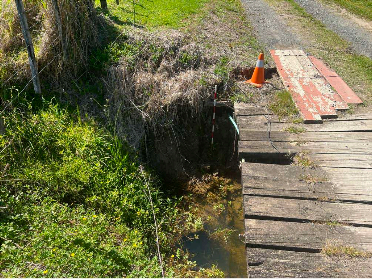
Figure 12. View adjacent to proposed bridge replacement
