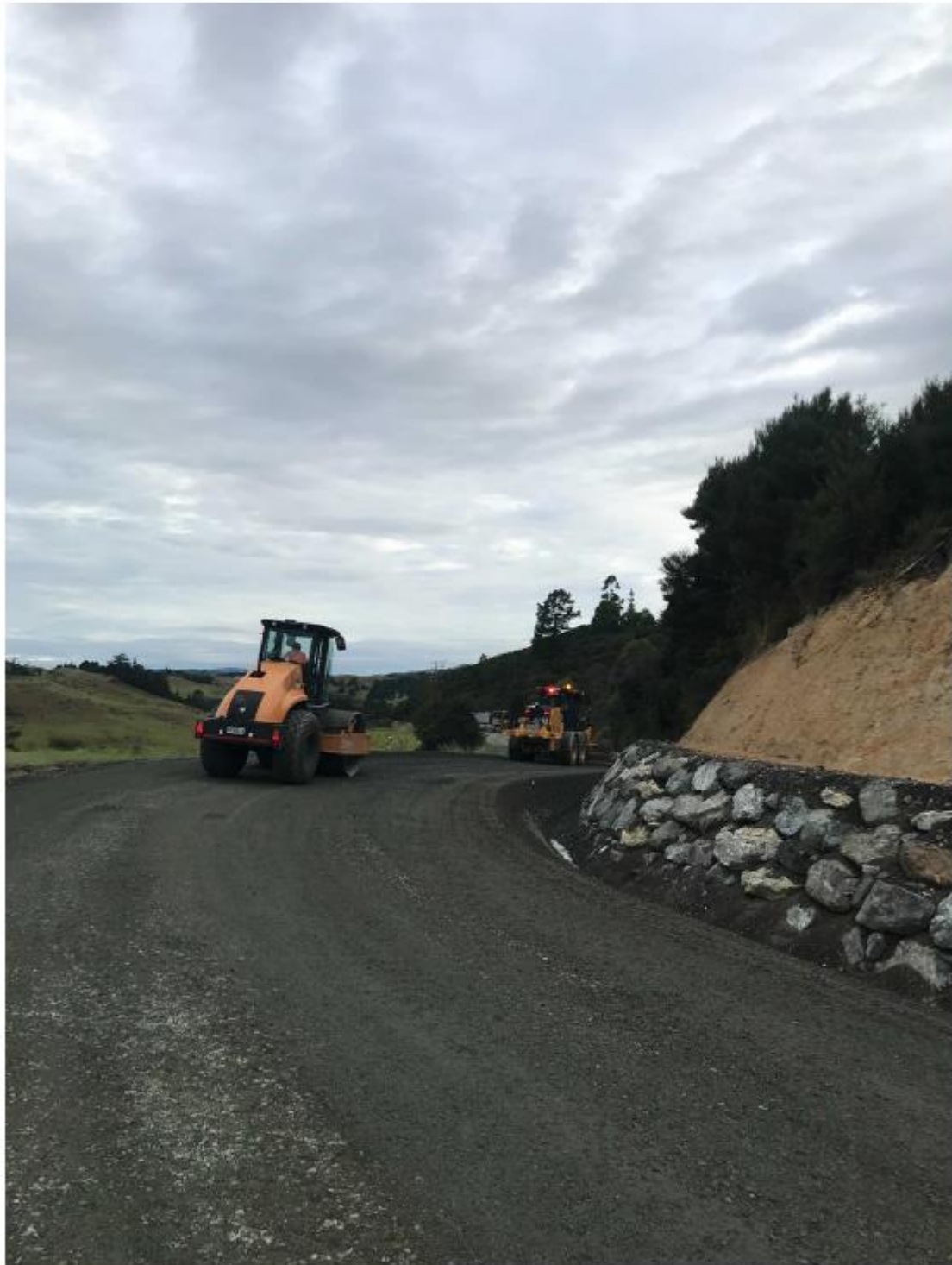
Figure 10: Overlay in progress in Section Three
