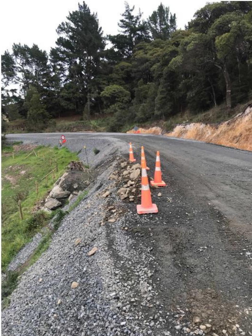
Figure 8: Rock wall construction in Section Three
