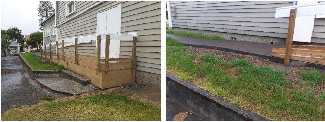
Rawene Hall Accessibility Ramp
