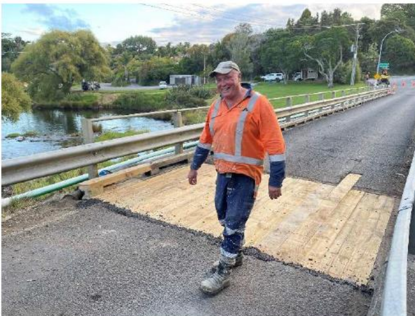
Landing Rd Bridge – Deck replacement with chipsealing booked for early March
