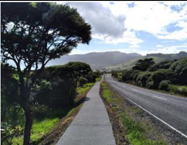
Signal Station Road/ Completed Footpath
