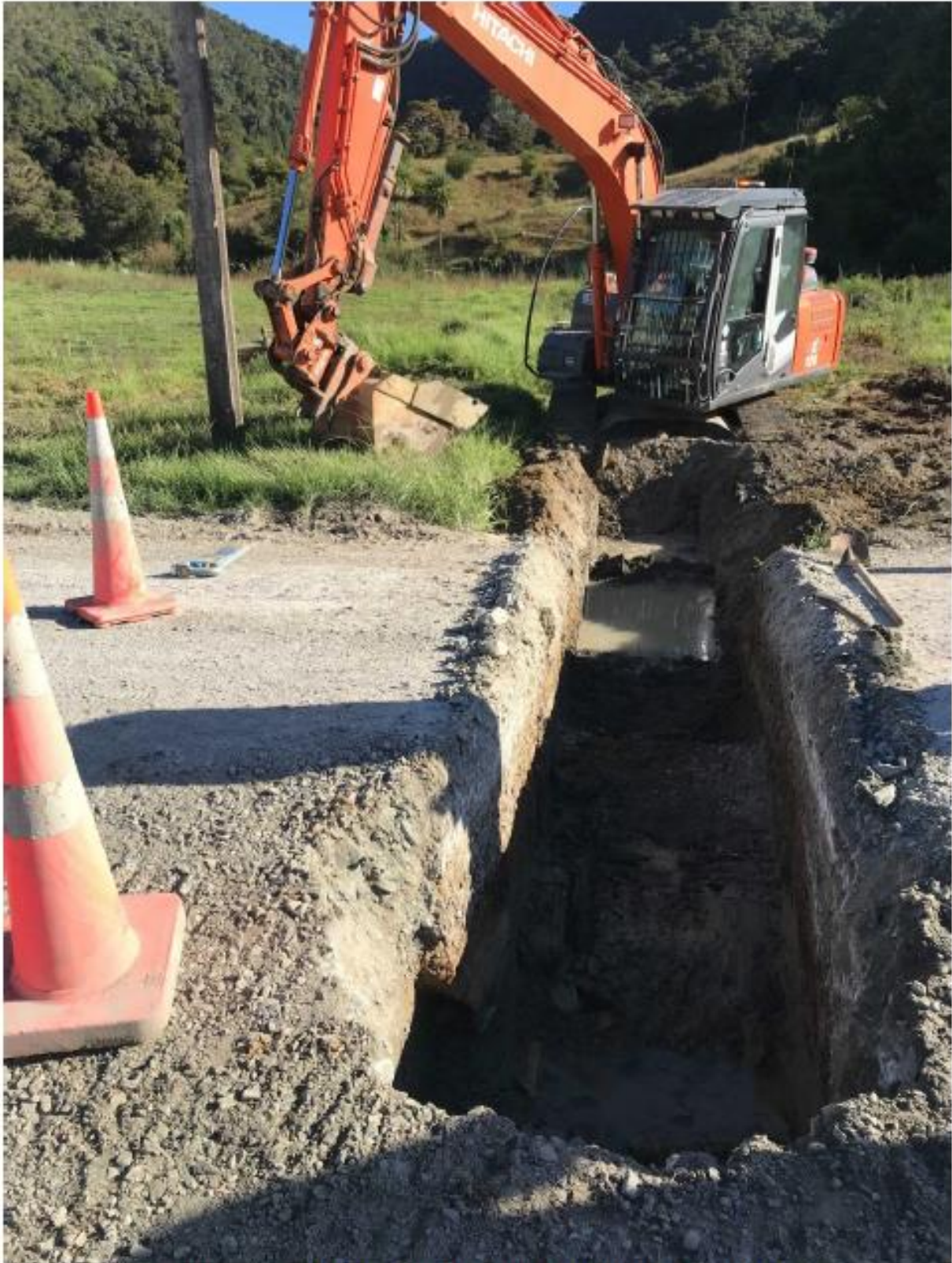
Figure 7: Section 4 culvert replacements in progress
