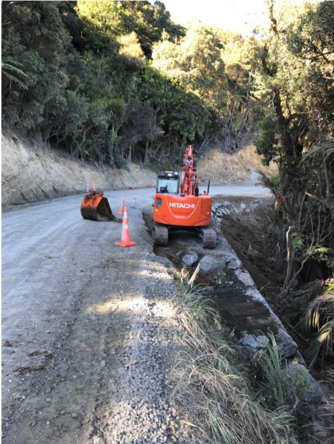
Figure 8: Section 4 Rock wall construction in progress
