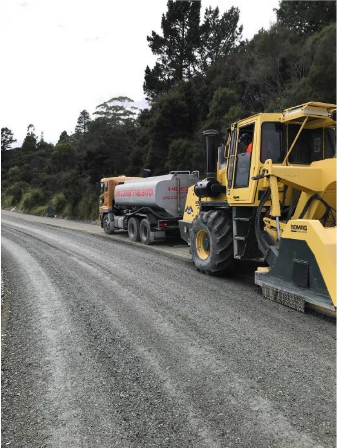
Figure 13: Section Three Stabilising in progress
