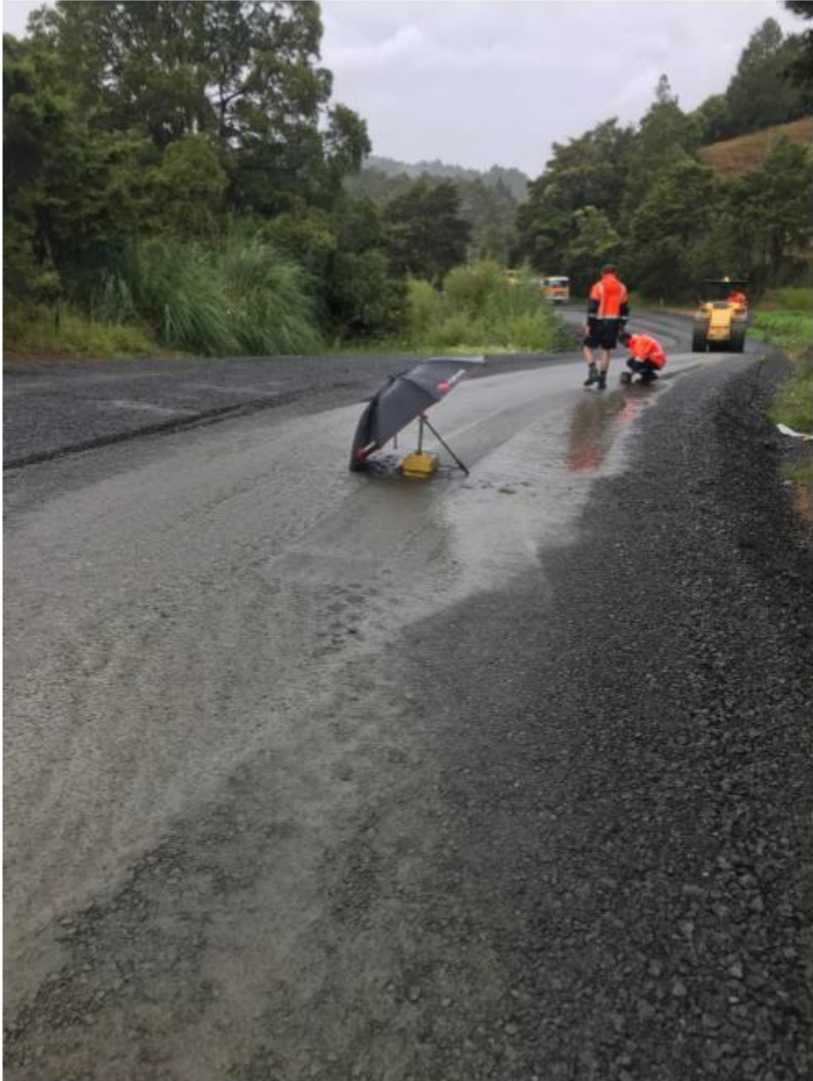
Figure 2: Nuke testing on stabilised section
