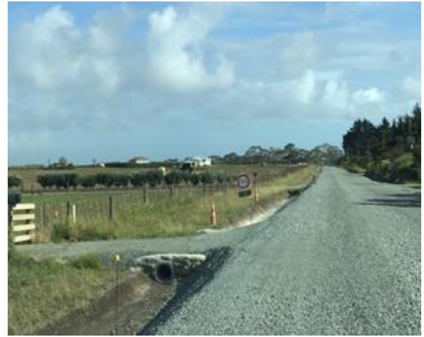
Church Road, Kaitia Seal Extension/Culvert installation and overlay progress
