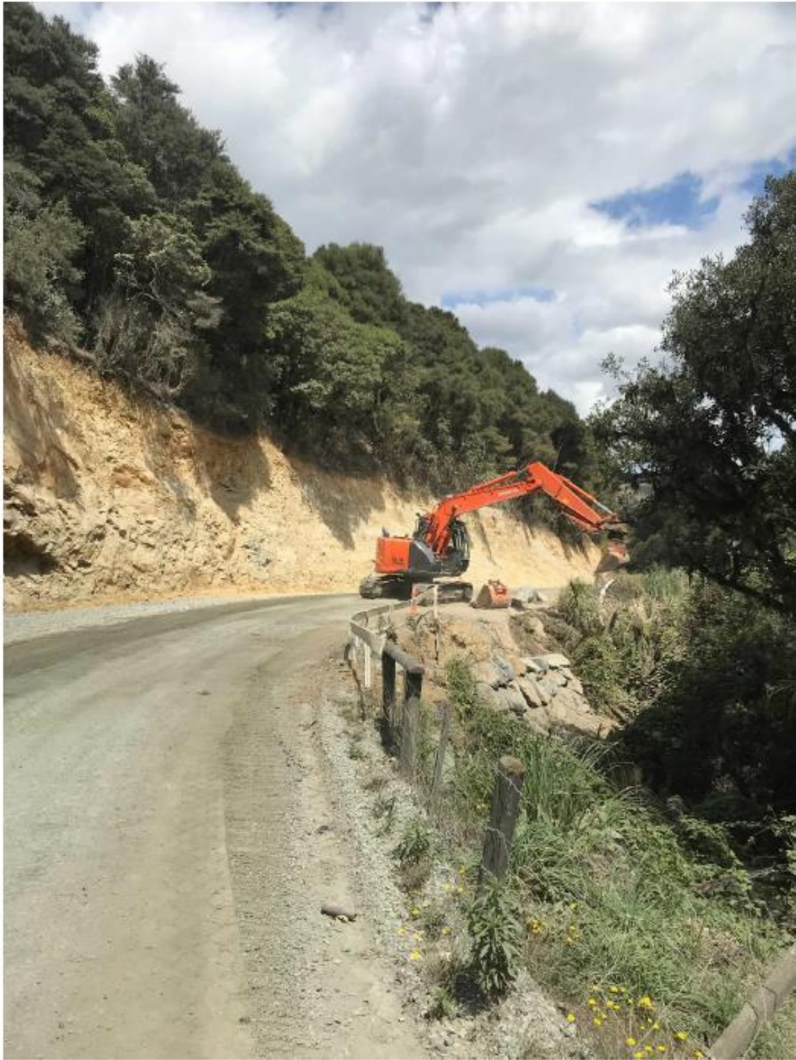
Figure 4: Rock wall construction in Section Four
