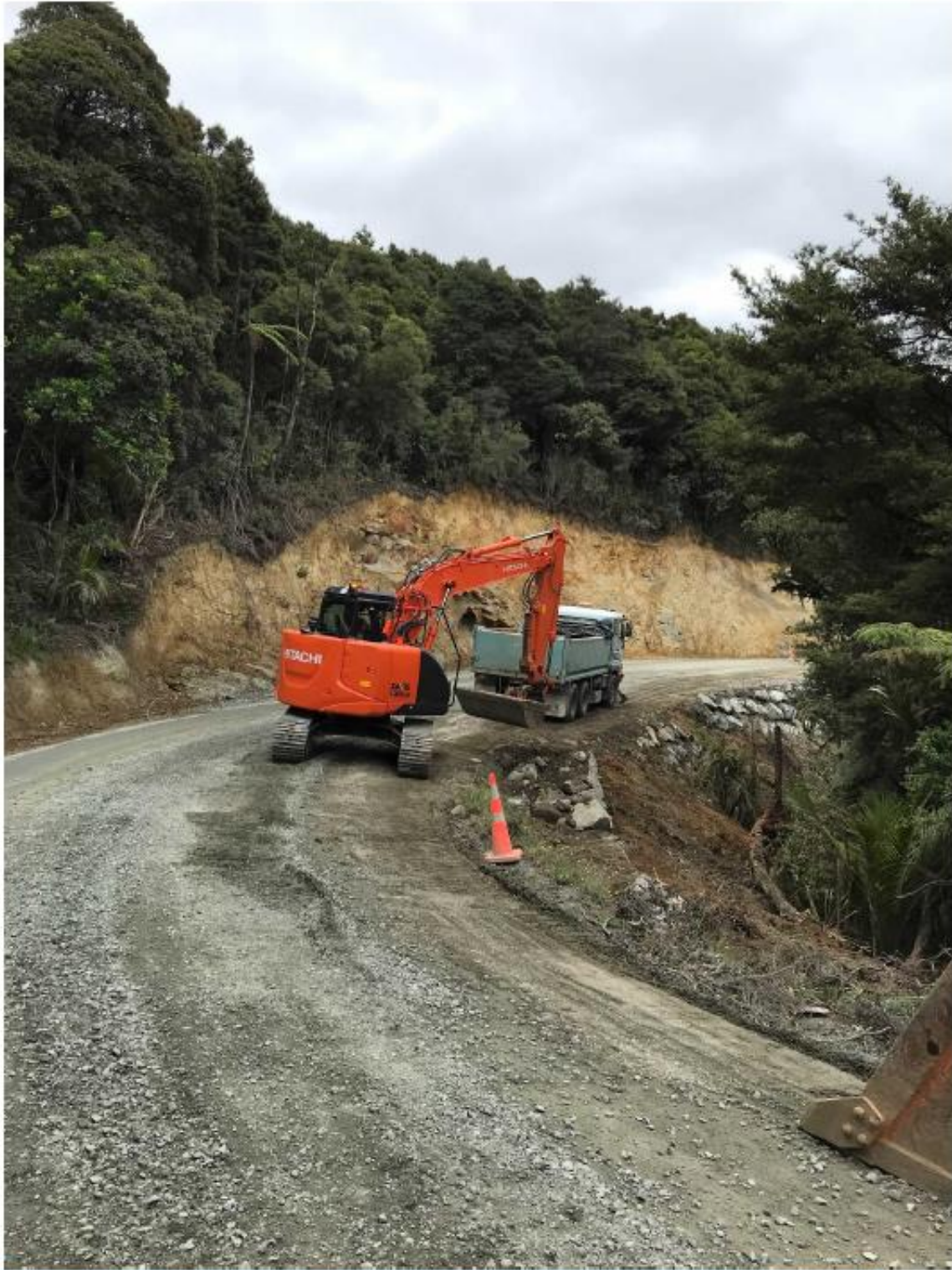
Figure 3: Rock wall Construction in Section Four
