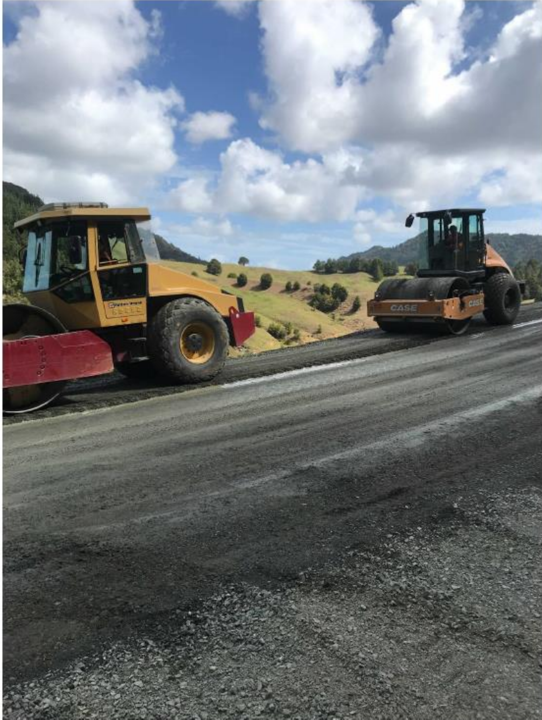
Figure 5: Section Three stabilising in progress
