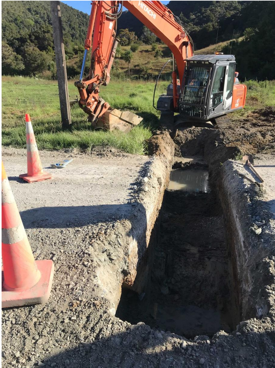
Replacement of culvert in Section 4.
