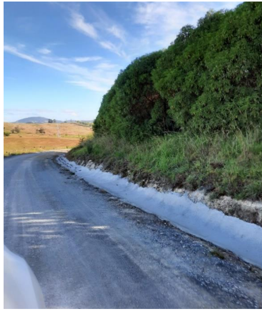
Jobe Rd – concrete lined channel
