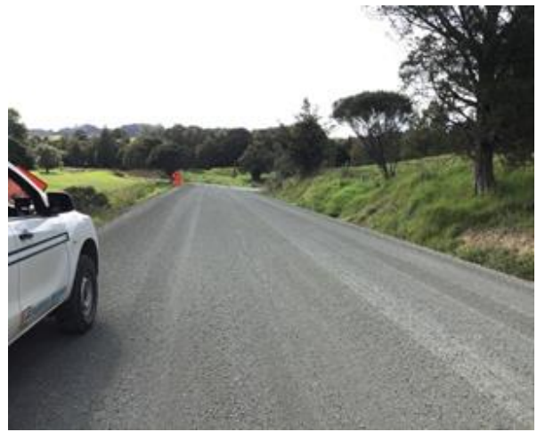
Pawarenga Rehab / Prepared pavement surface (ready for seal) with running coarse
