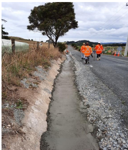
Schoemaker Rd - concrete lined channel
