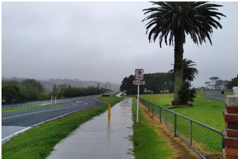
The Beginning Location of the shared path section
