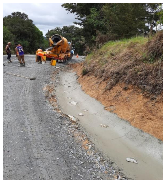
Helmsdale Rd - concrete lined channel
