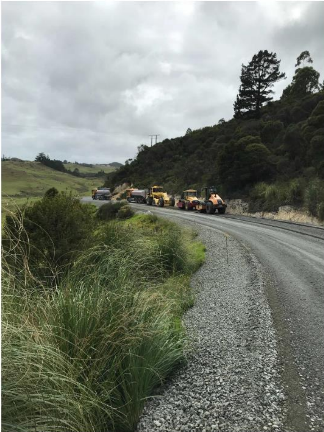
Figure 12: Section Three Stabilising in progress
