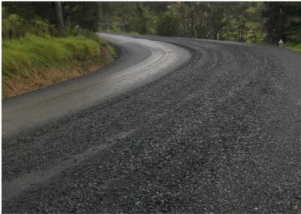
Figure 1: LHS stabilisation in progress
