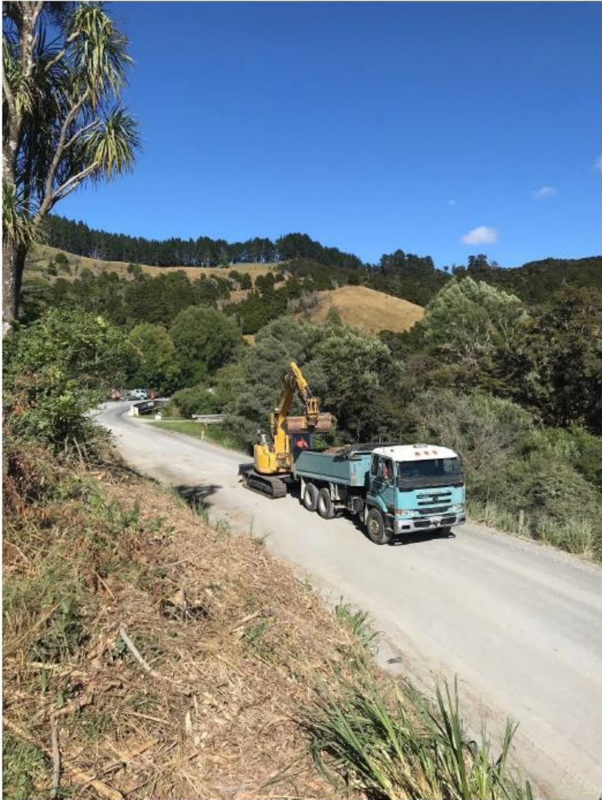
Figure 2: Clearing in progress Section Five
