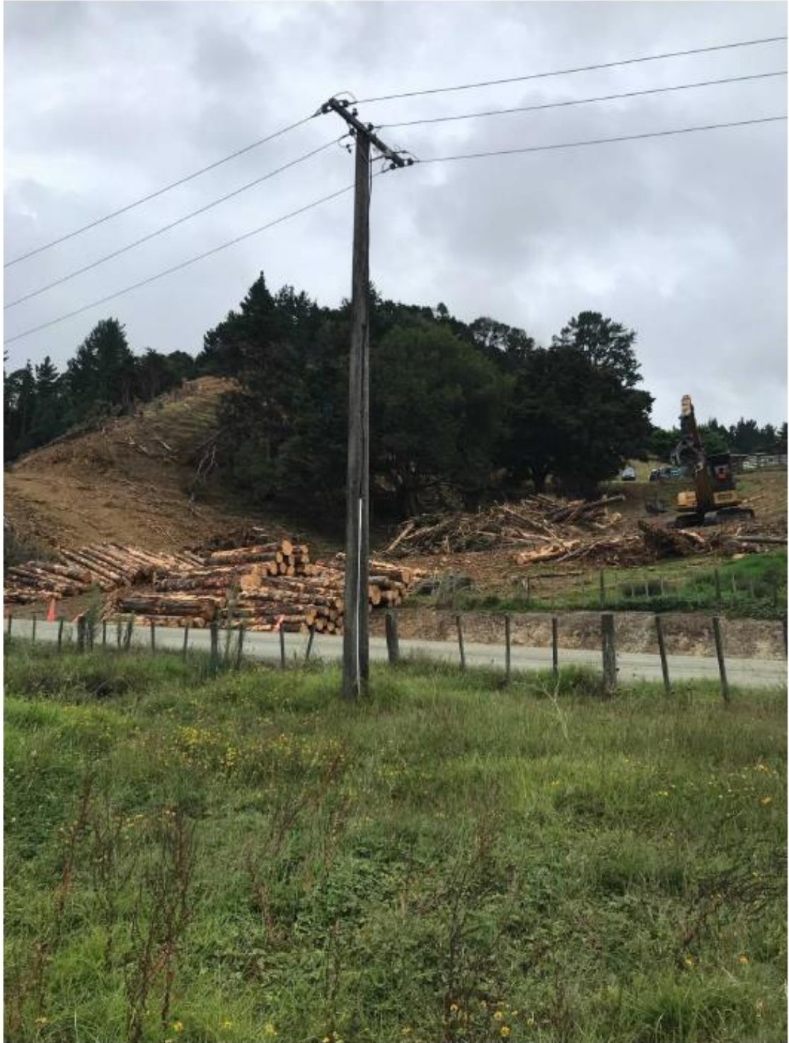
Figure 7: Tree removal in Section Four
