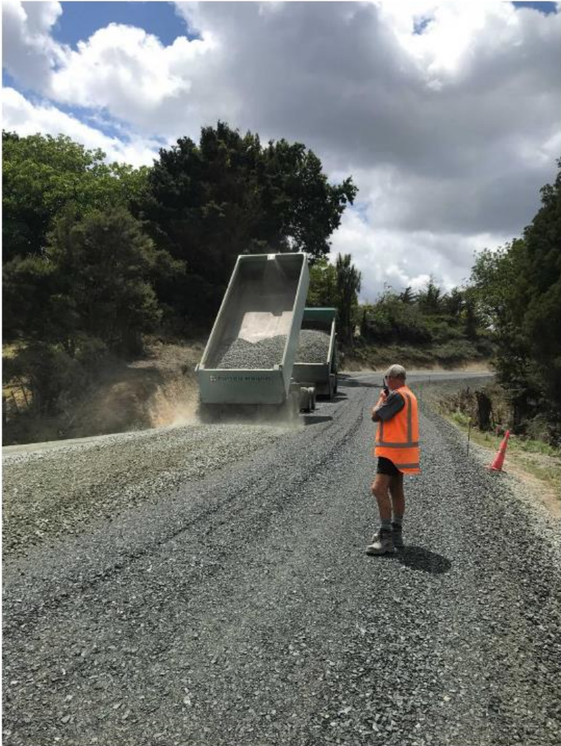
Figure 5: Overlay in progress Section Three
