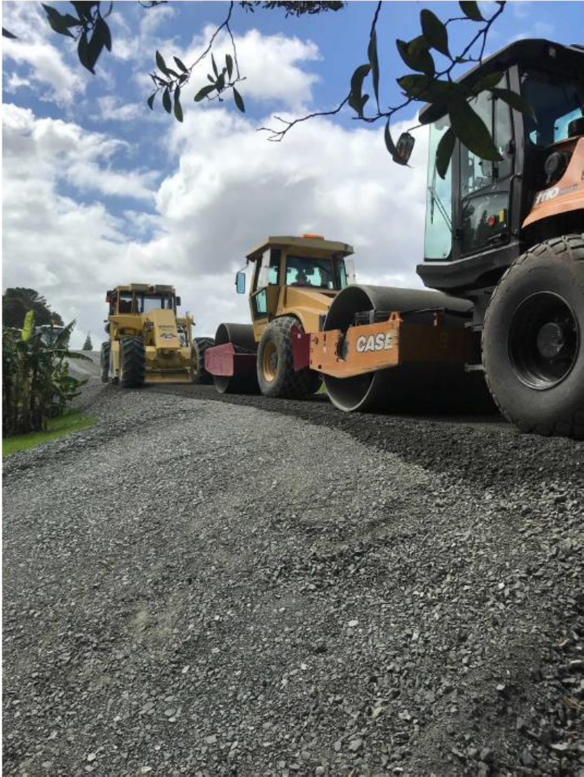
Figure 6: Section Three stabilising in progress
