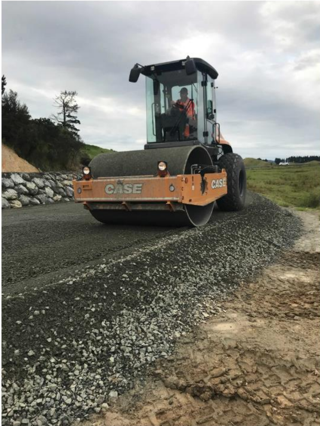
Figure 11: Overlay in progress in Section Three
