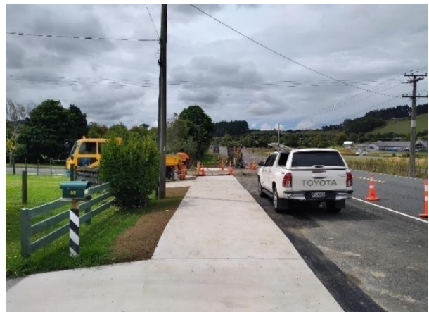
Final culvert installation and Shared Path section (W=2.5m)
