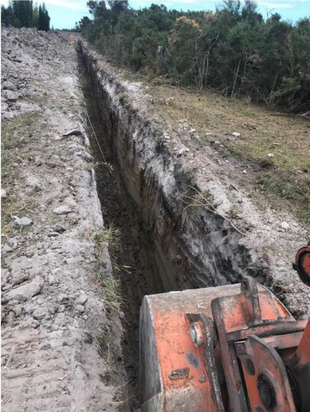
Figure 1: Drainage through private property in progress
