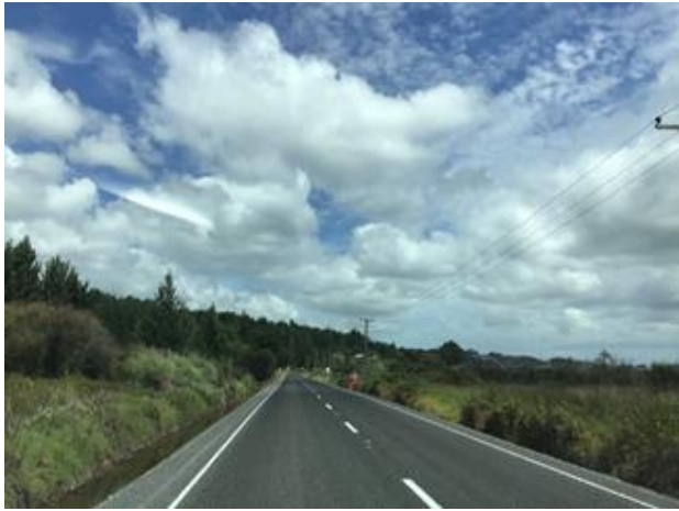
Horeke Road Rehab/Completed Seal Surfacing
