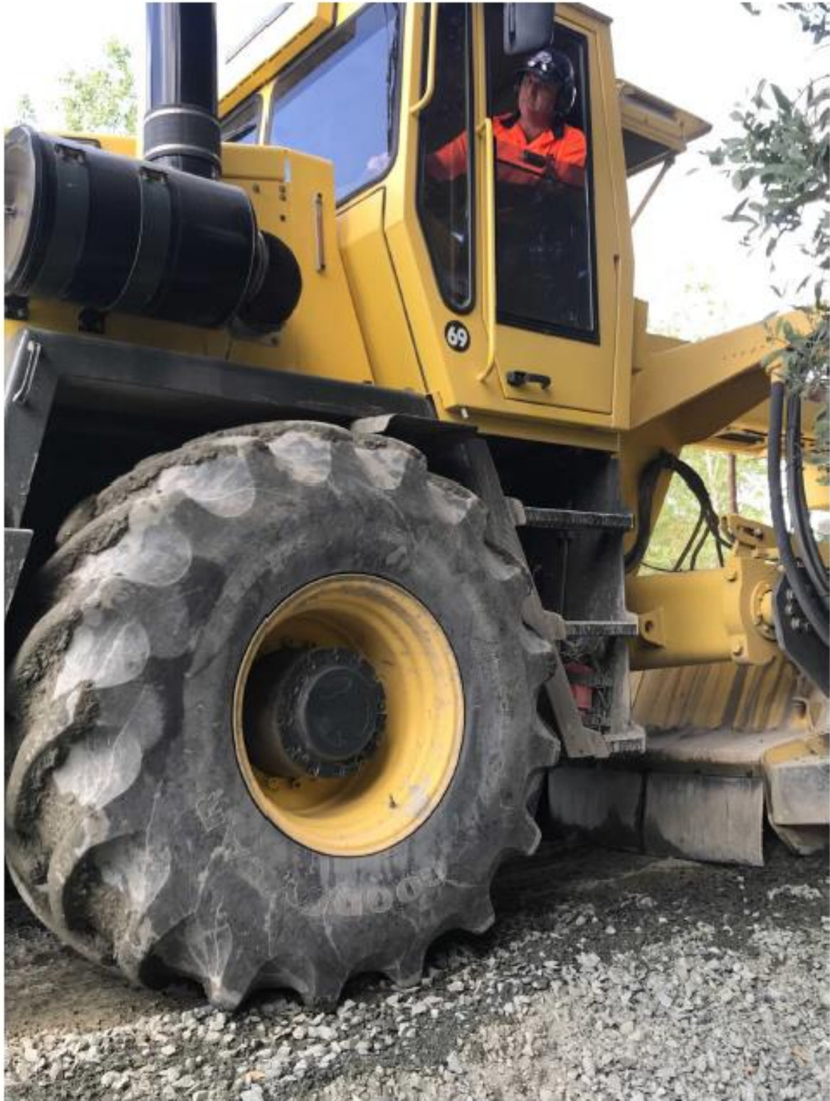
Figure 4: Section Three stabilising in progress
