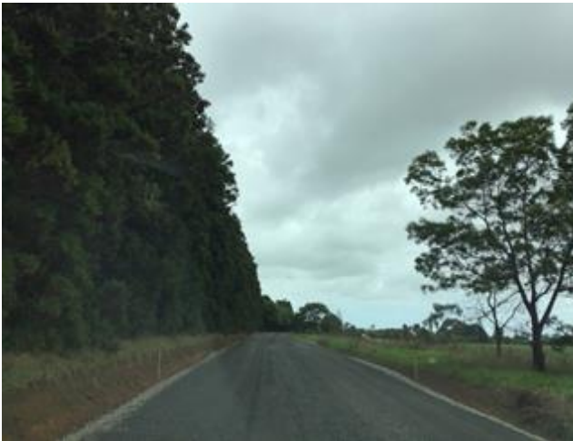
Koropewa Road, Waipapa Seal Extension / Sub-base overlay progress
