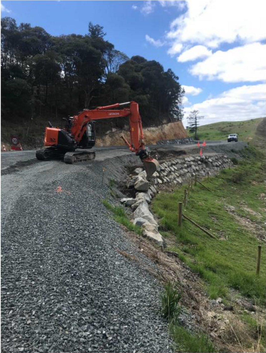
Figure 9: Rock wall construction in Section Three
