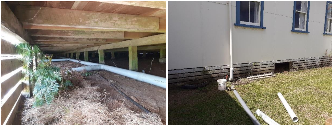
Okaihau Hall Stormwater Renewal Works
