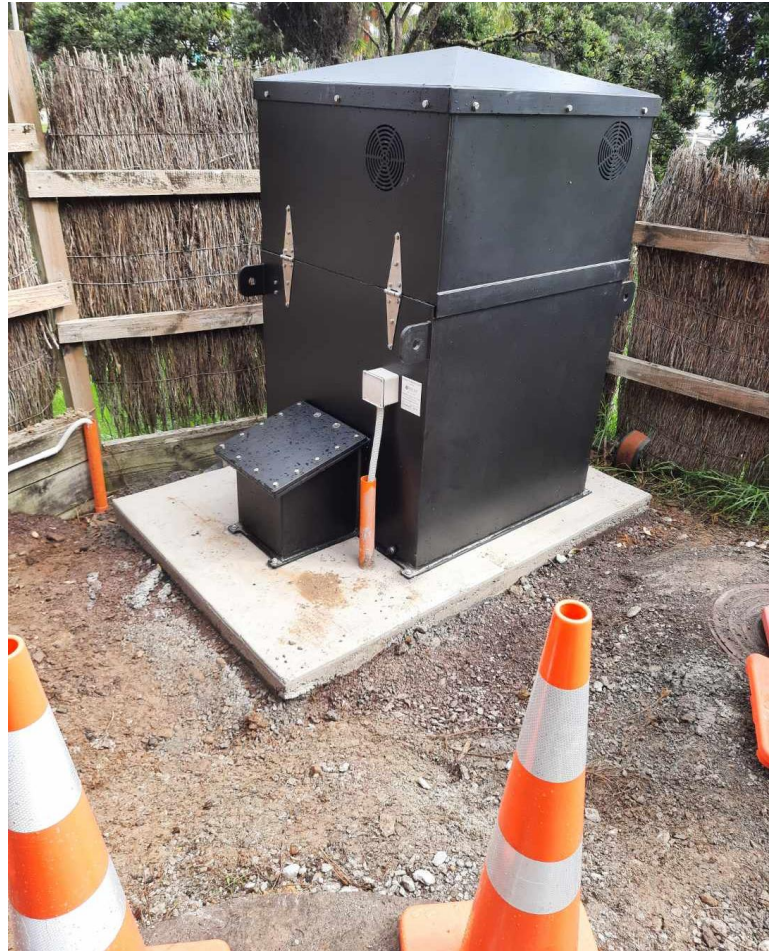
1Mill Road Odour Unit Install - Mangonui
