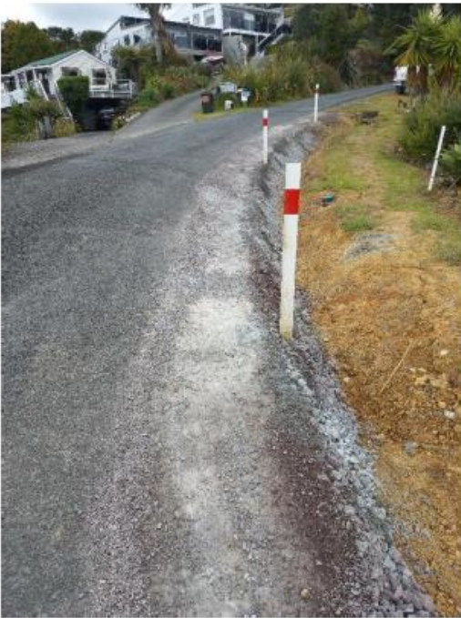
School Rd, Paihia - Washed out shoulder repairs
