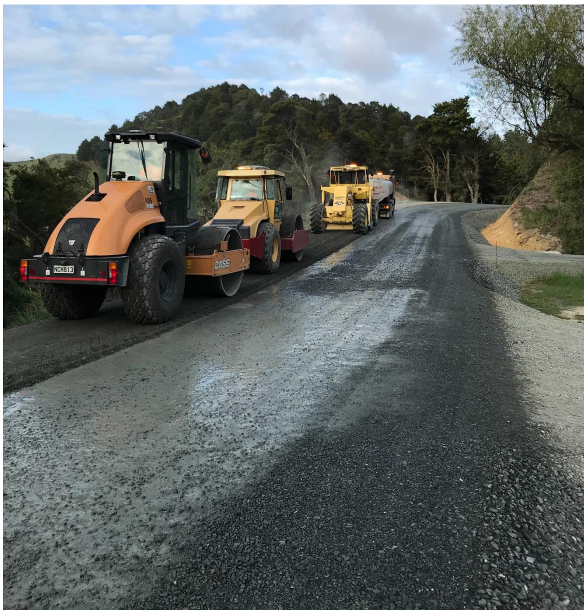
Stabilising in progress at Peria on Section 3
