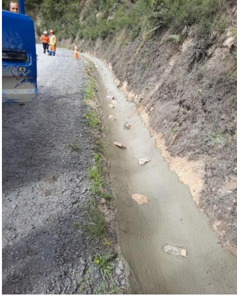
Waipu Caves Rd – concrete lined channel
