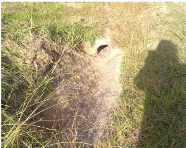
Harrison Rd – Routine Culvert Clearing
