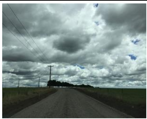
Pungaere Road, Waipapa Seal Extension/Pavement overlay progress section 1
