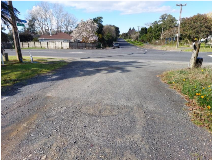
Existing crossing, with Riverview Road opposite.
