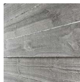
G. CONCRETE SHUTTER
