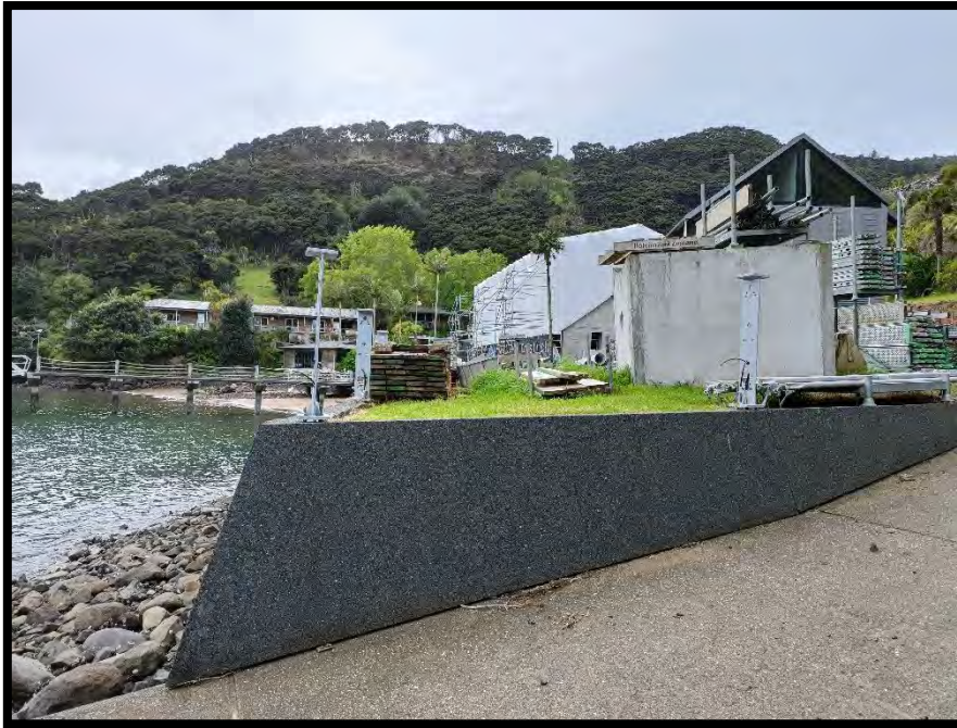
Figure 2 – Main lodge and boat shed currently under redevelopment
