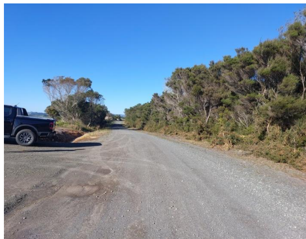
Tahanga Road with extra width crossing to serve Lots 4 & 5 at left of picture
