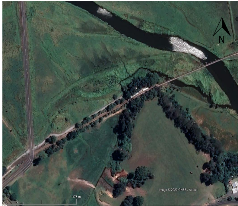
C 7 Aerial photograph taken in 2022. Contemporary use with train parked at station (Source: Google Earth)
