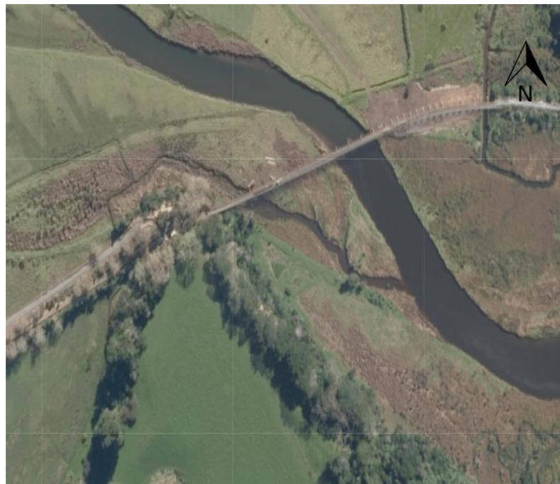
C 6 Aerial photograph taken in 2014-2016 showing bridge repair works (Source: LRIS)
