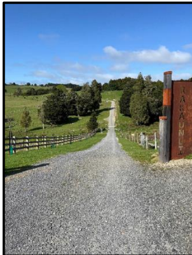
Figure 23: View of the existing access within Proposed Easement B, showing straight alignment and pullover bay. Image taken from the LDE report.
