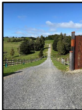
Figure 19: View of the access within Easement B showing straight alignment and ample sight distances. Image taken from LDE report.
