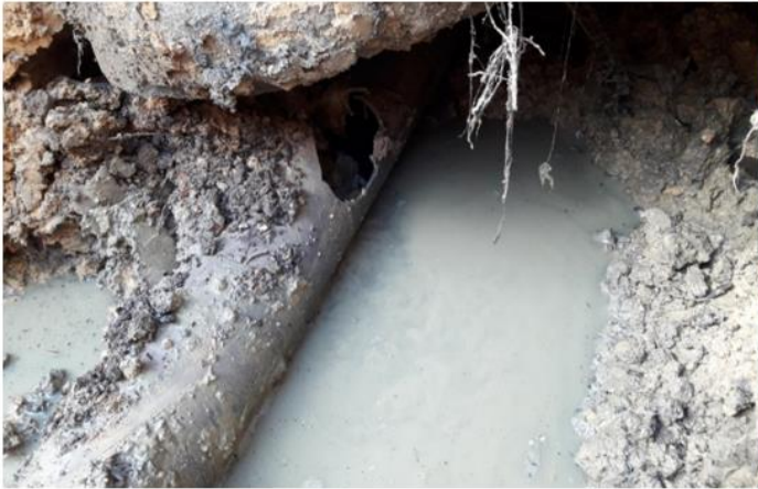
Cable Bay 100mm Sewer line repair.
