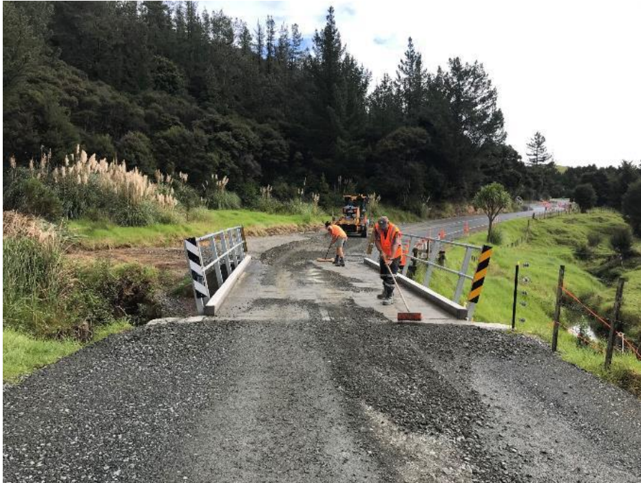
Figure 5: Peria Road Bridge Approaches
