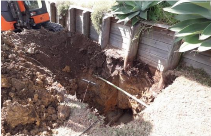
Cable Bay 100mm Sewer line repair.
