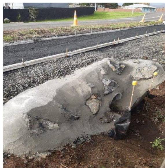
Kotare Street Culvert Extension & Headwall
