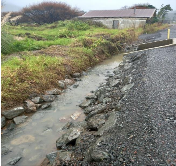
Panguru improvement / Scour Protection Work
