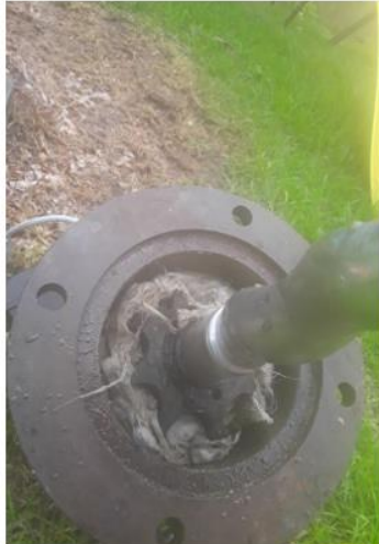
Ragged and blocked LPS Pump.
