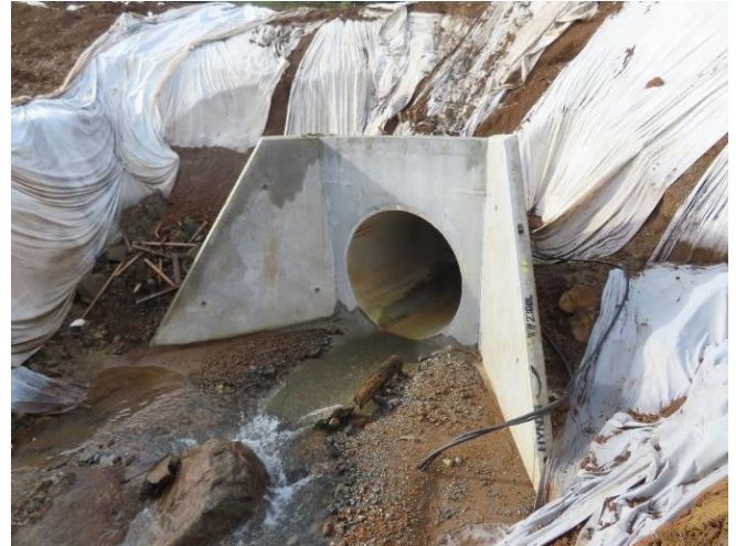
Headwall inlet to 2100mm diameter culvert
