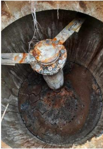
Sewer line Air Release Valves
