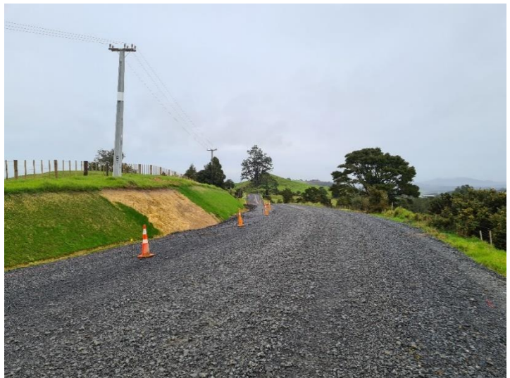
New pole installed and stay wire removed.
