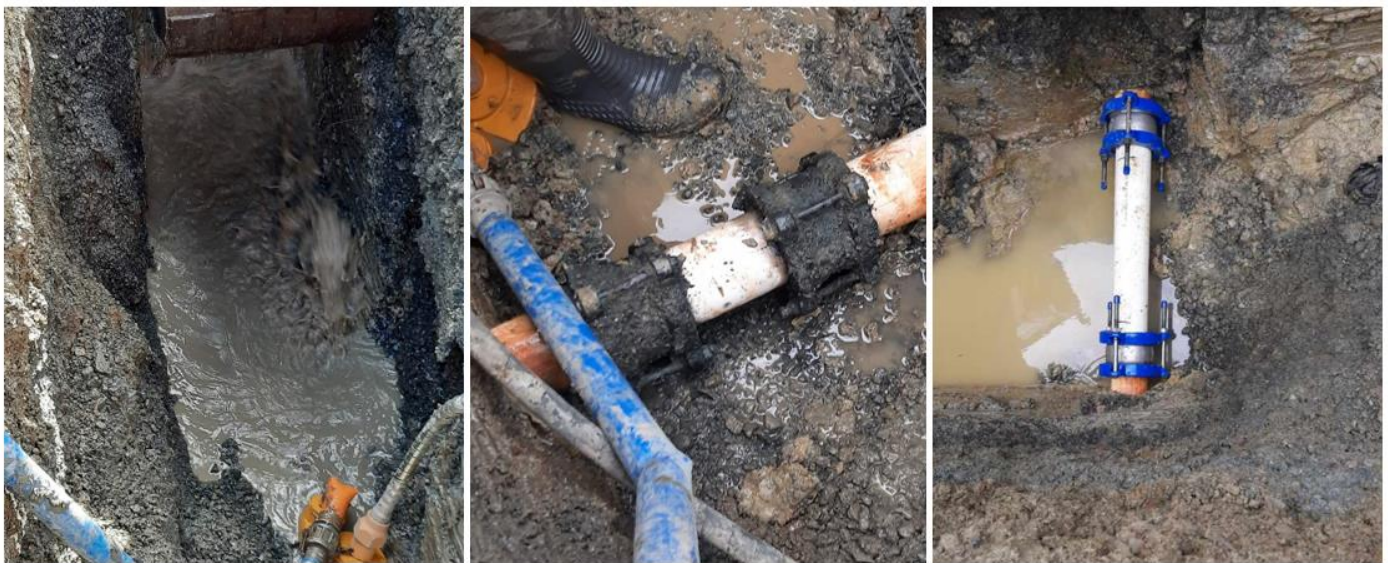
North Road, Kaitiaia. Water break and repair.
