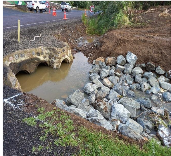
Panguru improvement works / Construction of Rock Weir Structure
