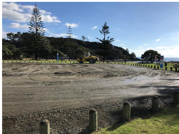
Figure 4: Cable Bay Carpark Upgrade
