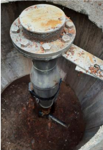
Sewer line Air Release Valves
