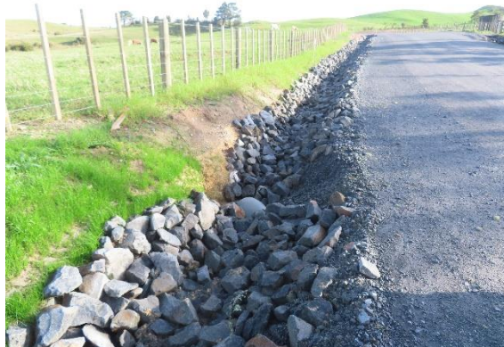
Rock lining roadside drains
