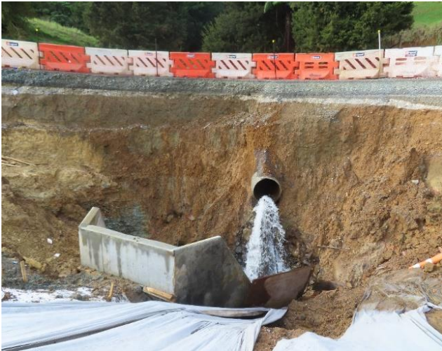
Existing culvert outlet and new headwall to 2100mm diameter culvert
