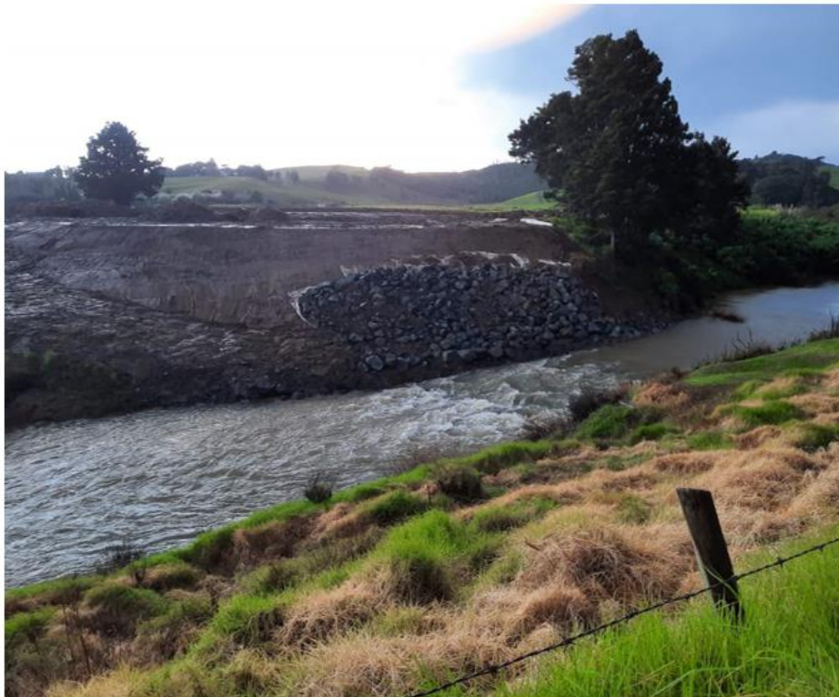
Awanui Intake Stabilization Work
