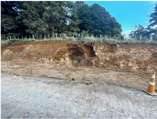
Above photos showing an embankment cavity after a large rock has been removed and new rocks uncovered and placed safely out of the works carriageway whilst proposed locations are determined.
