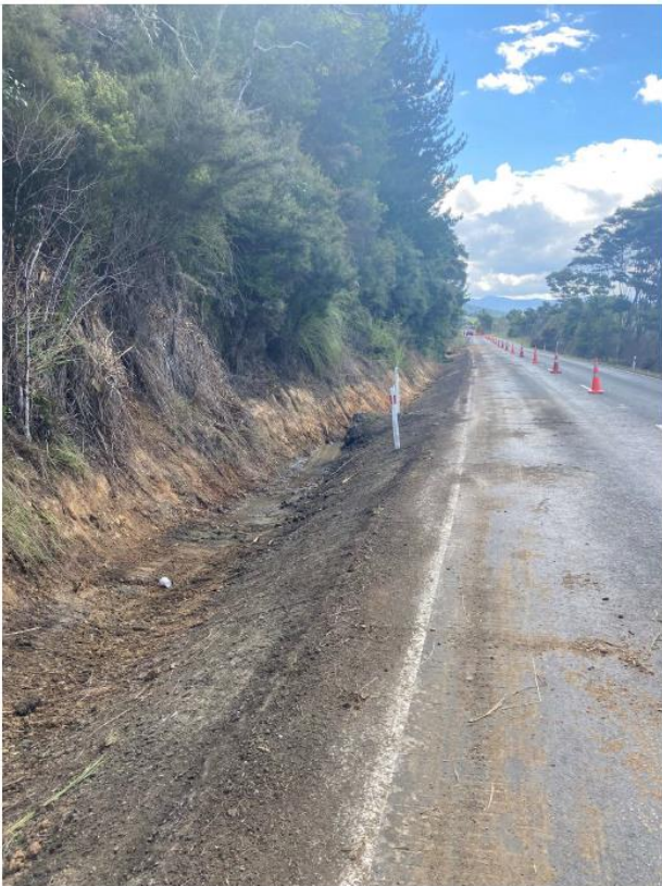
Figure 14: Kohukohu Rd Rehabilitation Water tabling
