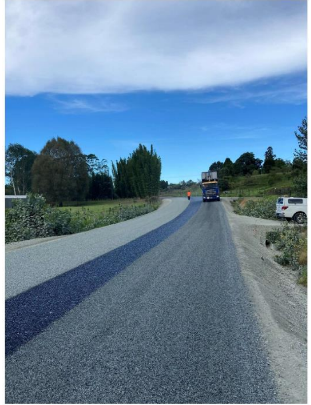
Figure 13: Oruru Rd Rehabilitation Site 2 Sealing
