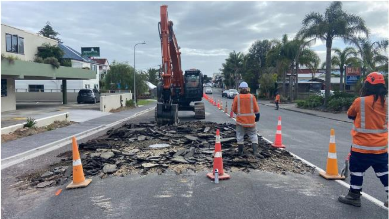
Kings Rd – First day breaking ground
