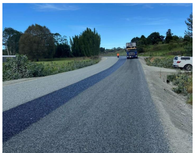
Oruru Rd Rehabilitation Site 2/ Sealing
