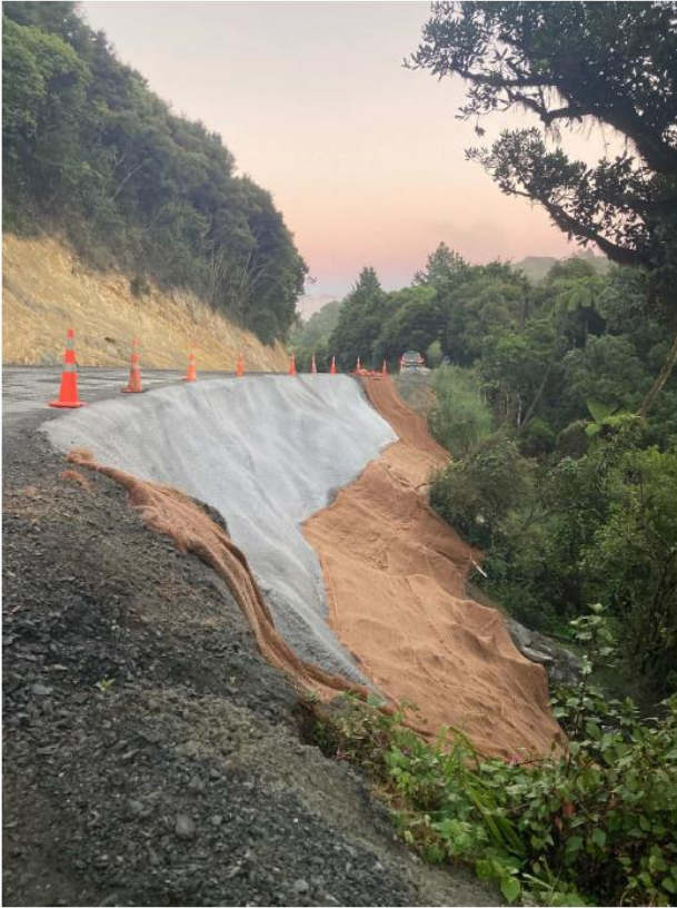
Figure 4: Peria Rd Seal Extension RP4100 Slip Repair
