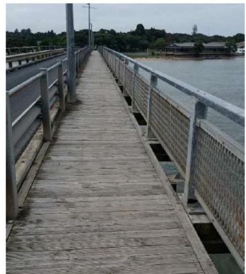
Waitangi Bridge (Footbridge)
