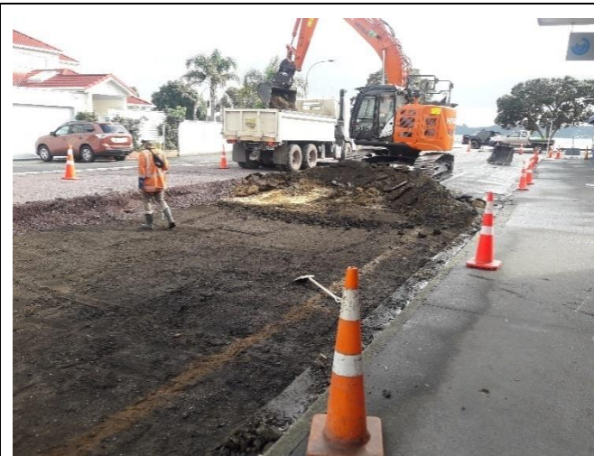
Kings road, Paihia/ Rehabilitation
