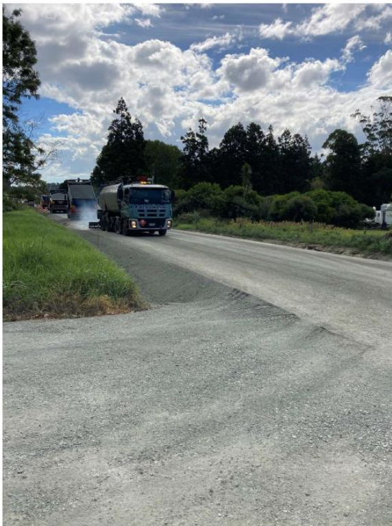
Figure 11: Oruru Rd Rehabilitation Site 2 Sealing
