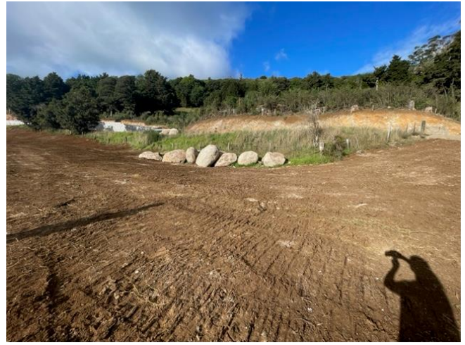
Above photos showing an embankment cavity after a large rock has been removed and new rocks uncovered and placed safely out of the works carriageway whilst proposed locations are determined.
