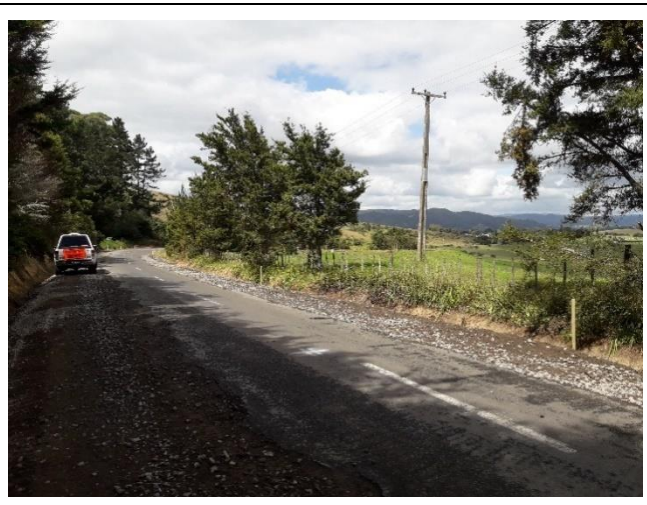
Waimatenui Mataraua Road/ Rehabilitation
