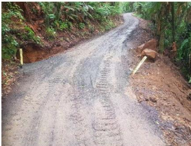
Wekaweka Rd – New culvert line after pic
