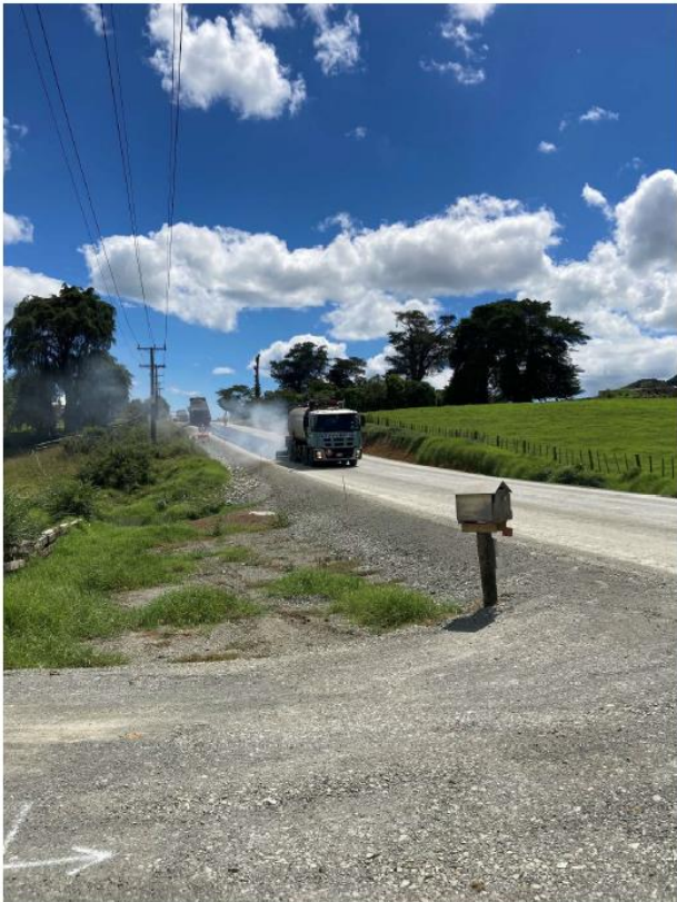
Figure 6: Oruru Rd Rehabilitation Site 1 Sealing
