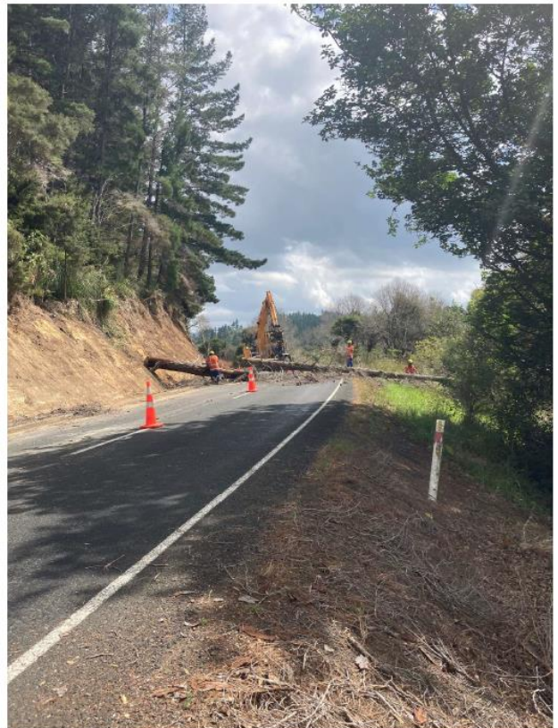
Figure 15: Kohukohu Rd Rehabilitation Tree Removal
