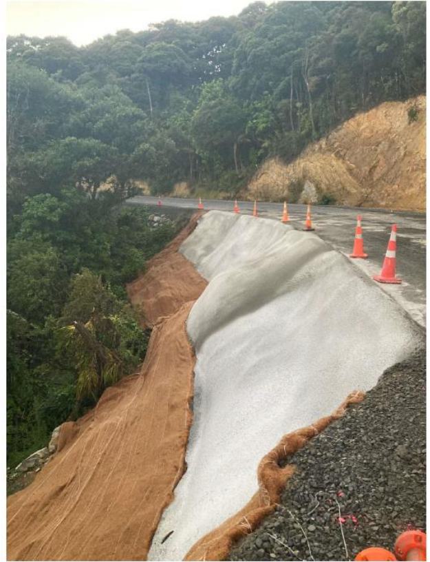
Figure 5: Peria Rd Seal Extension RP4100 Slip Repair
