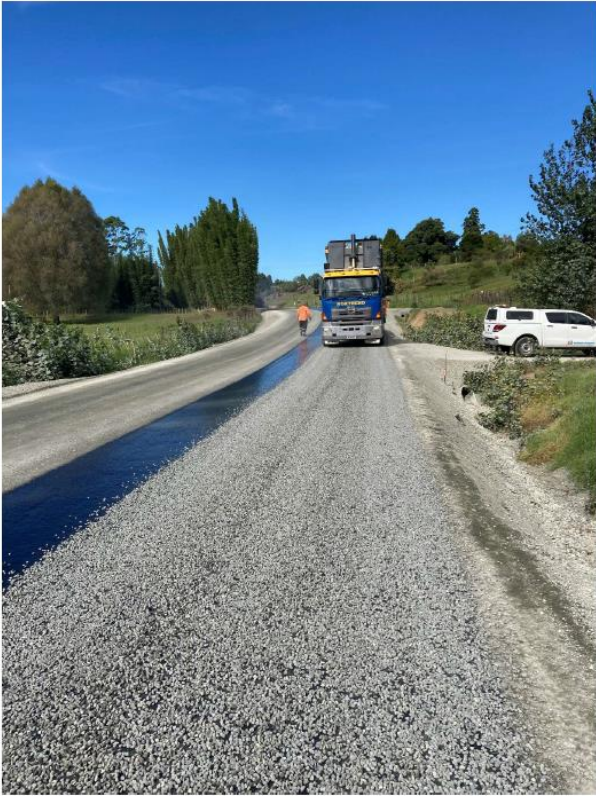
Figure 12: Oruru Rd Rehabilitation Site 2 Sealing
