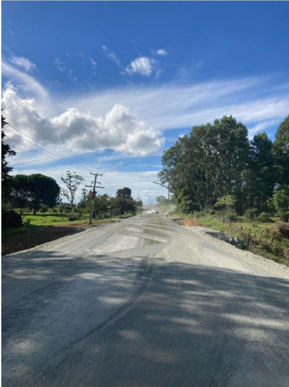
Figure 8: Oruru Rd Rehabilitation Site 1 Seal Preparation
