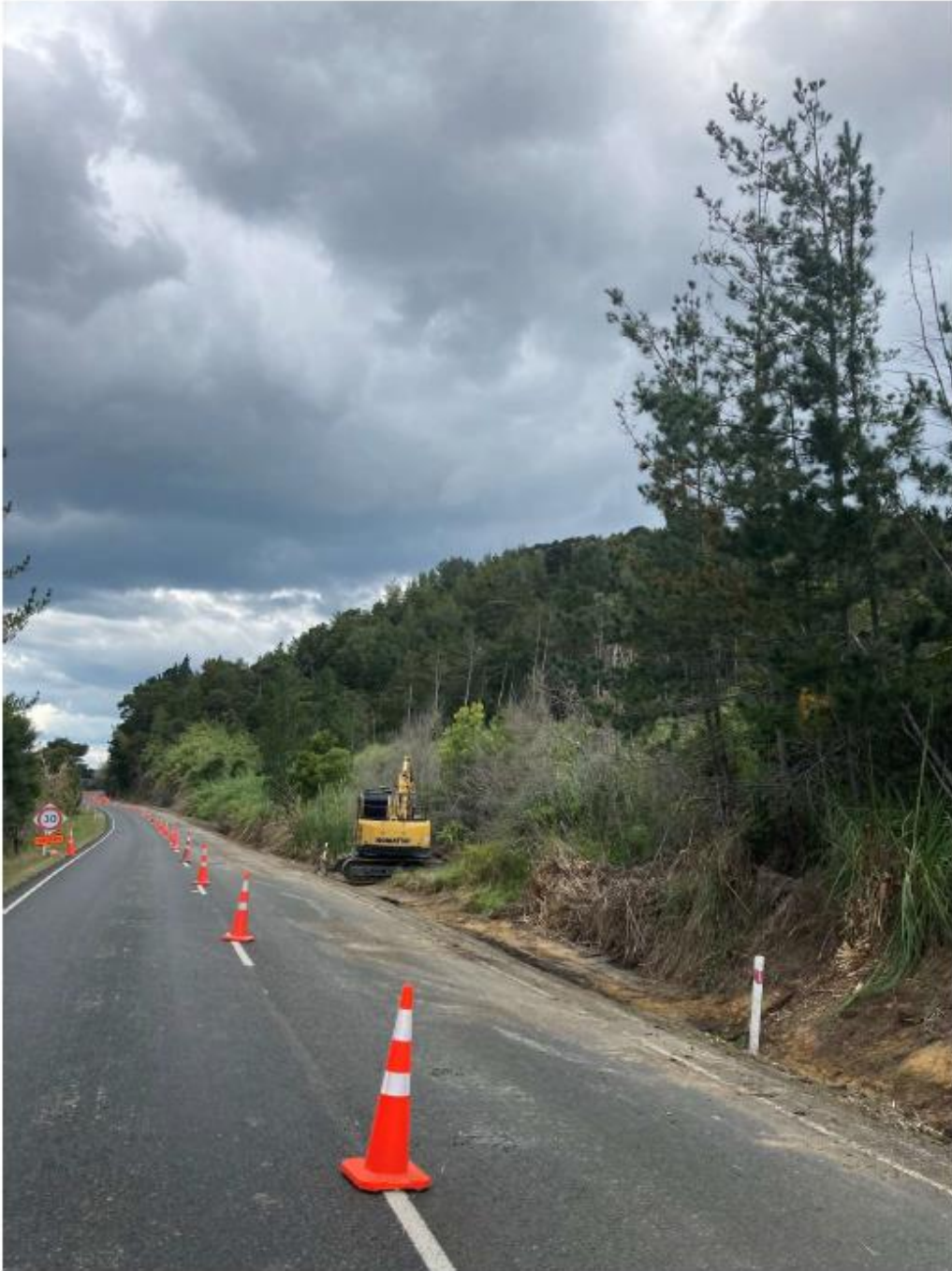
Figure 16: Kohukohu Rd Rehabilitation Site Clearing
