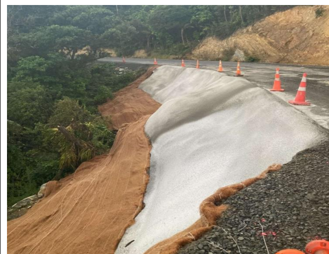
Peria Road / Seal Extension RP4100 Slip Repair
