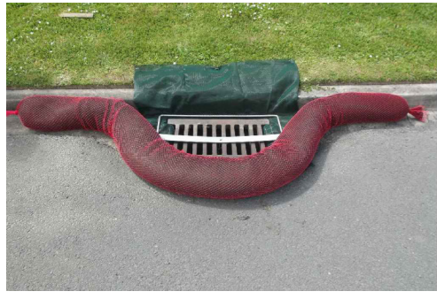
CATCH PIT E&S PROTECTION VIA SILT FENCE
