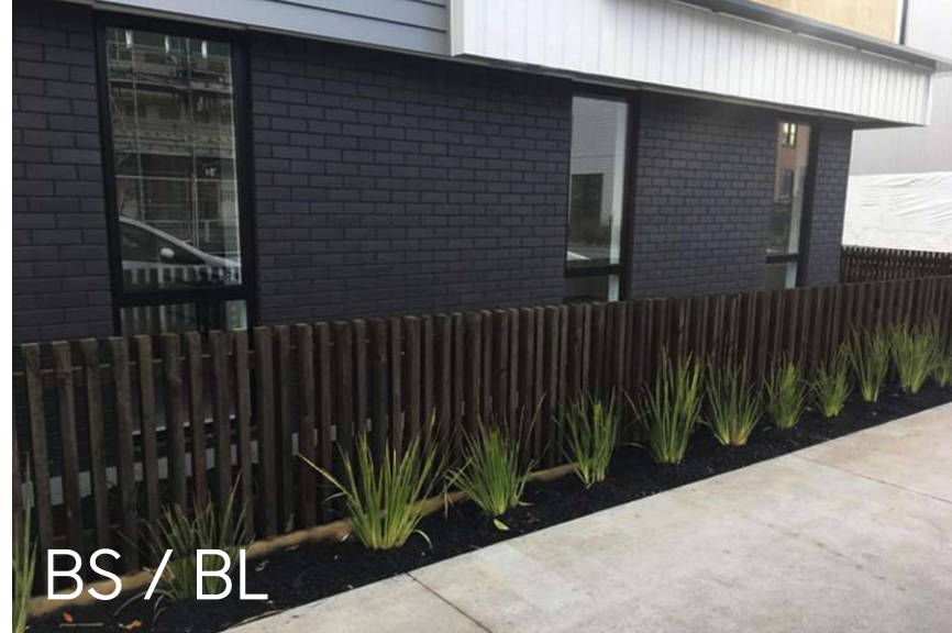
BS / BL 1.2m / 0.9m Timber batten fence
