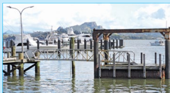
Three wharves in Whangaroa Harbour are set for upgrades.
